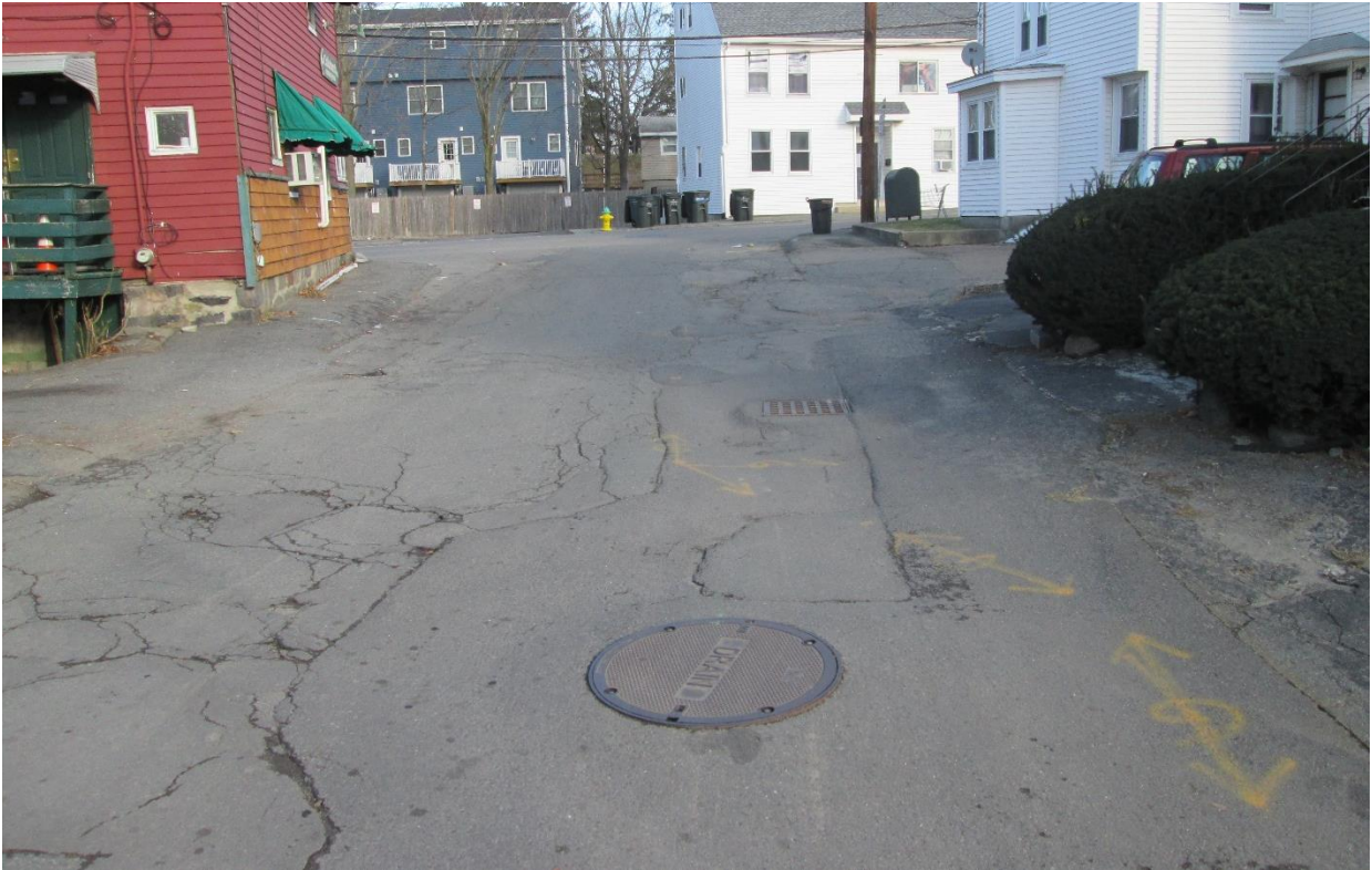
Photo #2: Furnace Avenue looking north.
