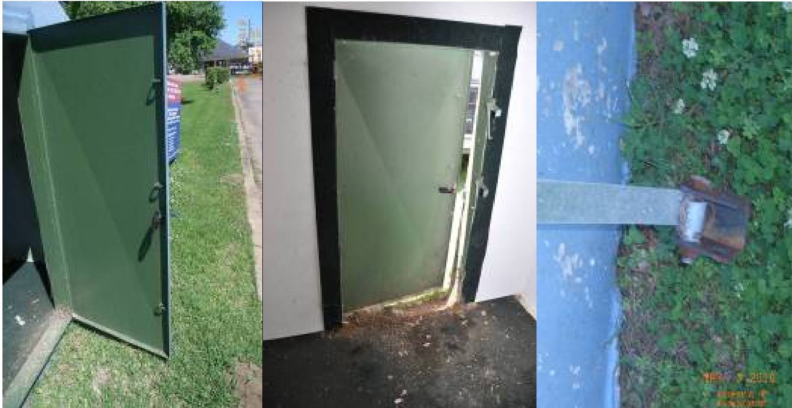
Figure 22: Durant Police Station, Holmes County, FEMA 361 Community Safe Room
