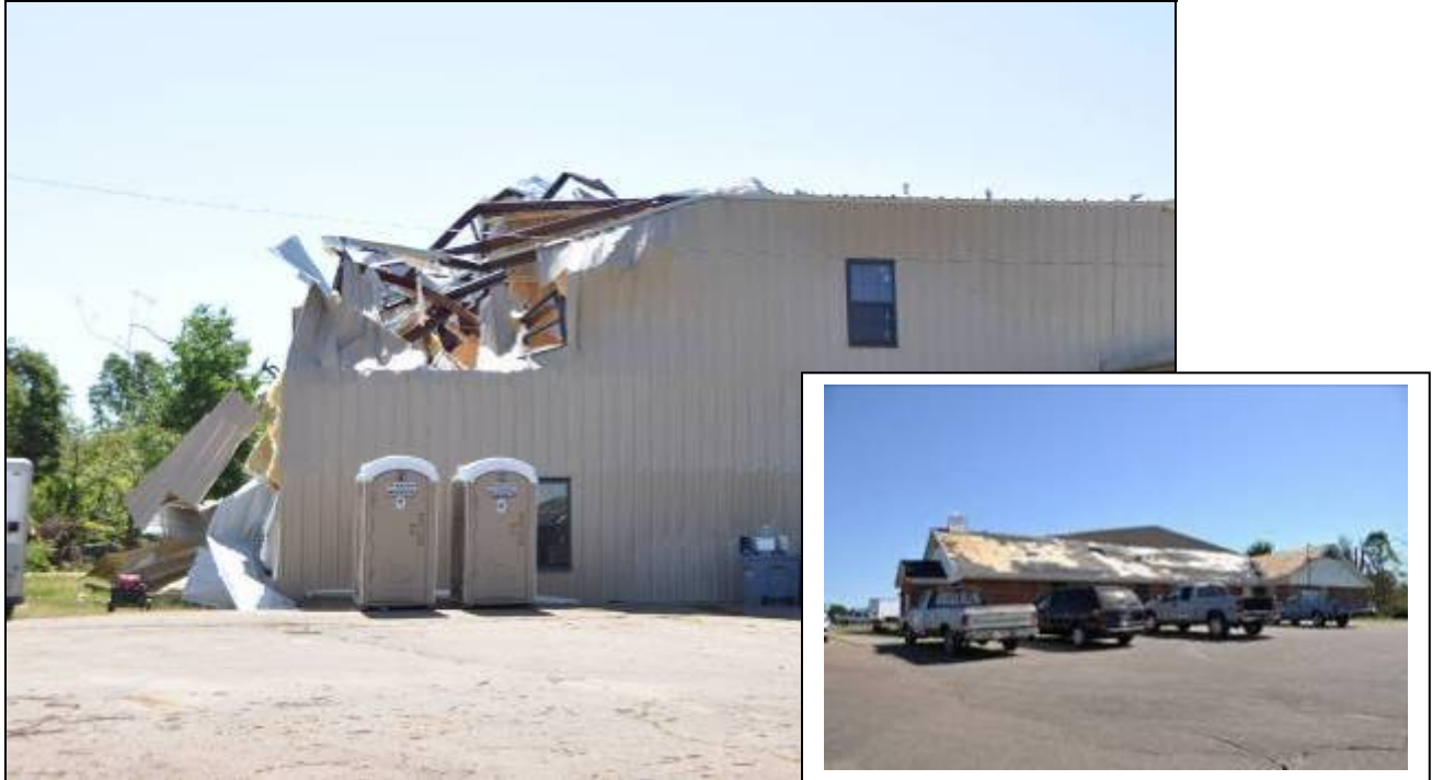
Figure 9: Sanctuary and Fellowship Hall (Left), Mills Spring Missionary Baptist Church (Bottom Right), Choctaw County, MS, EF-2, 120 mph
