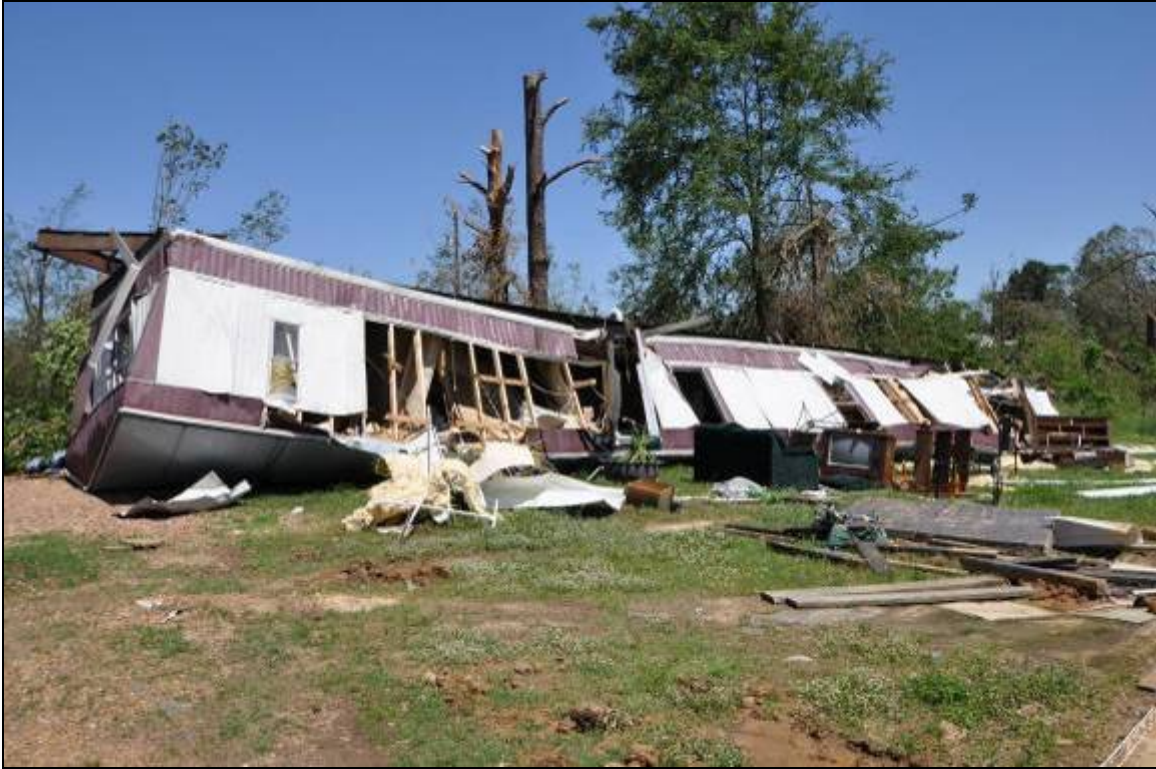
Figure 7: Rolled Manufactured Home, Ebenezer, Holmes County, MS, EF-2, 110 mph
