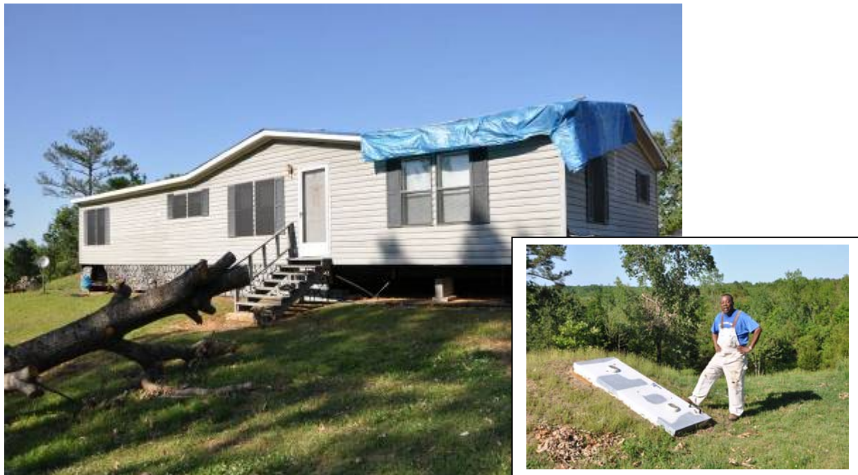
Figure 19: Safe Room #9, Oktibbeha County, MS
