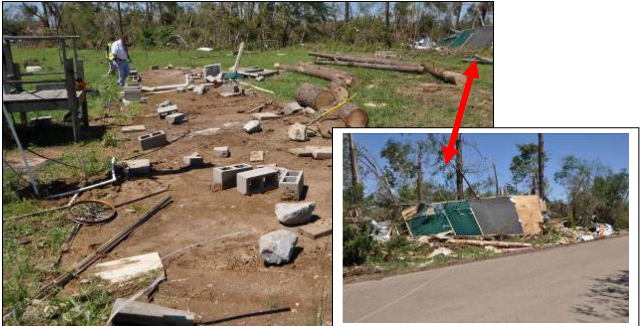
Figure 8: Vaulted Manufactured Home, Ebenezer, Holmes County, MS, EF-2, 110 mph
