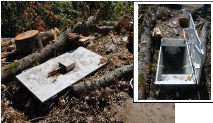
Figure 11: Safe Room #1, Yazoo County, MS
