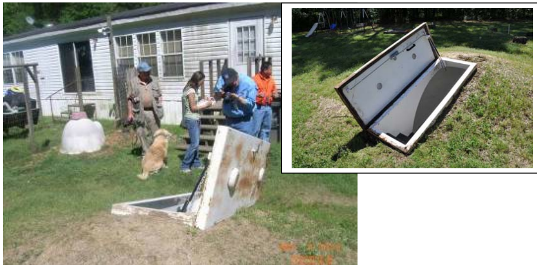
Figure 18: Safe Room #8, Starkville, Oktibbeha County, MS
