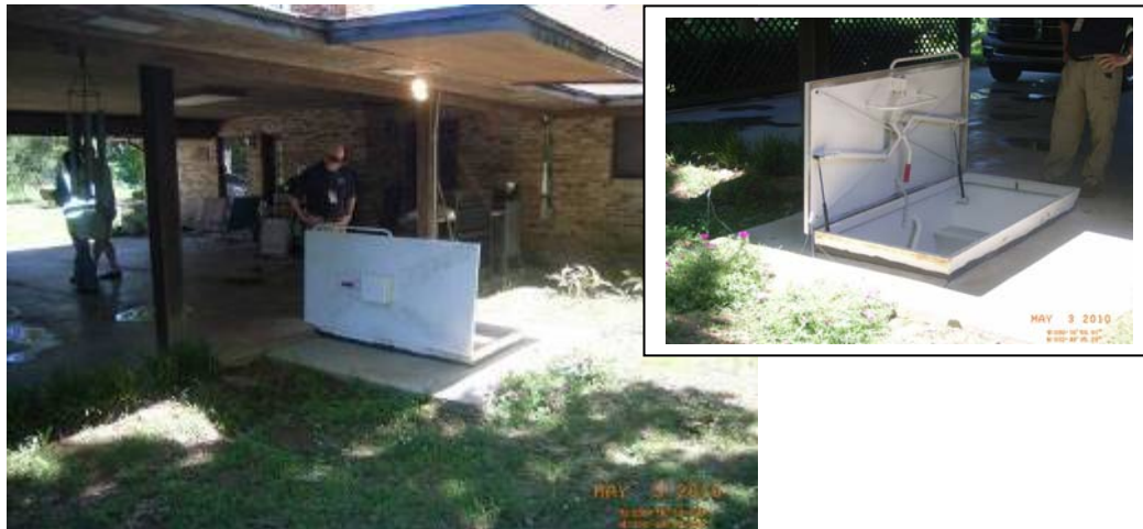
Figure 13: Safe Room #3, Yazoo County, MS
