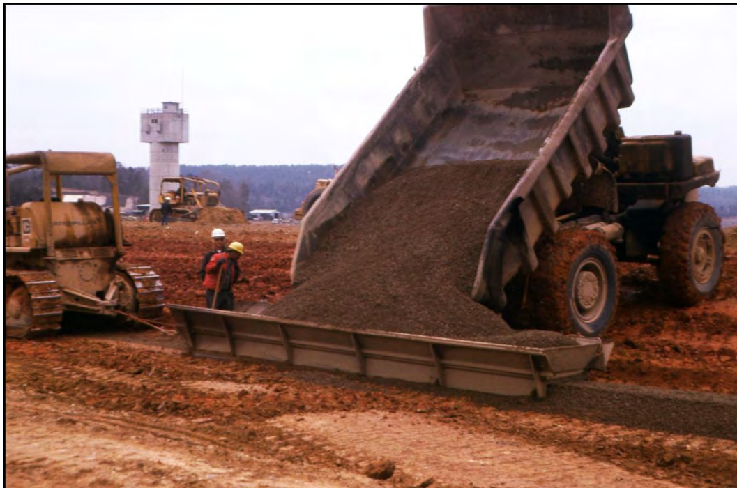
Figure 7-16. Dumping into spreader box.
