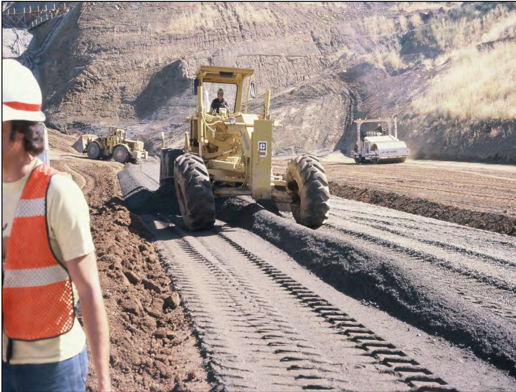
Figure 7-13. Spreading sand filter material.
