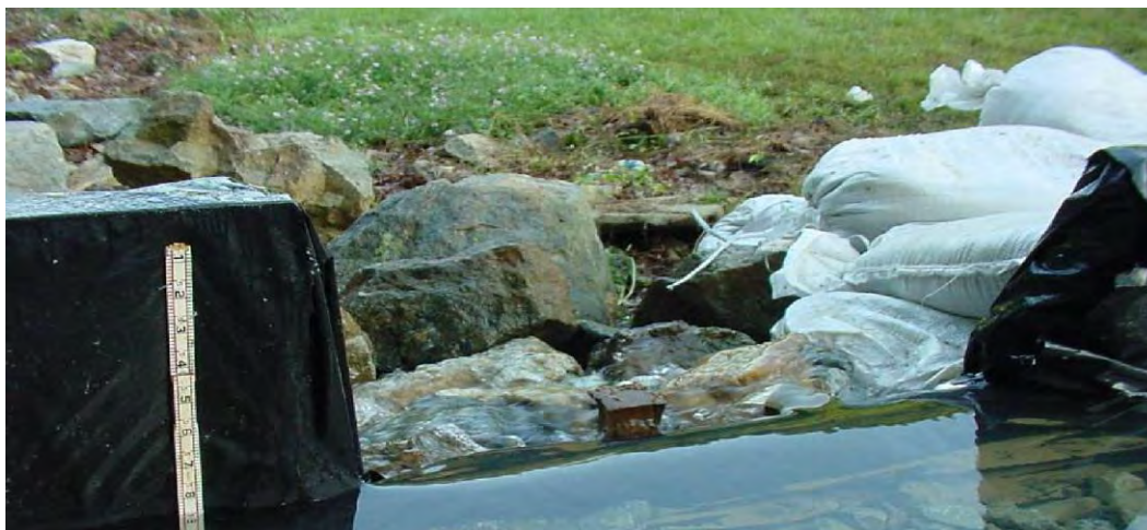
Figure L-26-3.—Although a gravel filter was placed over the flow area, it was so coarse that it would not have been an effective filter for eroding fine particles, had there been any. Fortunately, in this situation, the flow in the bedrock was not in contact with the embankment, and no erosion of the fill occurred.
