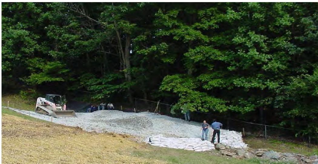
Figure L-26-2. Gravel drain being placed over seepage area.
