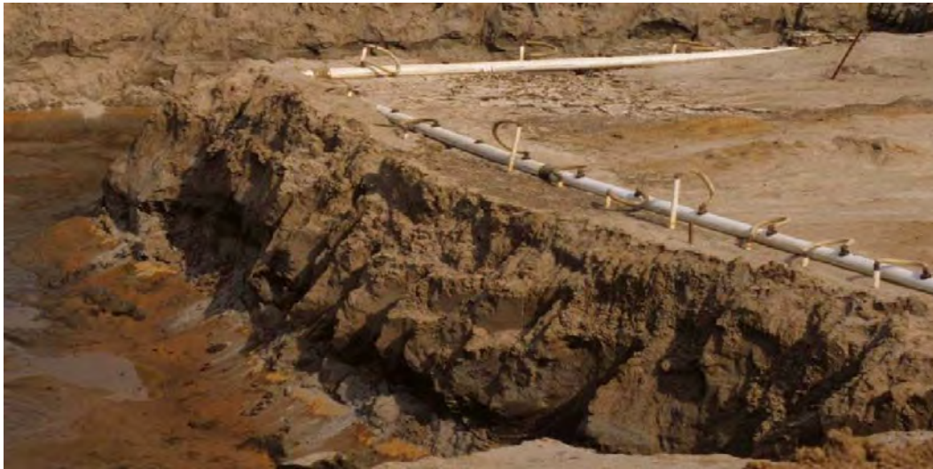
Figure L-32-1.—Well points used to dewater excavation below the water table.
