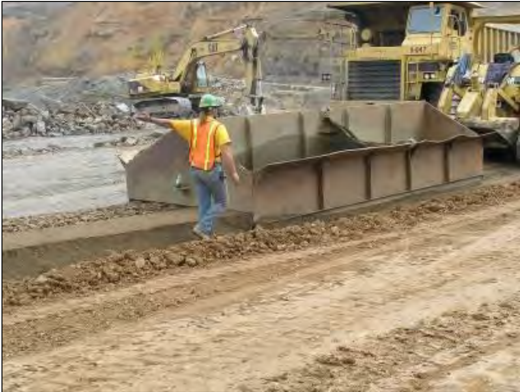
Figure 7-17. Towing spreader box.
