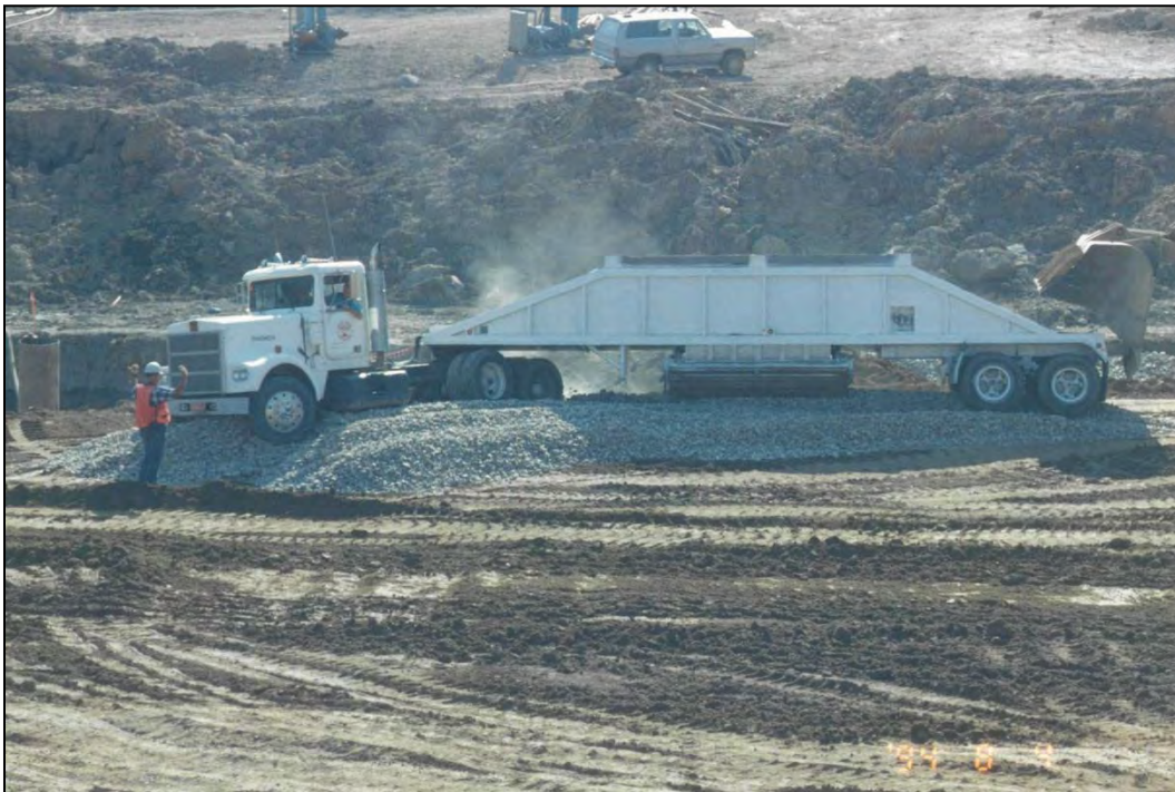
Figure 7-12. Articulated bottom-dump truck. The photo illustrates difficulty that can arise when the truck dumps too quickly for the speed of the truck. The trailer will then hang up and require assistance from other equipment.
