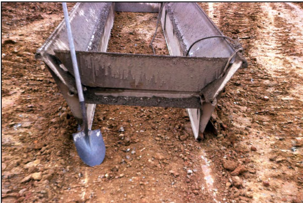
Figure 7-14. Basic single-bin spreader box.
