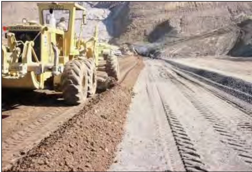
Figure 7-3. Windrowing impervious material adjacent to a filter/drain.
