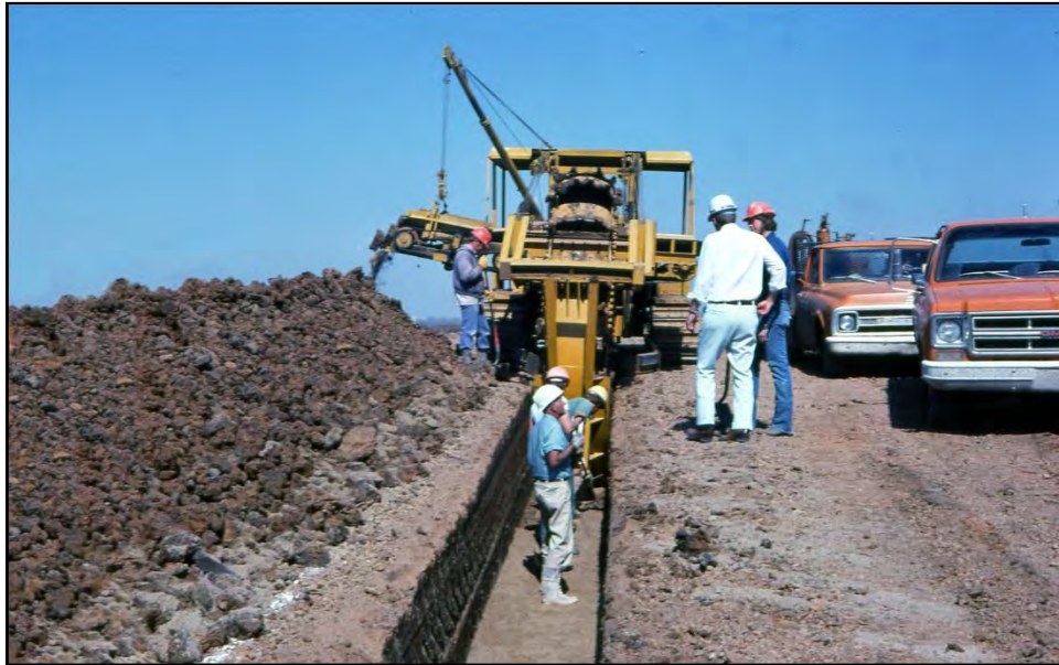
Figure 7-5. Trenching method – excavating trench.
