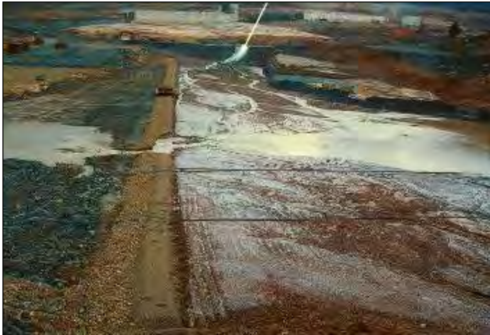
Figure 7-25. Surface water contamination of a chimney filter.
