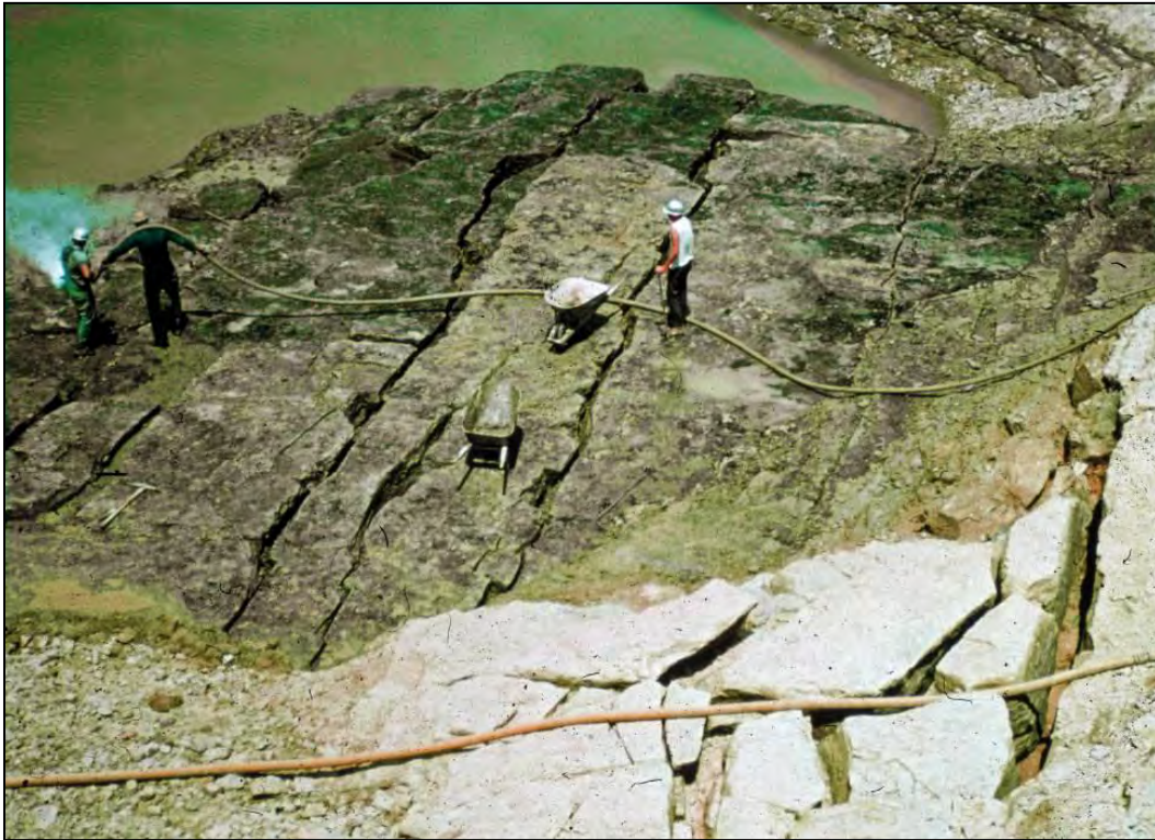
Figure 2-8. Pressure washing joints and fractures in bedrock prior to dental grouting and covering with blanket drain under downstream shell of dam. (Photo courtesy of NRCS.)
