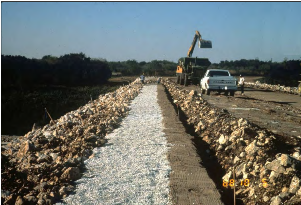
Figure 2-4. Multiple zone chimney filter being constructed in zoned dam by concurrent method of construction.
