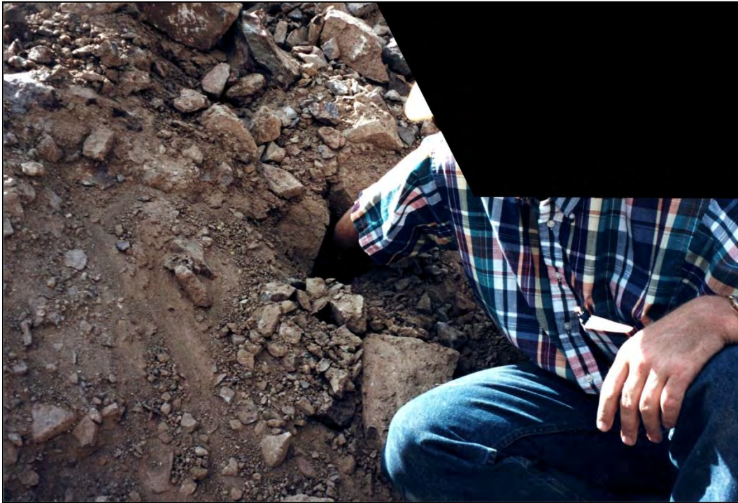
Figure 6-6. Open work present in the right abutment foundation of Ochoco Dam. The abutment consists of landslide debris.
