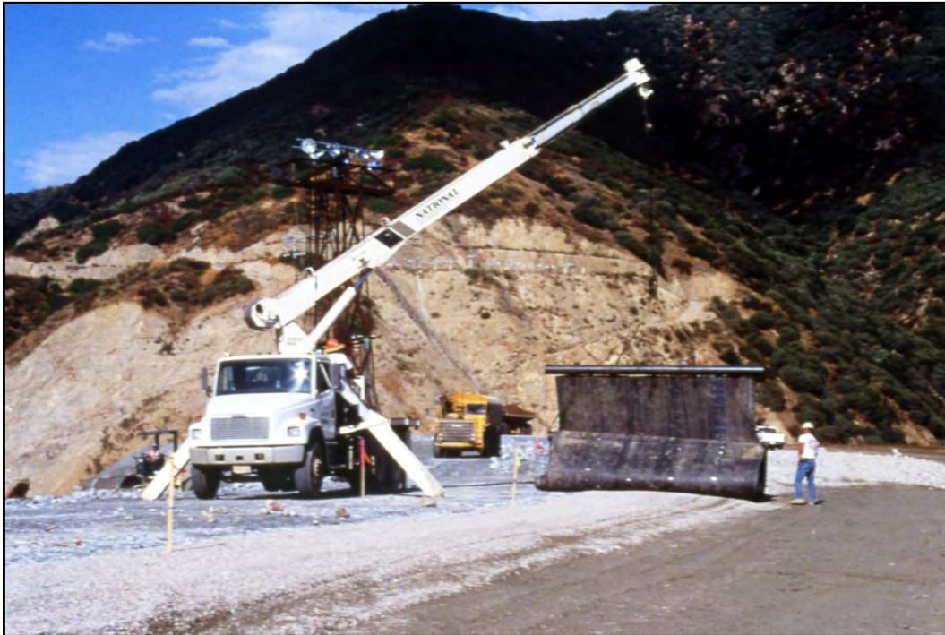
Figure 7-28. Placement of geomembrane at crossing over a chimney filter and drain.
