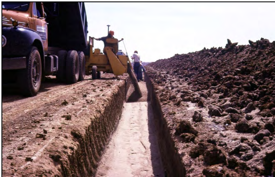
Figure 7-6. Trenching method – backfilling trench.
