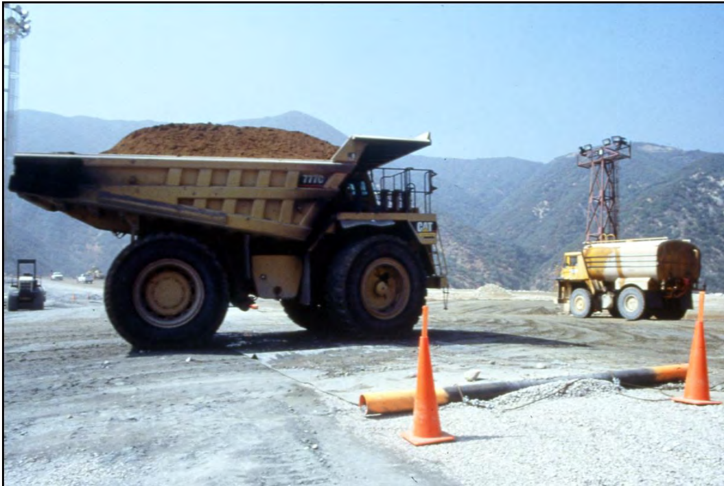
Figure 7-11. Large end-dump truck utilizing an equipment crossing over a chimney filter.
