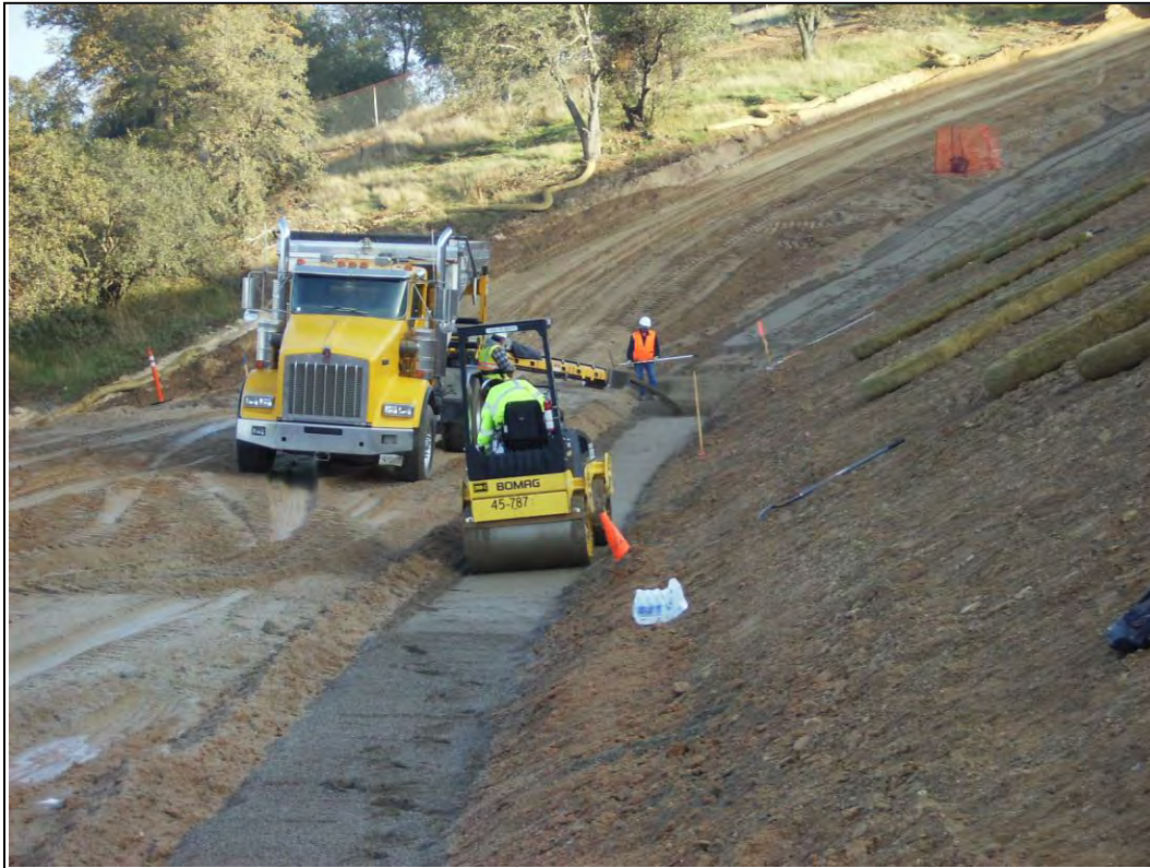
Figure 7-20. Truck conveyor delivering filter sand for the addition of a 4-ft-wide chimney filter to an existing embankment. Note that the material is uniformly placed from the conveyor, and no leveling is required. Dynamic compaction is provided by the roller shown in the foreground.
