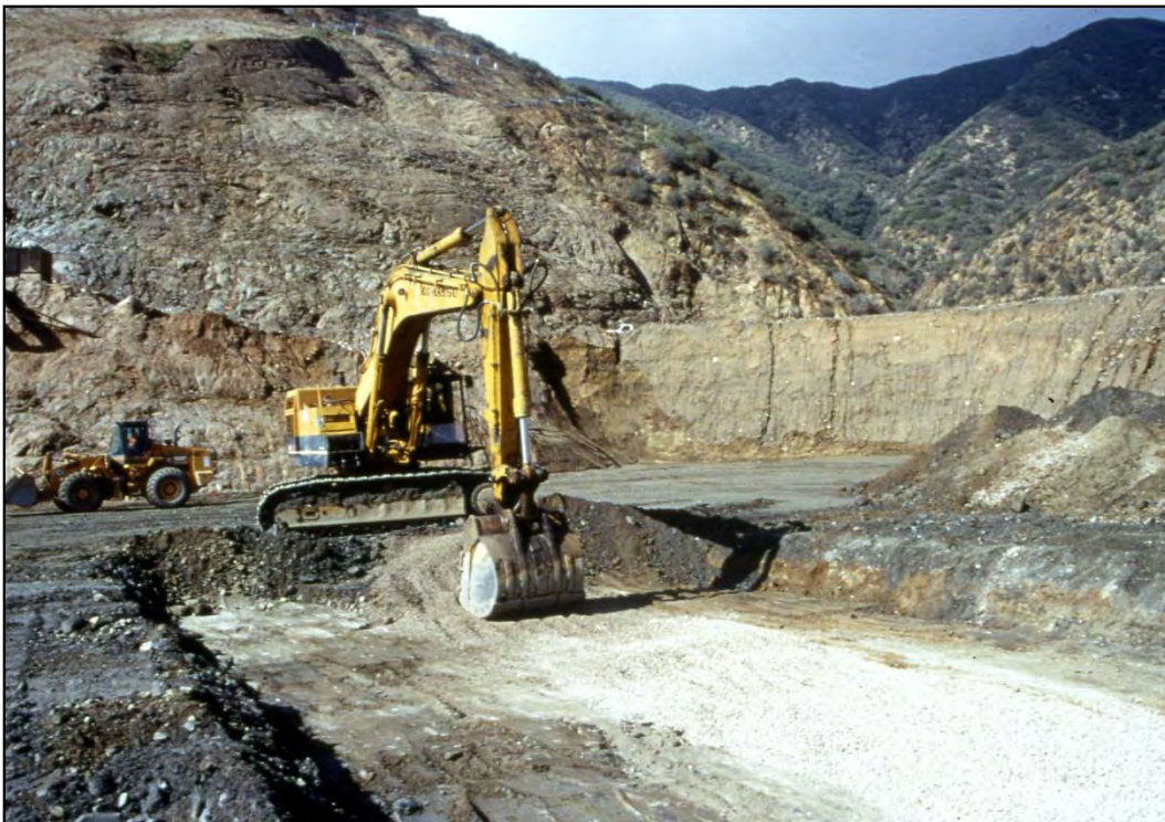
Figure 7-27. Excavation of filter material under equipment crossing.
