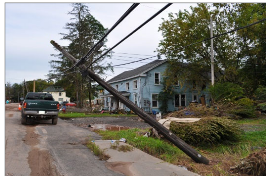
Power lines in NY damaged by Hurricane Irene and Tropical Storm Lee.
