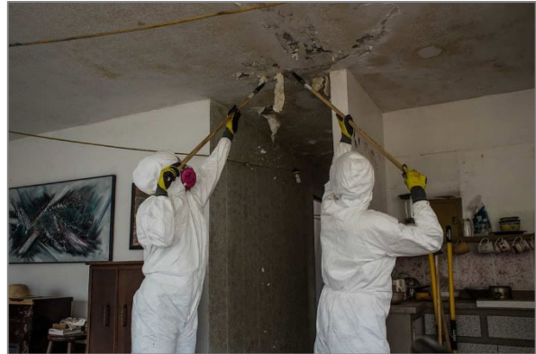
AmeriCorps members work to repair homes damaged by Hurricane Maria in Humacao, Puerto Rico.
