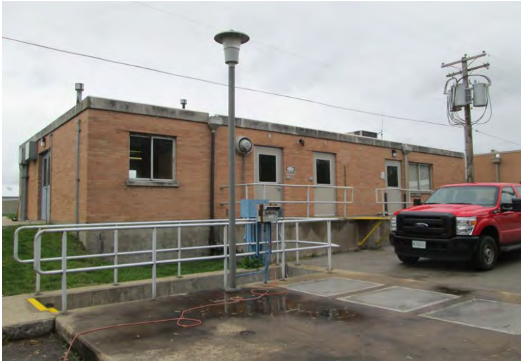
Photo 9: East elevation of c. 1974 Lab Building.
