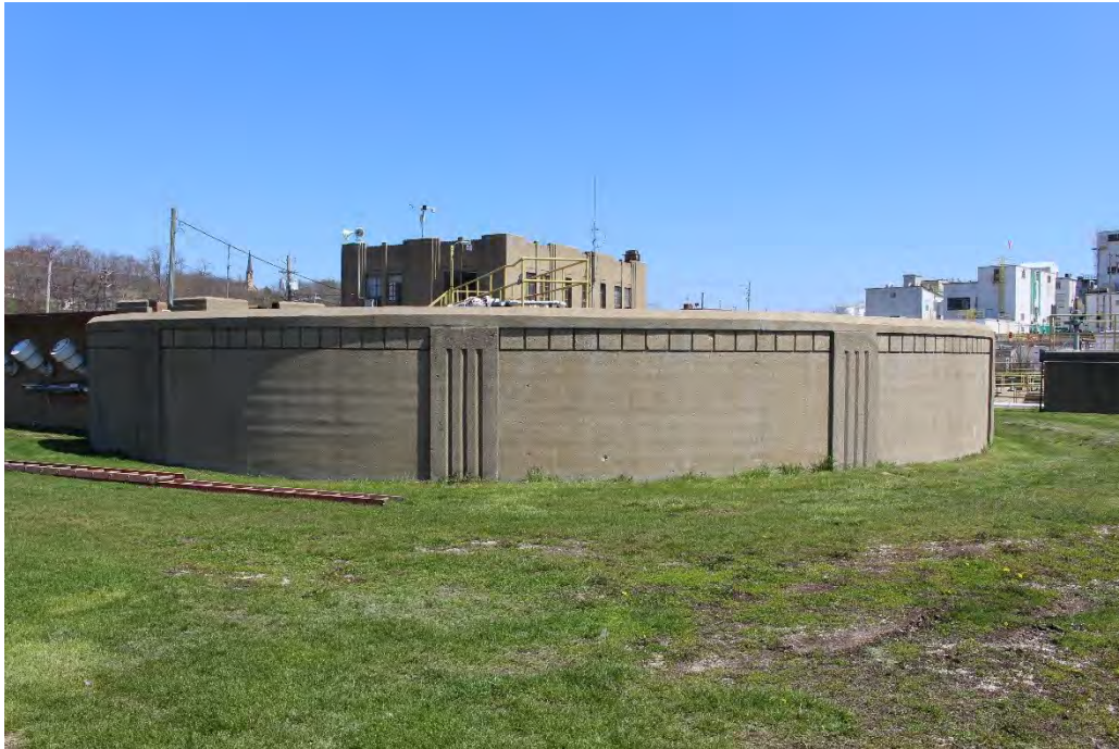
Photo 23: View northwest to c. 1939 Secondary Digester Tank.
