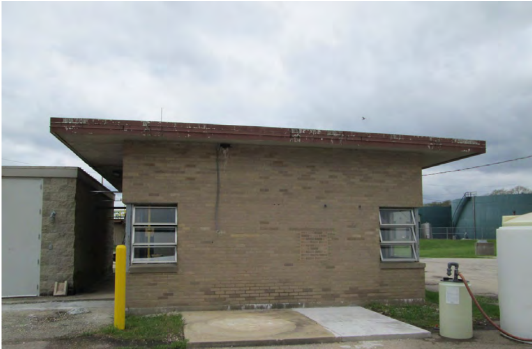
Photo 17: East elevation of Storm Building/Excess Flow.
