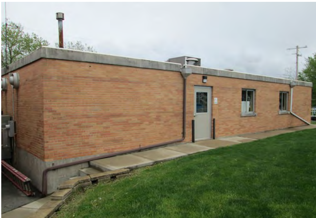
Photo 10: West elevation of Lab Building.
