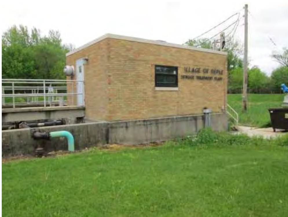
Photo 8: View southwest to north elevation of Lab and Pump Building.
