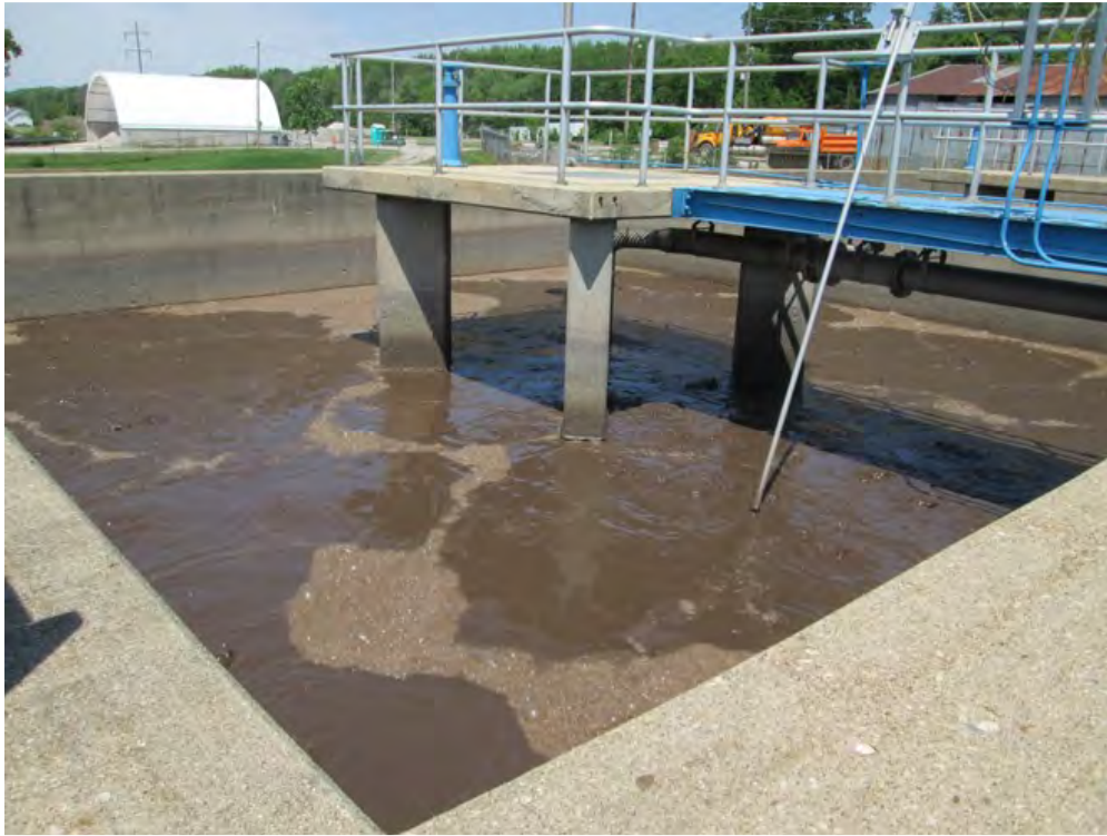
Photo 21: View northwest across c. 1974 Aerobic Digesters.
