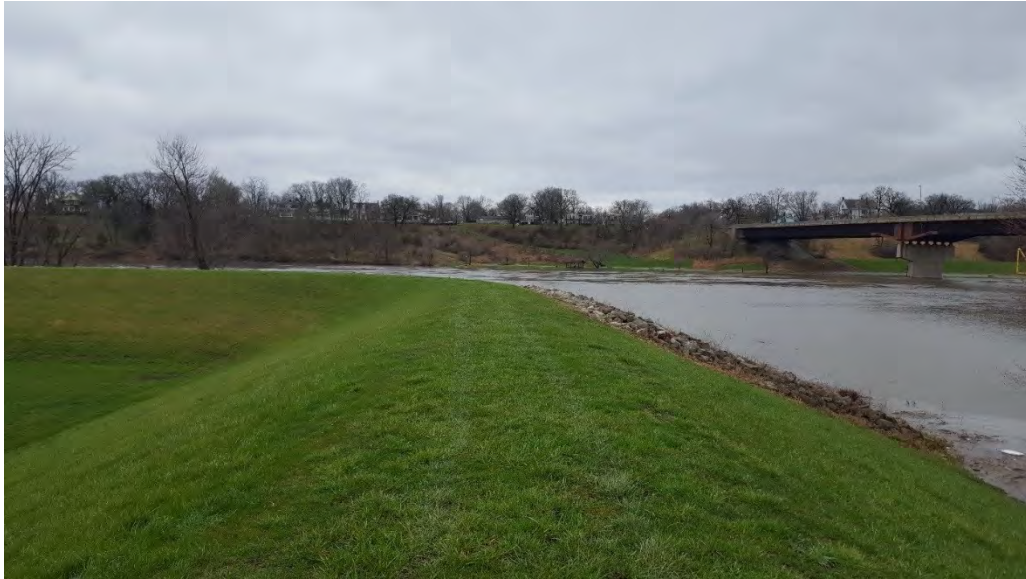
Photo 1: View South along existing levee toward the confluence of the Illinois and Fox Rivers.
