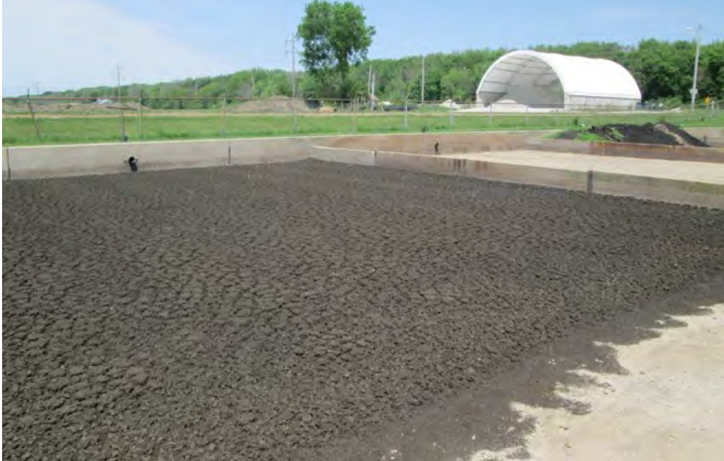
Photo 25: View northwest across Sludge Drying Beds.
