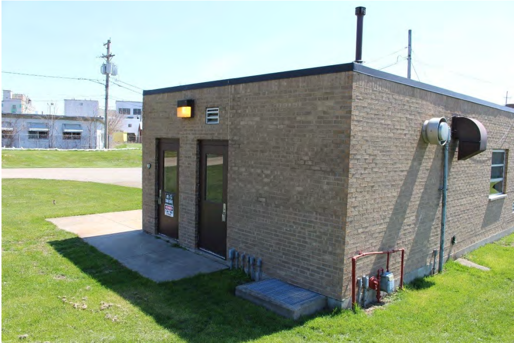
Photo 4: View southeast to north and west elevations of Grit Building.
