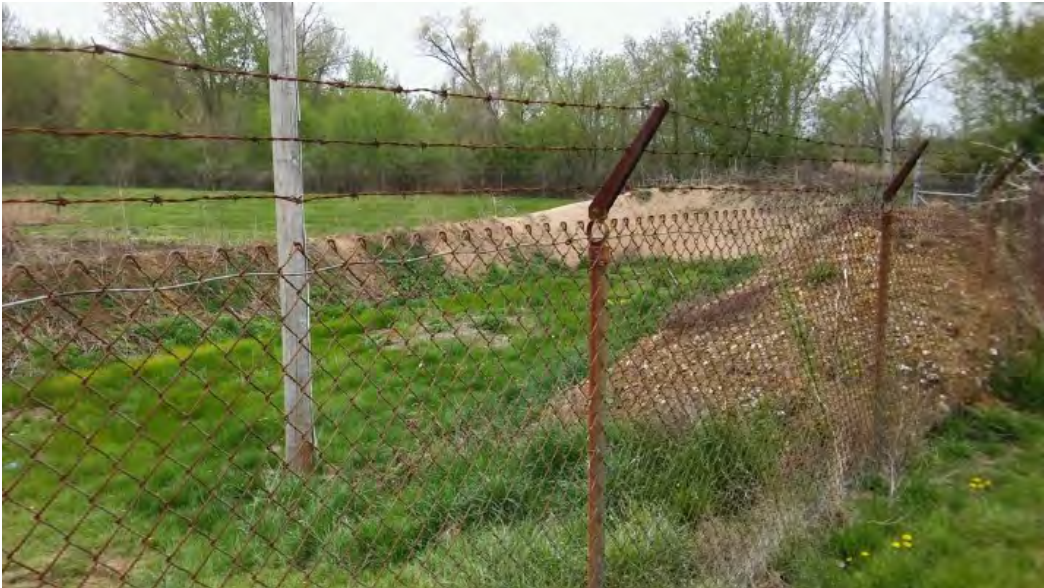
Photo 17: Facing southwest toward northwest corner of levee along north facility boundary.
