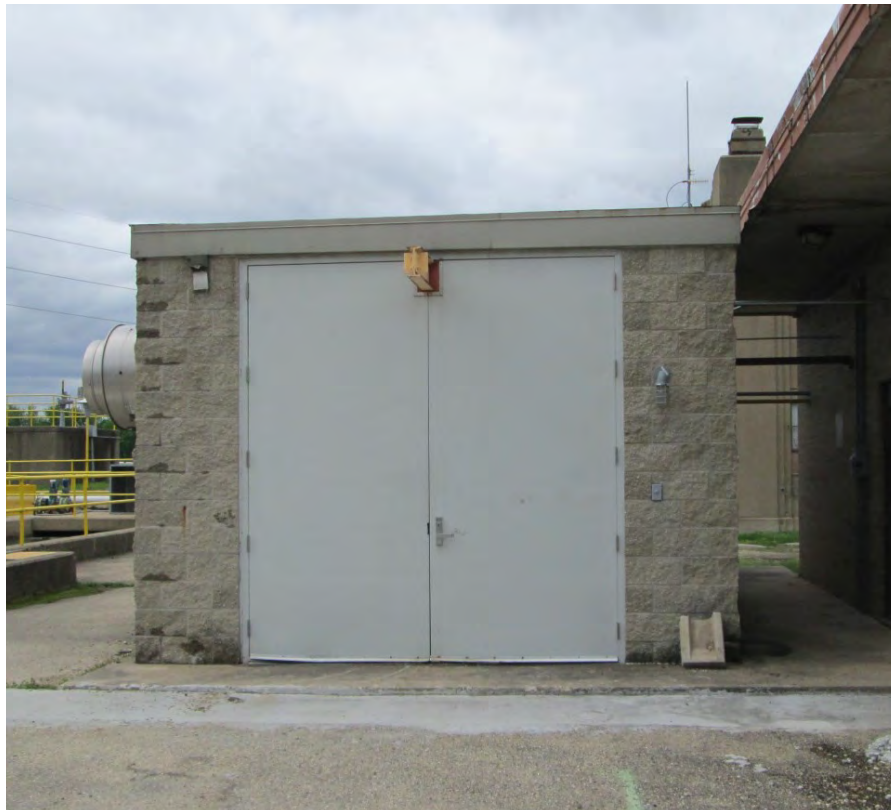
Photo 18: East elevation of Chlorine Building
