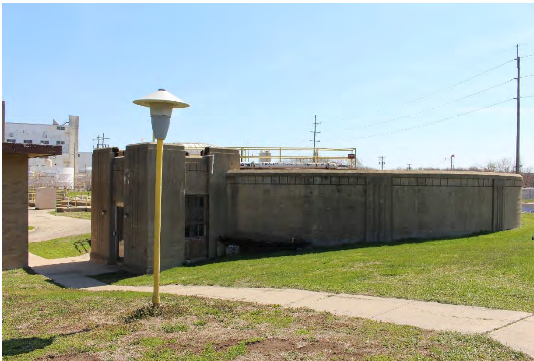
Photo 24: View southeast to Secondary Digester Tank and attached building.
