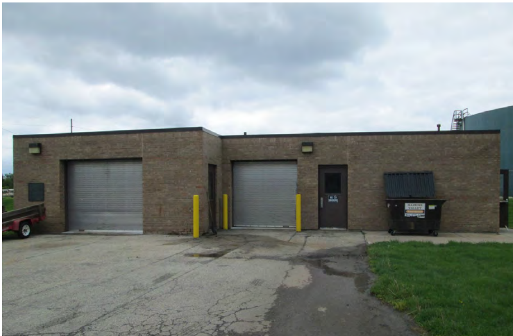
Photo 2: East elevation of Grit Building.
