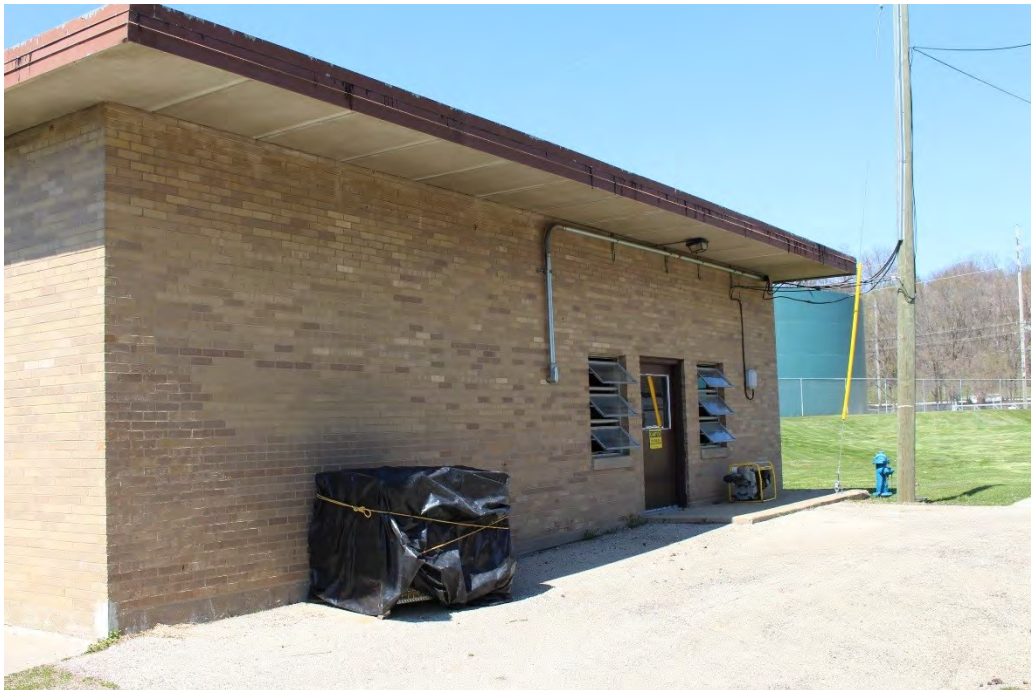
Photo 5: View northwest to east elevation of Blower Room Building.
