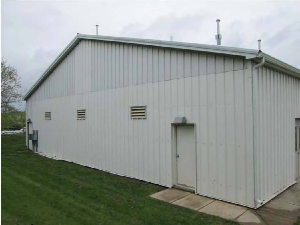
Photo 16: South elevation of Press Room/Sludge Room/Storage Building #2.
