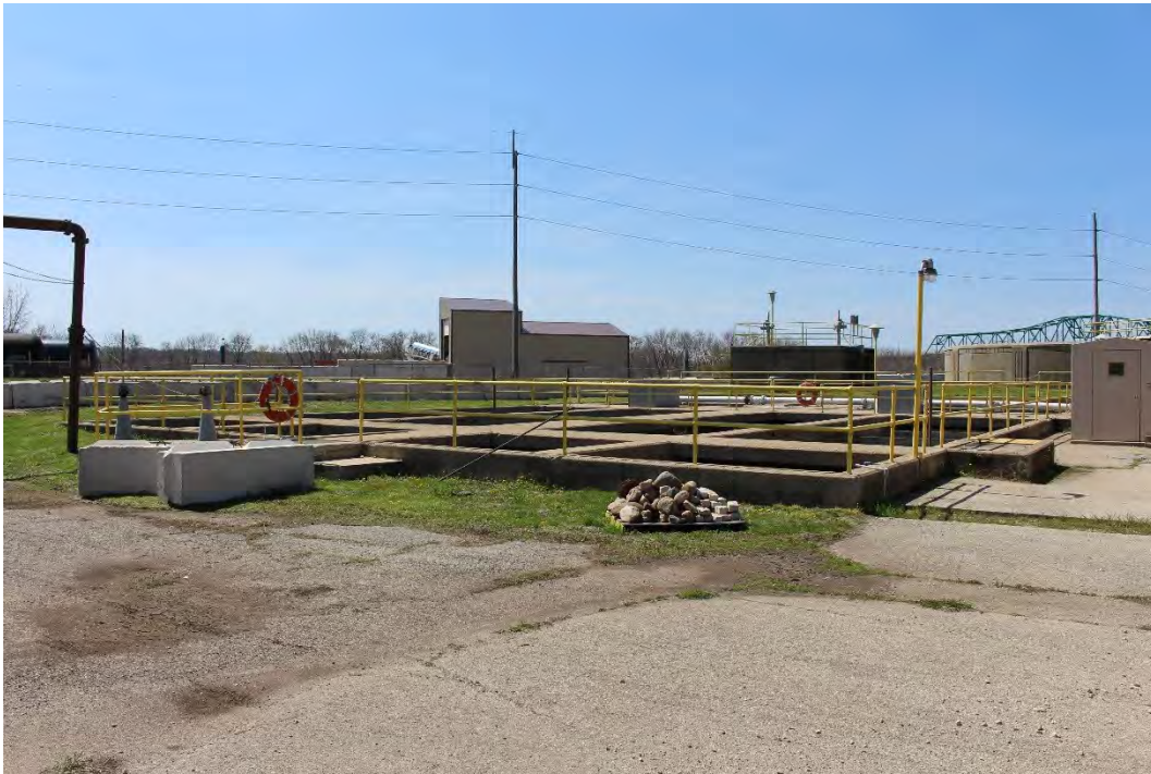
Photo 21: View southwest to Storage Tank.
