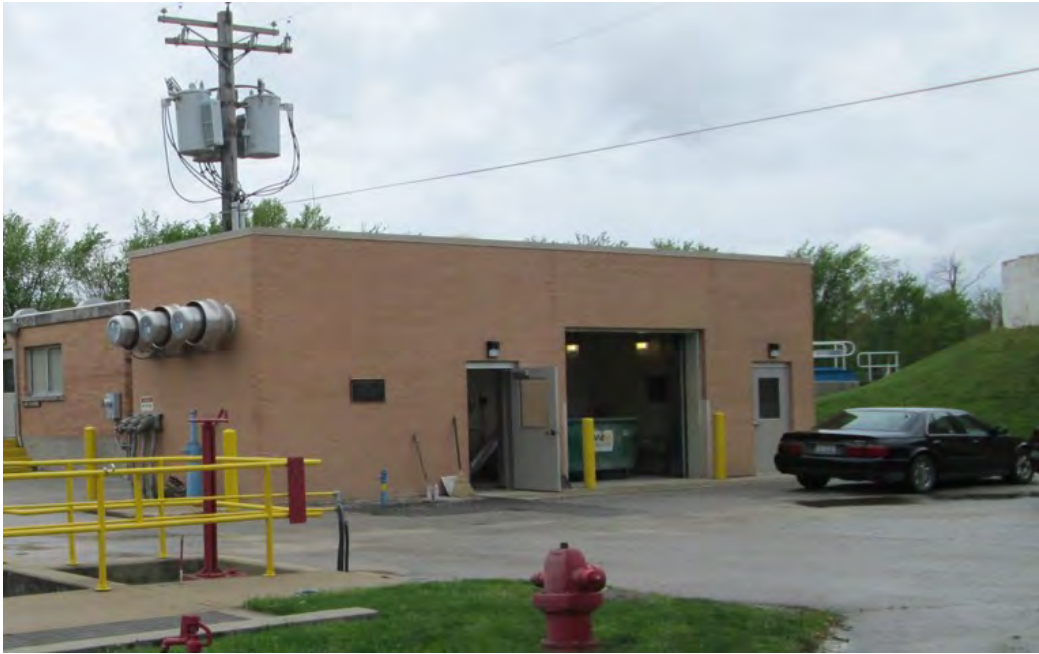
Photo 7: View south-southwest to north elevation of c. 1939 Raw Sewage/Bar Screen Building.
