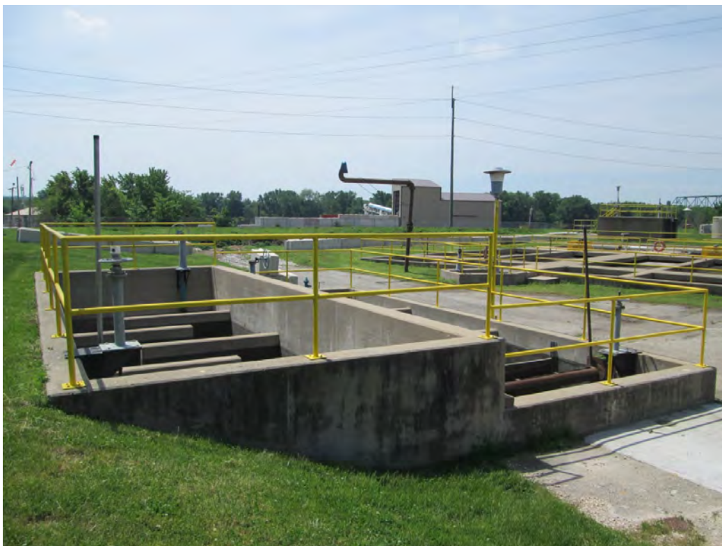
Photo 20: View southwest to Effluent Tank.
