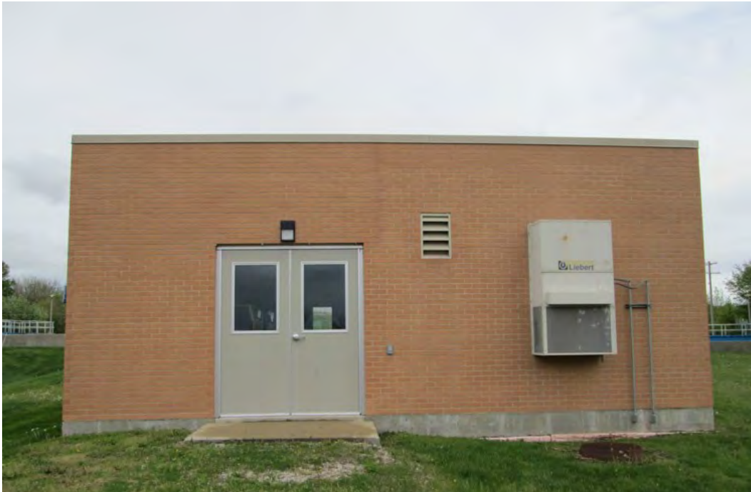
Photo 13: West elevation of c. 2010 Blower Room Building.
