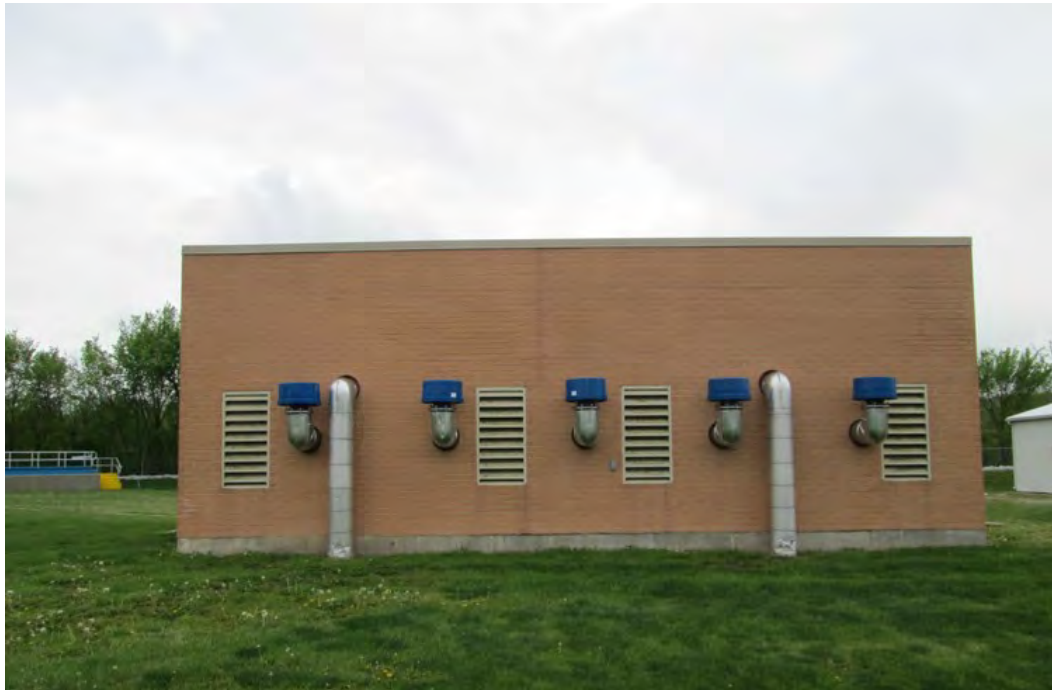
Photo 14: North elevation of Blower Room Building.
