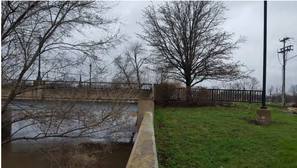
Photo 5: View North toward the Main Street Bridge along the existing concrete floodwall adjacent to the Fox River.
