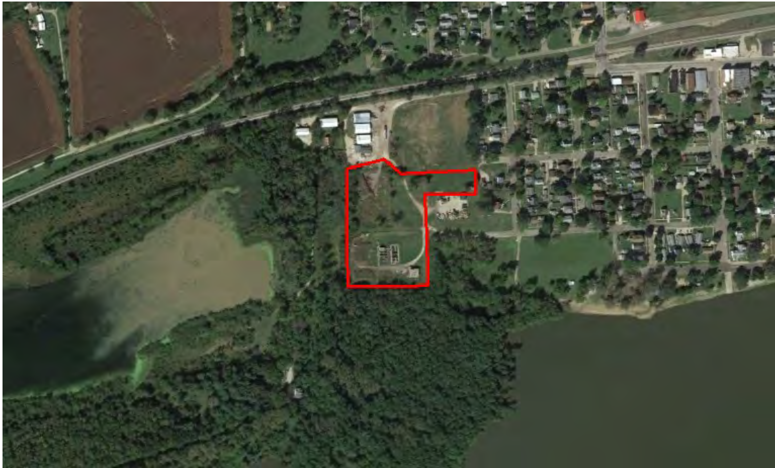
General Location for Proposed Floodwall Improvement ( Google Earth 2016 ).
