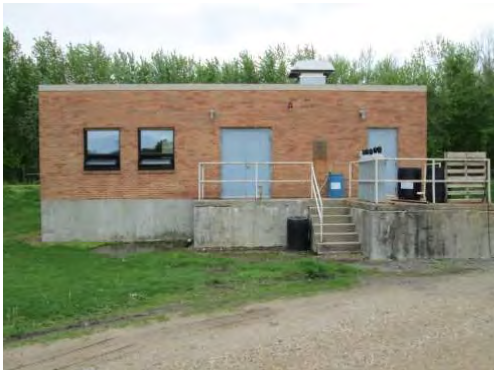
Photo 2: North elevation of Blower Building.
