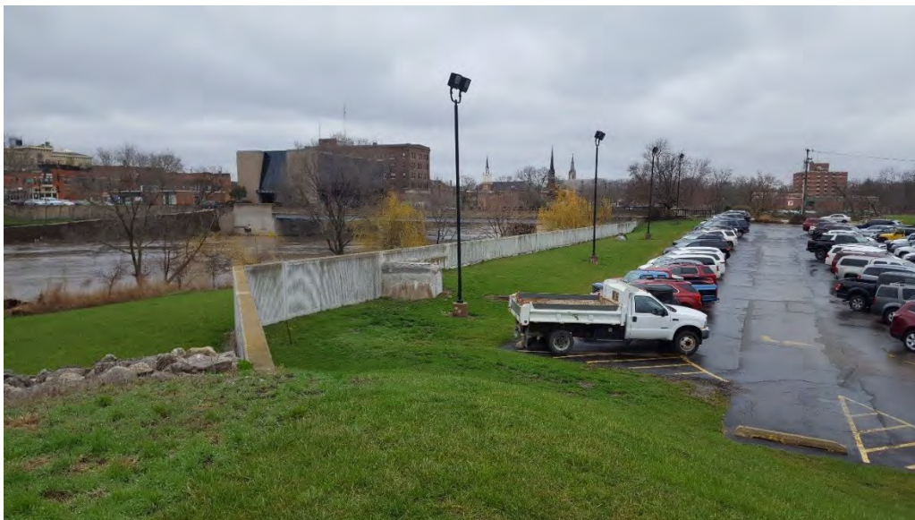
Photo 4: View Northwest of the existing concrete floodwall, riprap, and levee adjacent to the OTHS parking lot south of Main Street and the Fox River.
