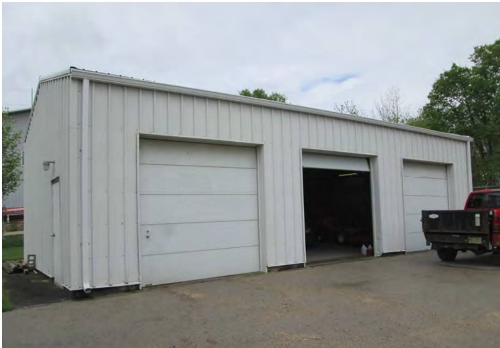
Photo 3: View north-northeast to south elevation of c. 2010 Storage Building.
