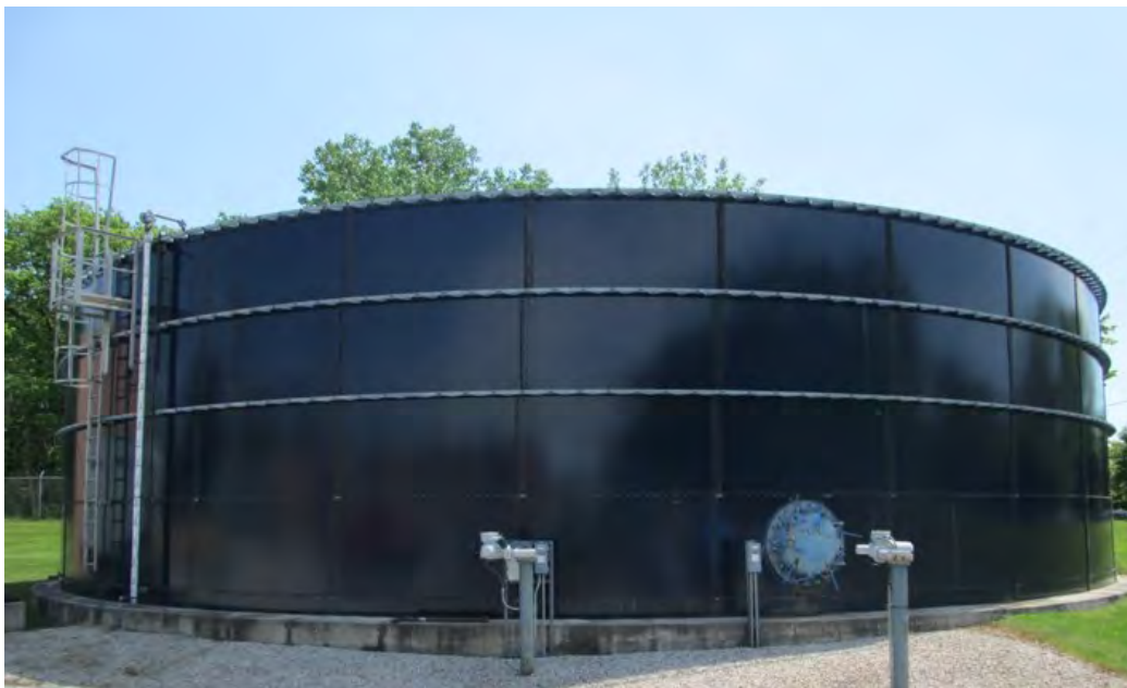
Photo 18: View east to c. 1974 Excess Flow Tank.
