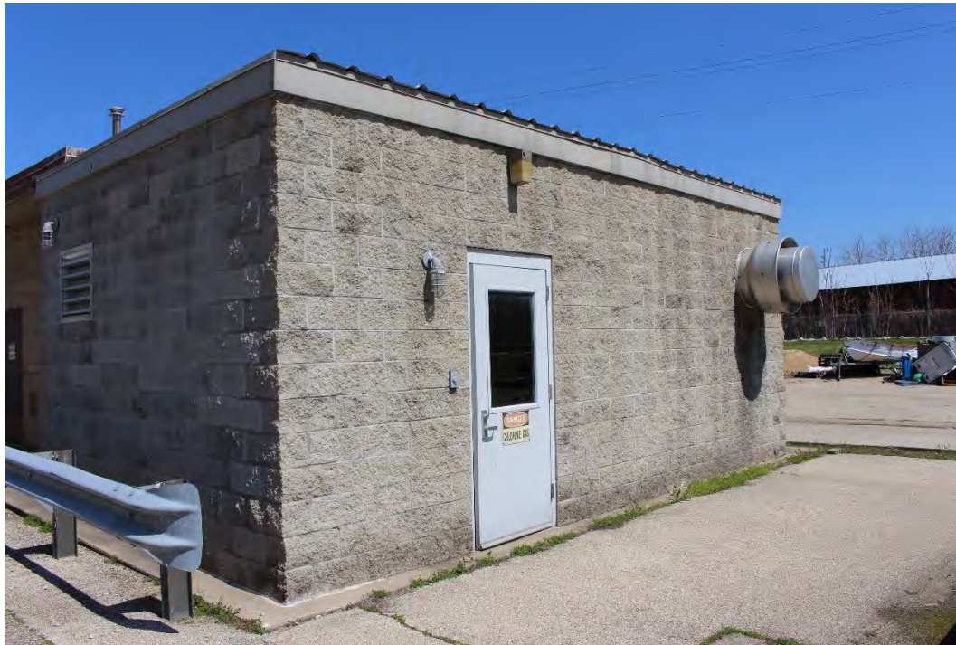
Photo 19: View northeast to west and south elevations of Chlorine Building.
