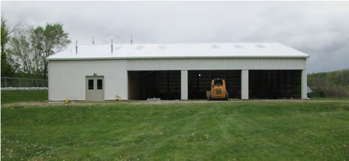
Photo 15: East elevation of c. 1974 Press Room/Sludge Room/Storage Building #2.
