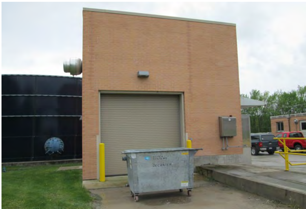
Photo 6: North elevation of Grit Building; Excess Flow Tank at rear left.
