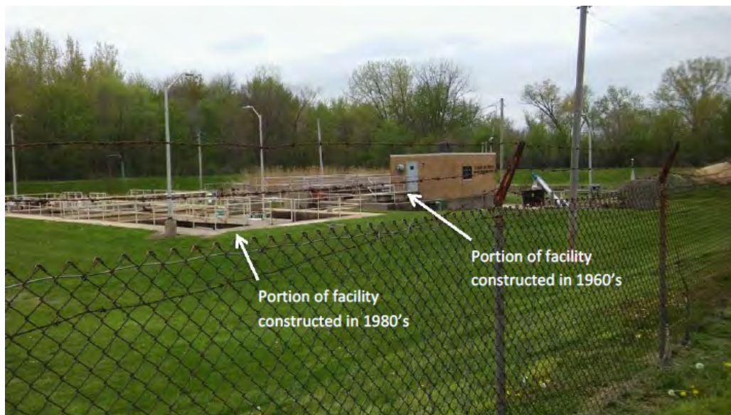
Photo 16: Facing southwest from levee along north facility boundary.
