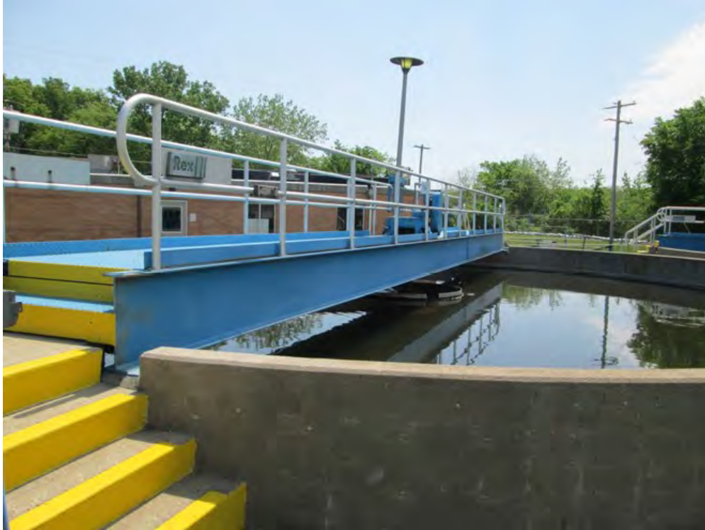
Photo 23: View northeast across c. 1974 Secondary Clarifiers.
