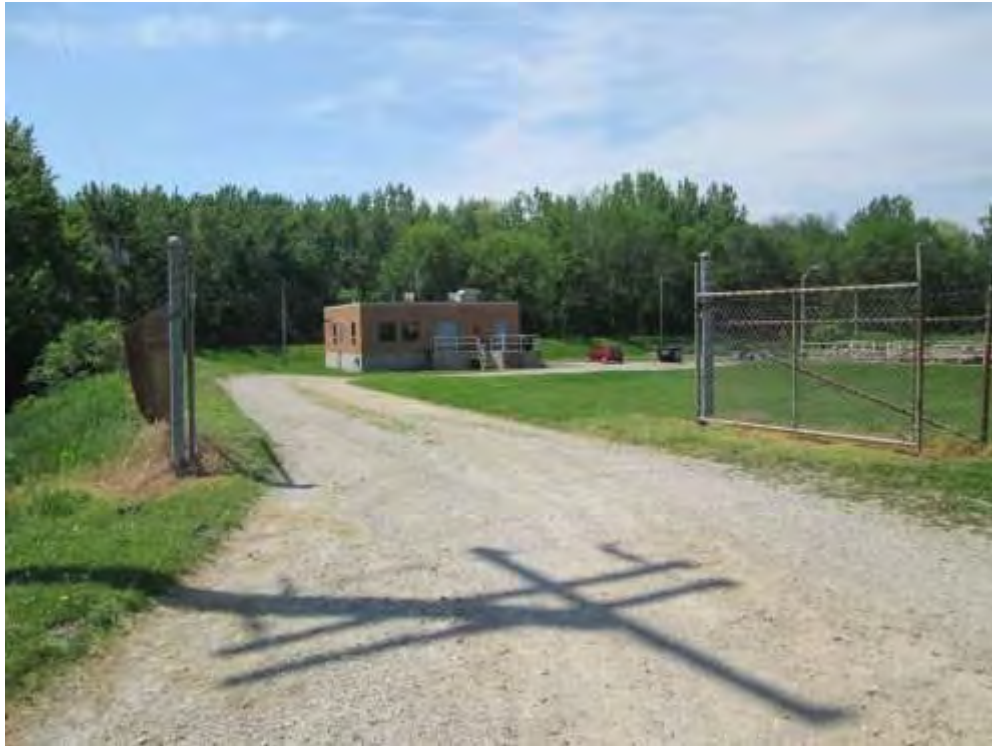
Photo 1: View south from DePue WWTP entrance, Blower Building at center.
