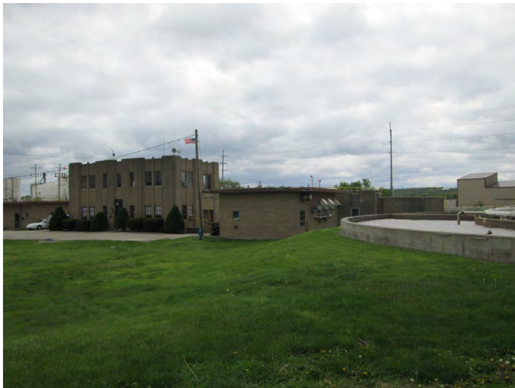
Photo 14: View south-southeast toward Control Building (left) and Blower Room Building (center).
