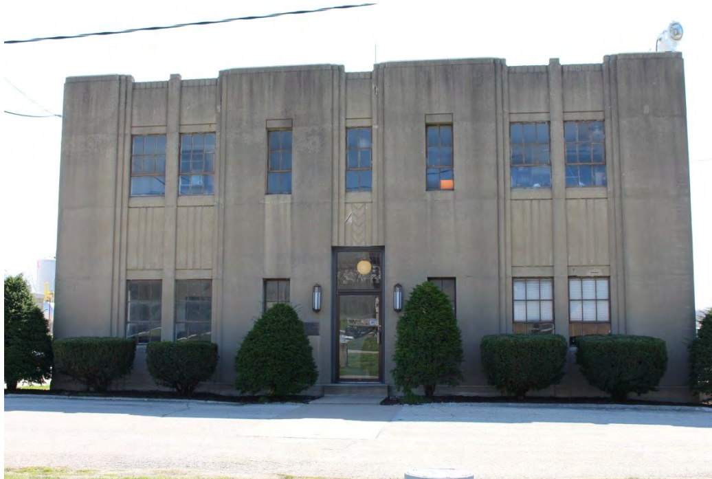
Photo 8: North elevation of c. 1939 Control Building.
