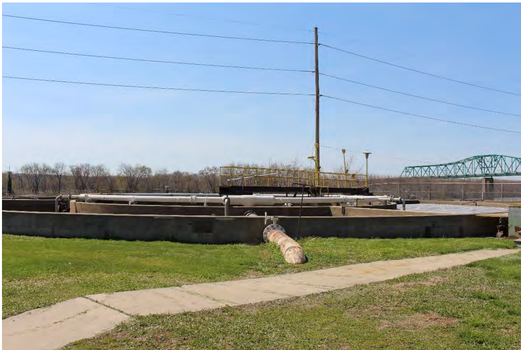
Photo 26: View south-southwest to Walker Processor Unit 2.
