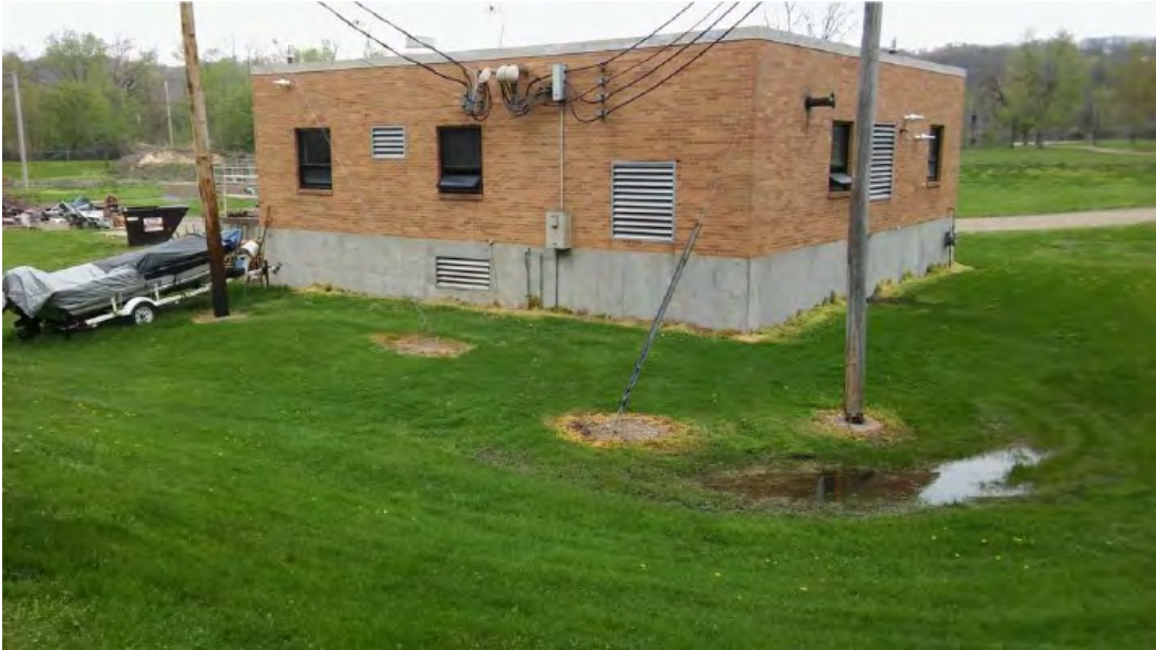
Photo 18: Facing northwest from southeast corner of levee.
