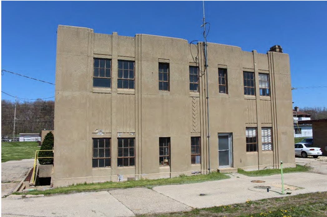
Photo 9: South elevation of Control Building.
