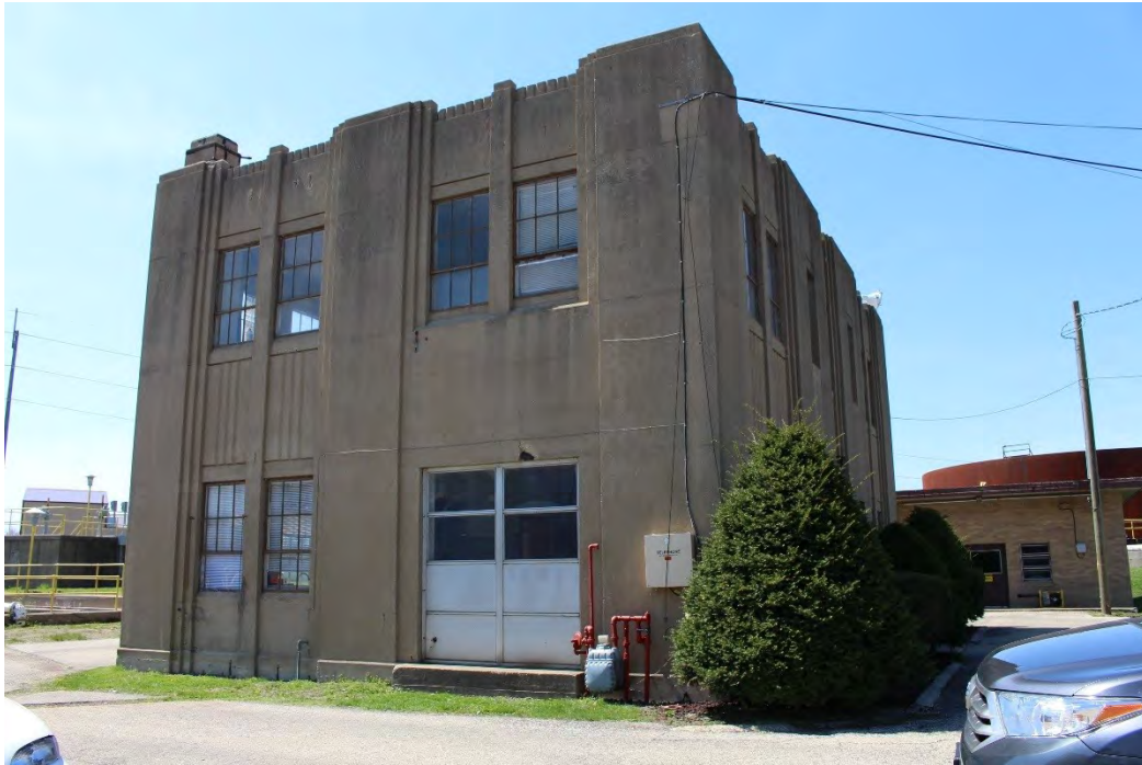
Photo 11: East elevation of Control Building
