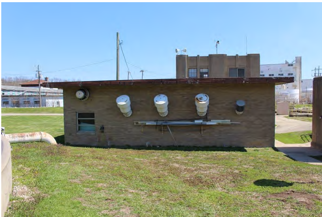
Photo 6: West elevation of Blower Room Building.
