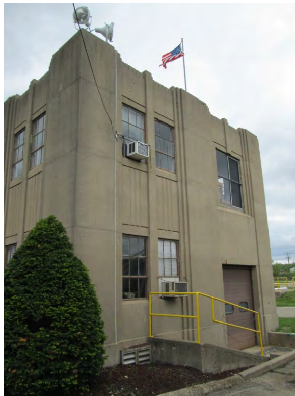
Photo 10: West elevation of Control Building
