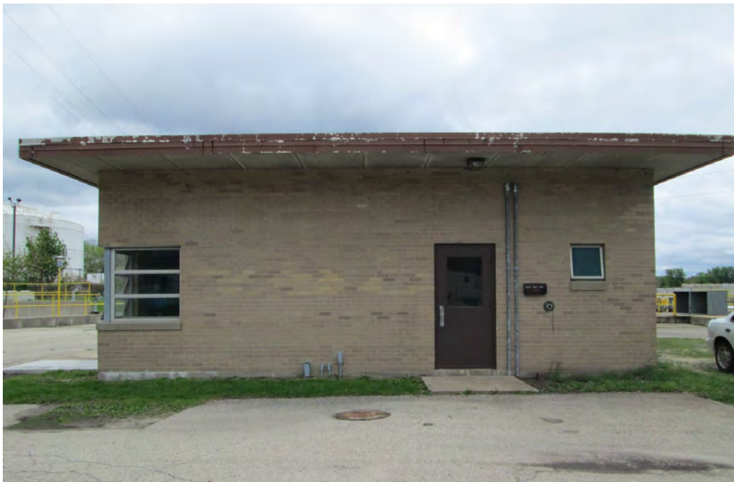
Photo 16: North elevation of Storm Building/Excess Flow.
