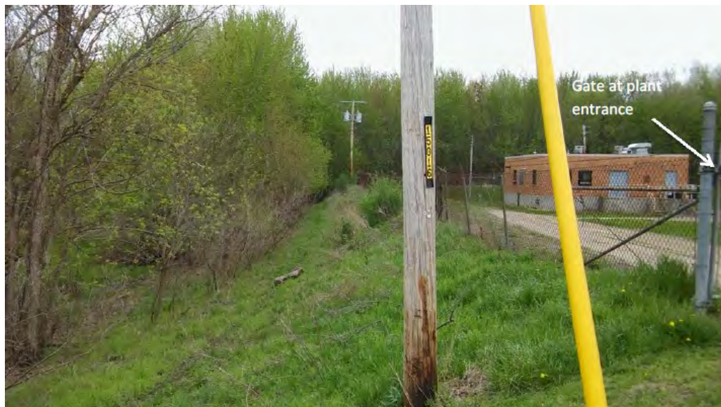
Photo 14: Facing south from northeast corner of levee.
