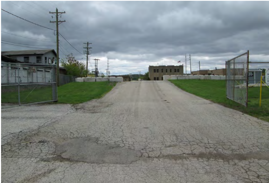
Photo 1: View south into WWTP; Control Building at center background.
