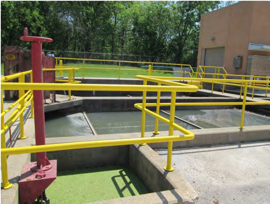
Photo 17: View east over c. 1939 Primary Clarifier; Grit Building at rear right.
