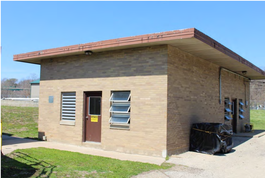
Photo 7: View north-northwest to south elevation of Blower Room Building.
