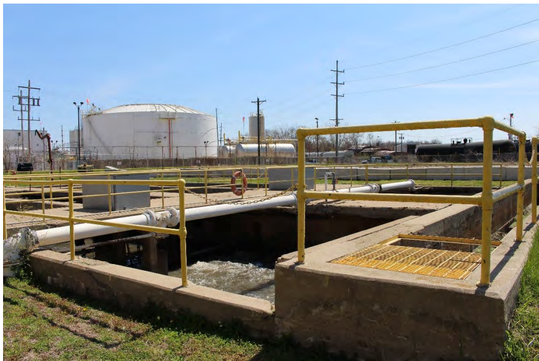
Photo 22: View southeast to Storage Tank.
