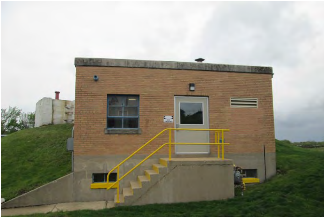
Photo 11: View southwest to northeast elevation of c. 1939 Boiler Room Building.
