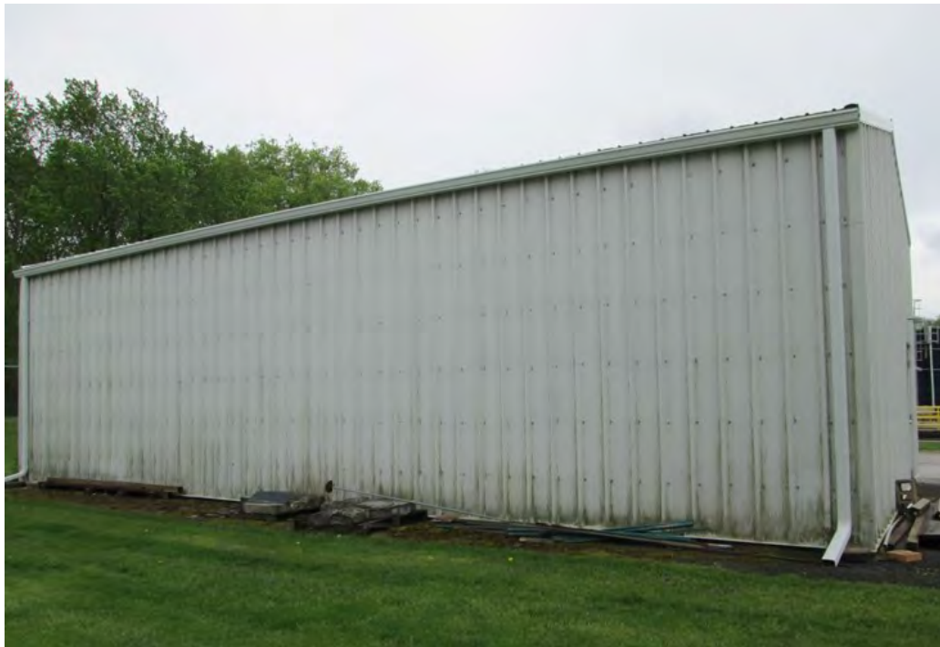
Photo 4: View southeast to north elevation of Storage Building.
