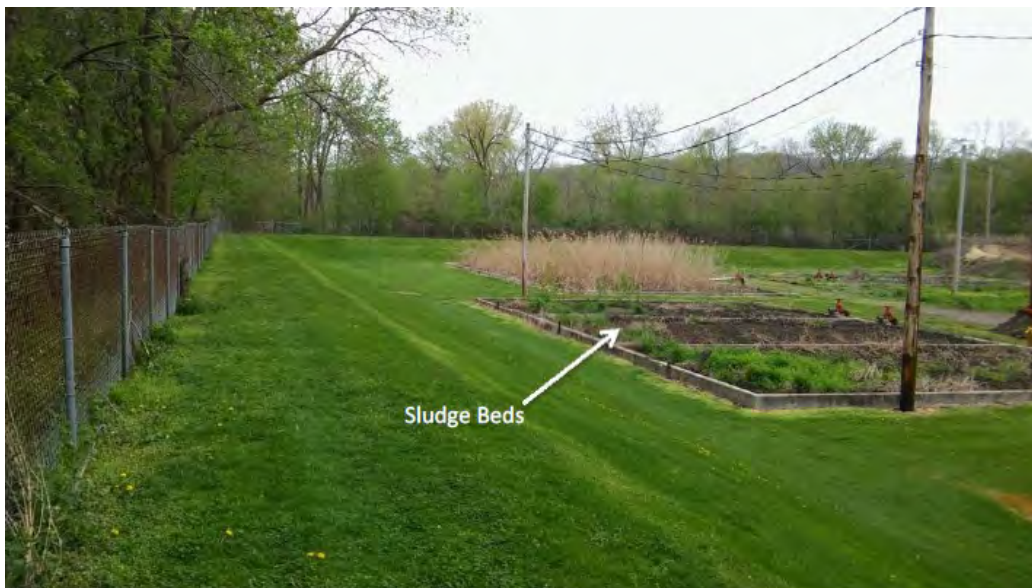
Photo 12: Facing west along top of southeast corner of levee.
