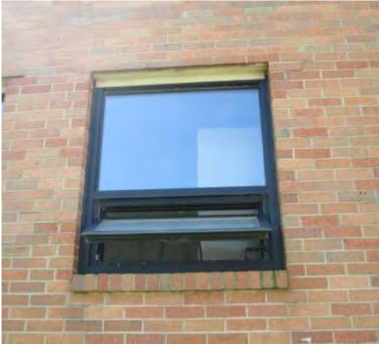
Photo 4: Detail view of vinyl window on north elevation of Blower Building.
