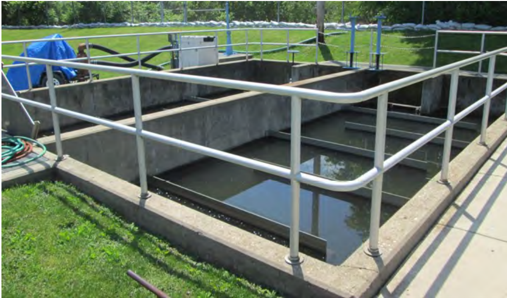
Photo 19: View southeast across c. 1974 Chlorine Contact Tank.
