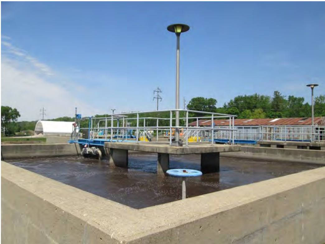
Photo 20: View northwest across c. 1974 Aeration Tank.
