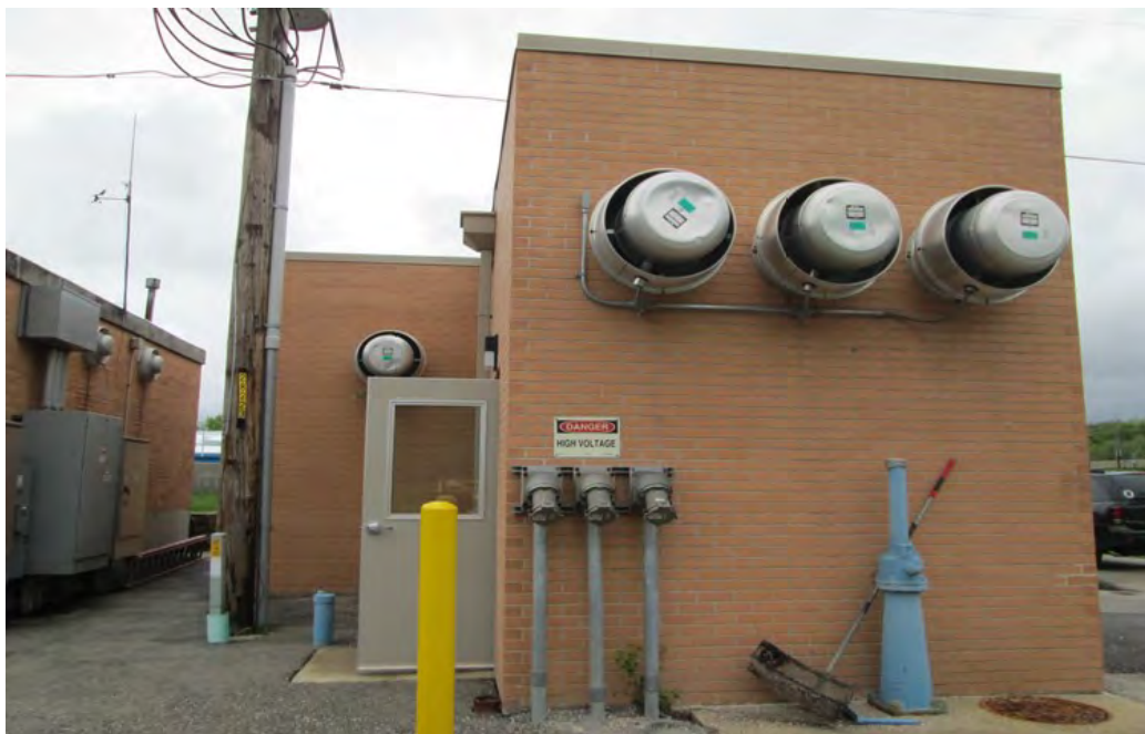
Photo 8: East elevation of Raw Sewage/Bar Screen Building.
