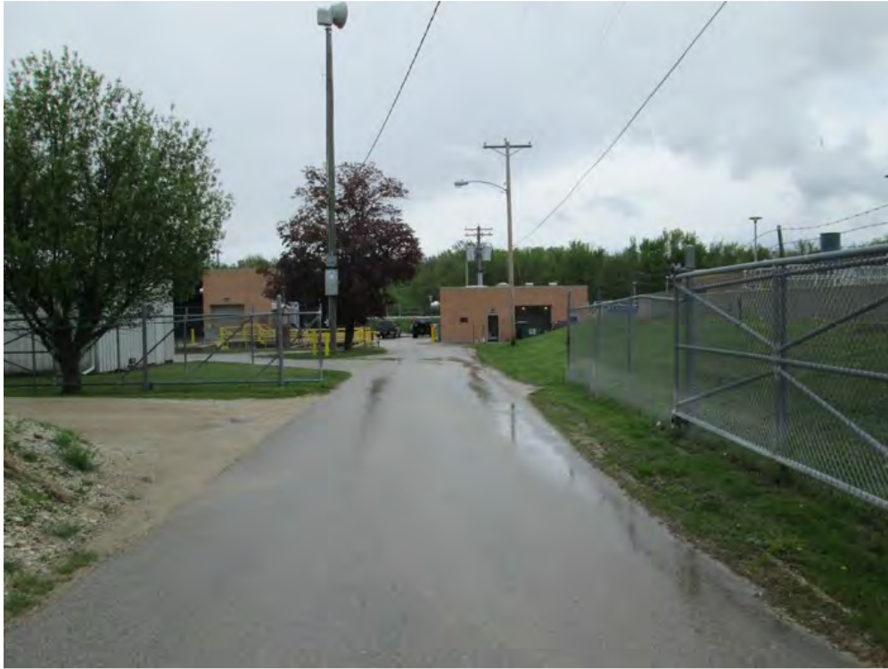
Photo 1: View south into east entrance to Marseilles WWTP.
