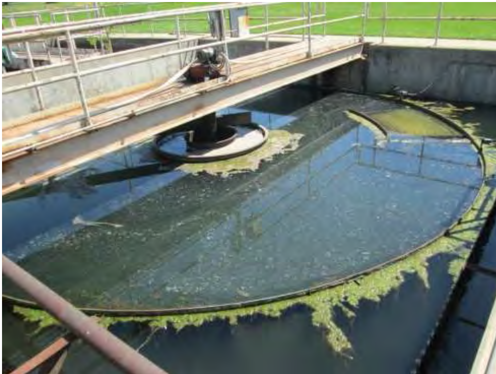
Photo 10: View to northeast across primary clarifier.
