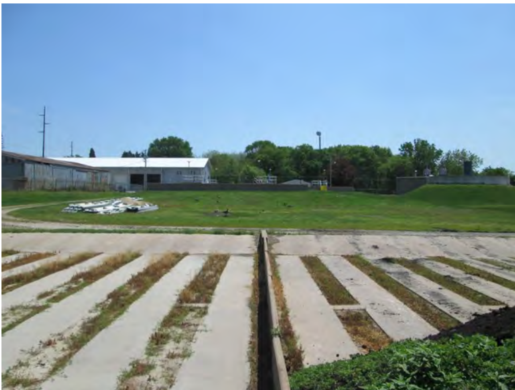
Photo 26: View east across Sludge Drying Beds.
