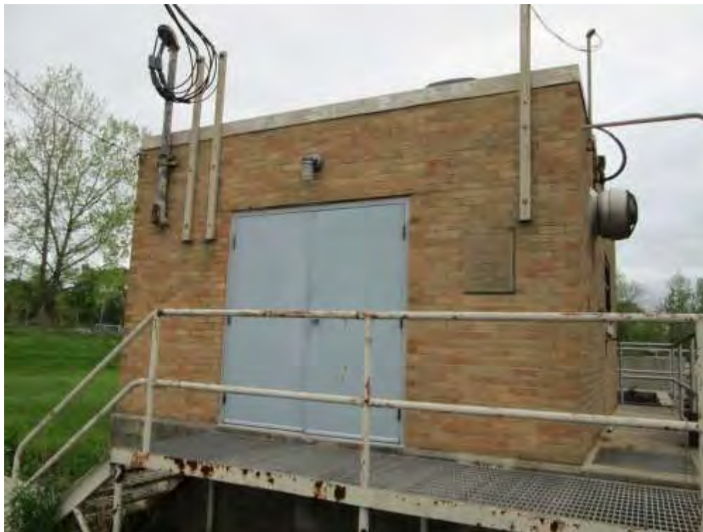
Photo 6: View east-northeast to west elevation of Lab and Pump Building.
