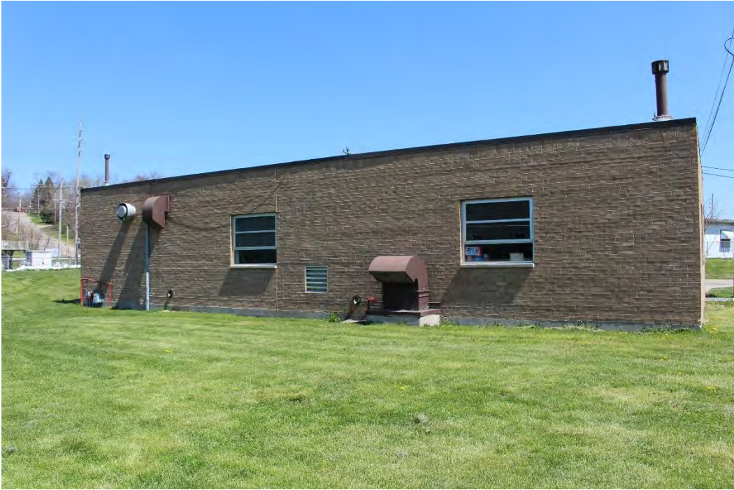
Photo 3: West elevation of Grit Building.
