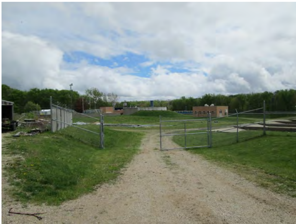
Photo 2: View southeast into west entrance to Marseilles WWTP.
