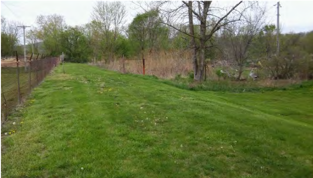
Photo 15: Facing west along levee at north facility boundary.
