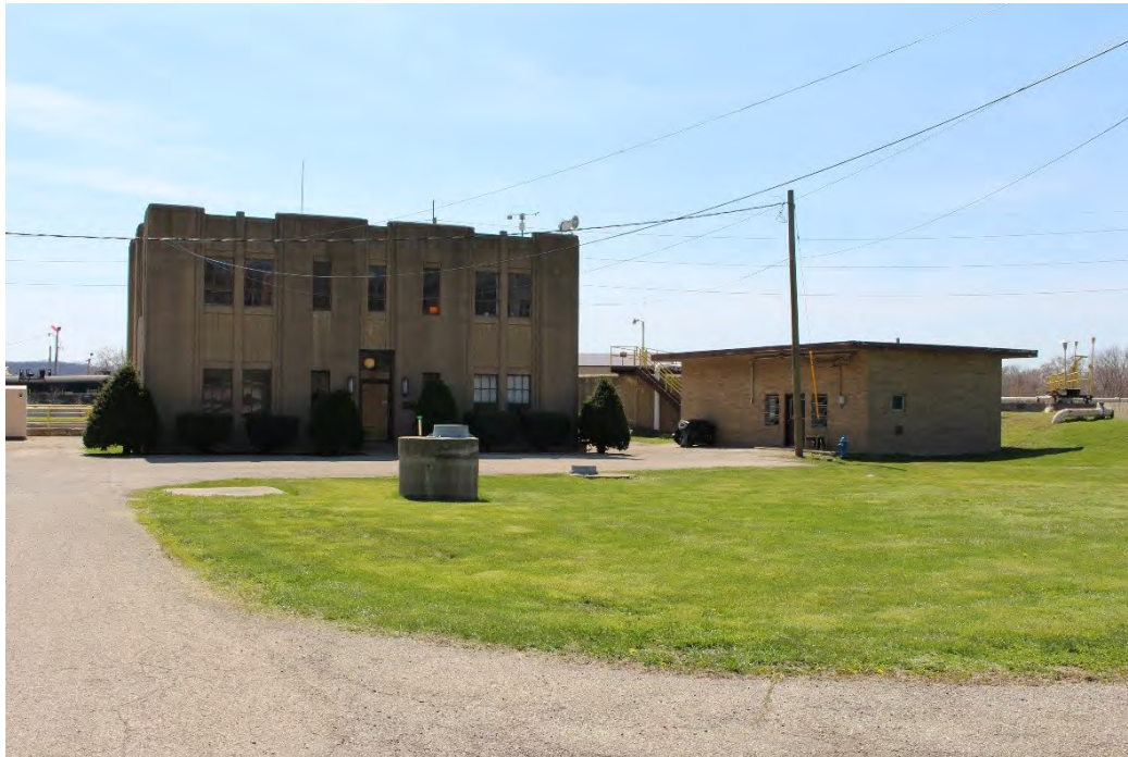
Photo 13: View south-southwest toward Control Building (left) and Blower Room Building (right).
