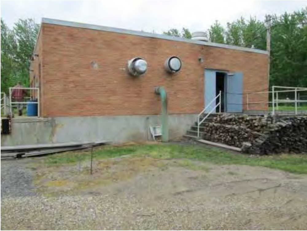
Photo 3: View east-southeast to west elevation of Blower Building.
