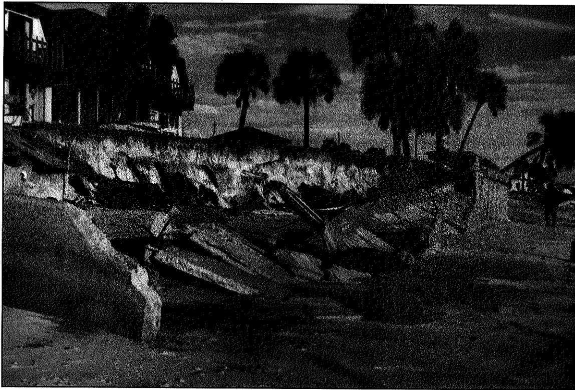
Figure 2-15 Fractured seawall, damaged by storm forces. Note the erosion of the bank behind the wall.
