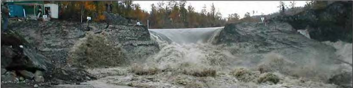
Figure 20. Embankment cross sections at various times and photograph of embankment as the embankment crest is breached, about time 1:45.
