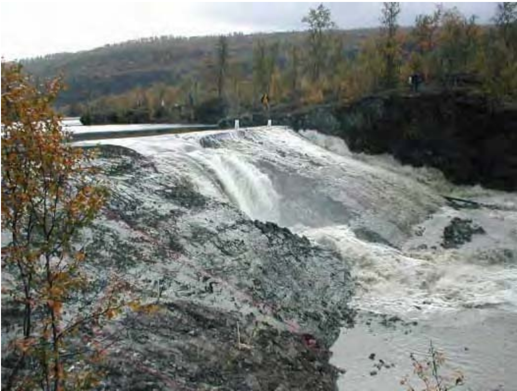
Figure 18. Erosion of the embankment after about one hour of overtopping.
