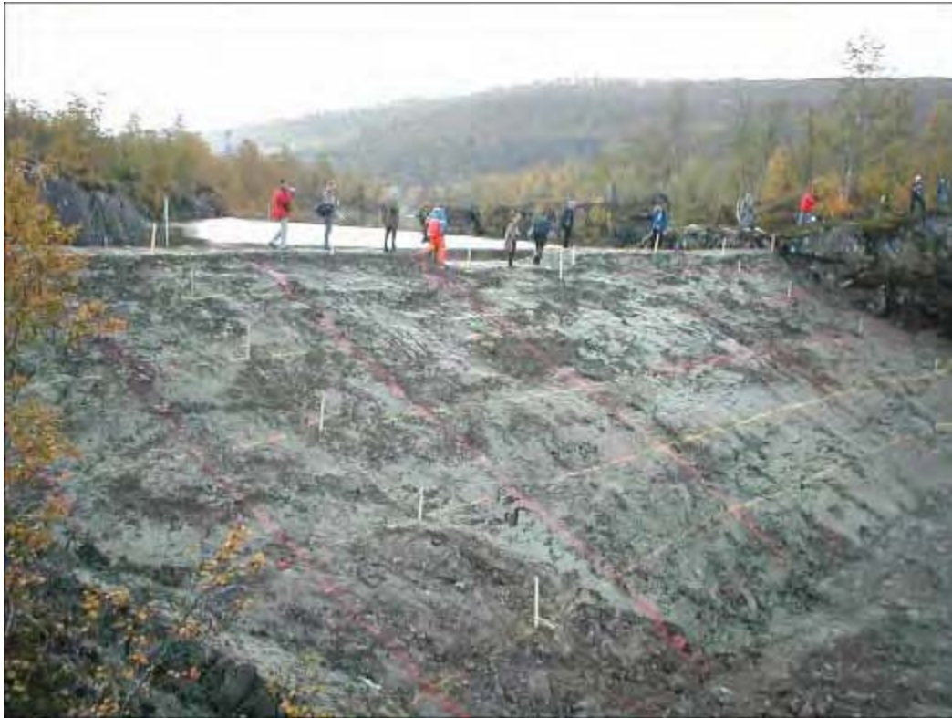
Figure 2. Experimental embankment at test site near Mo I Rana, Norway just before start of overtopping
