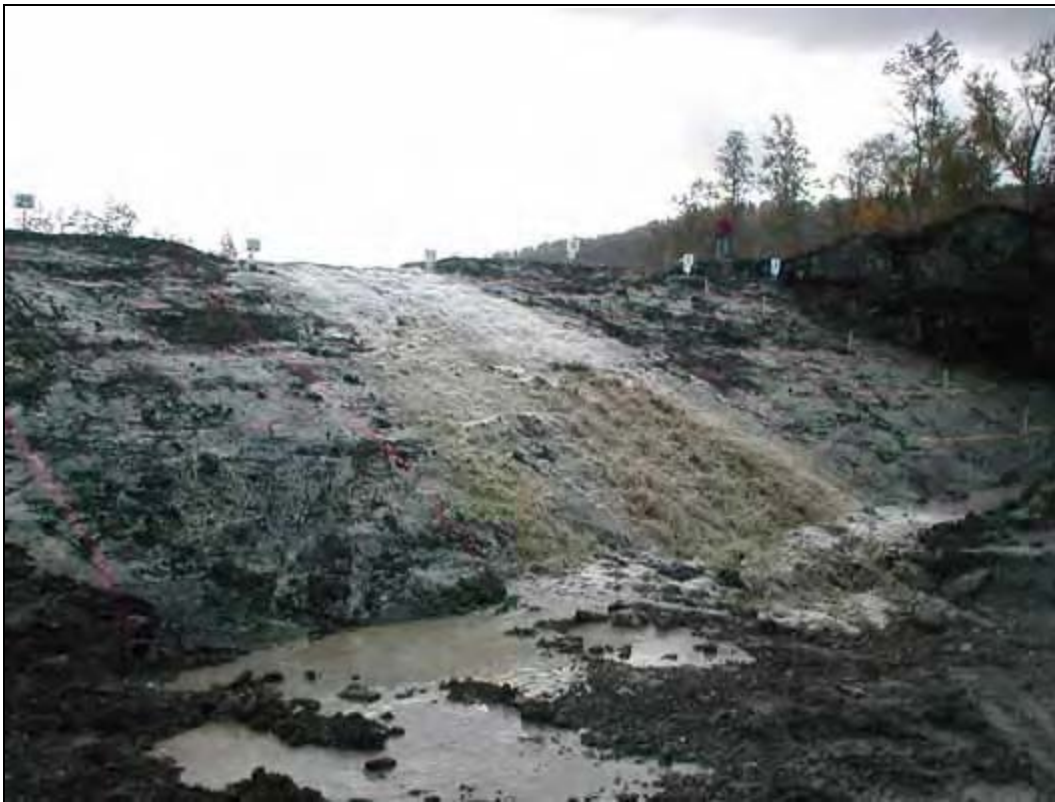
Figure 16. Start of overtopping flow.
