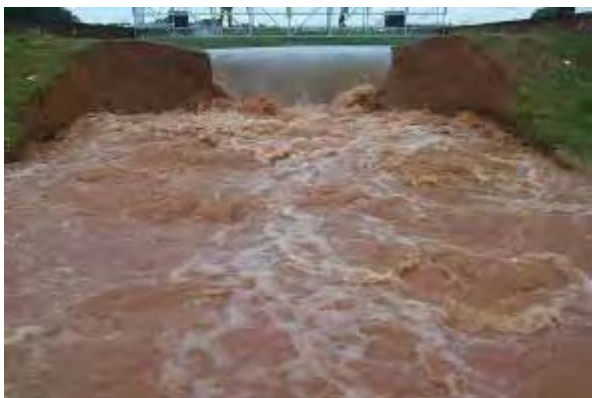
e) Flow through breach during Stage III at t = 40 min.
