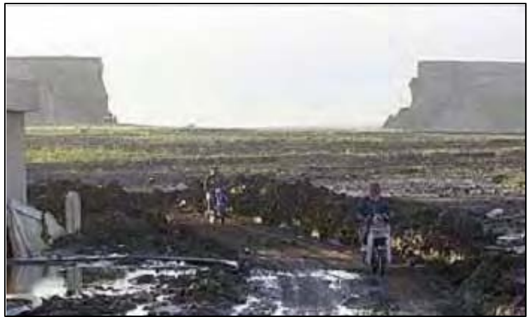
Figure 1. At least 20 people were killed when the Zeyzoun Dam in Syria failed on 4 Jun 2002. Several villages were flooded by depths up to four meters.
