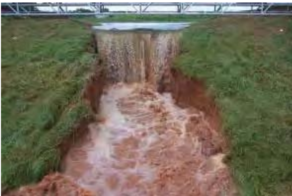
c) Headcut at downstream crest, transition from Stage I to Stage II at t = t_1 = 16 min.
