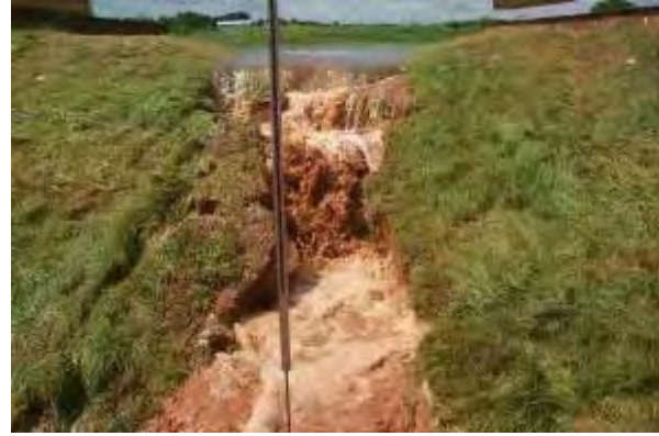
b) Consolidation of small overfalls during Stage I at t = 13 min
