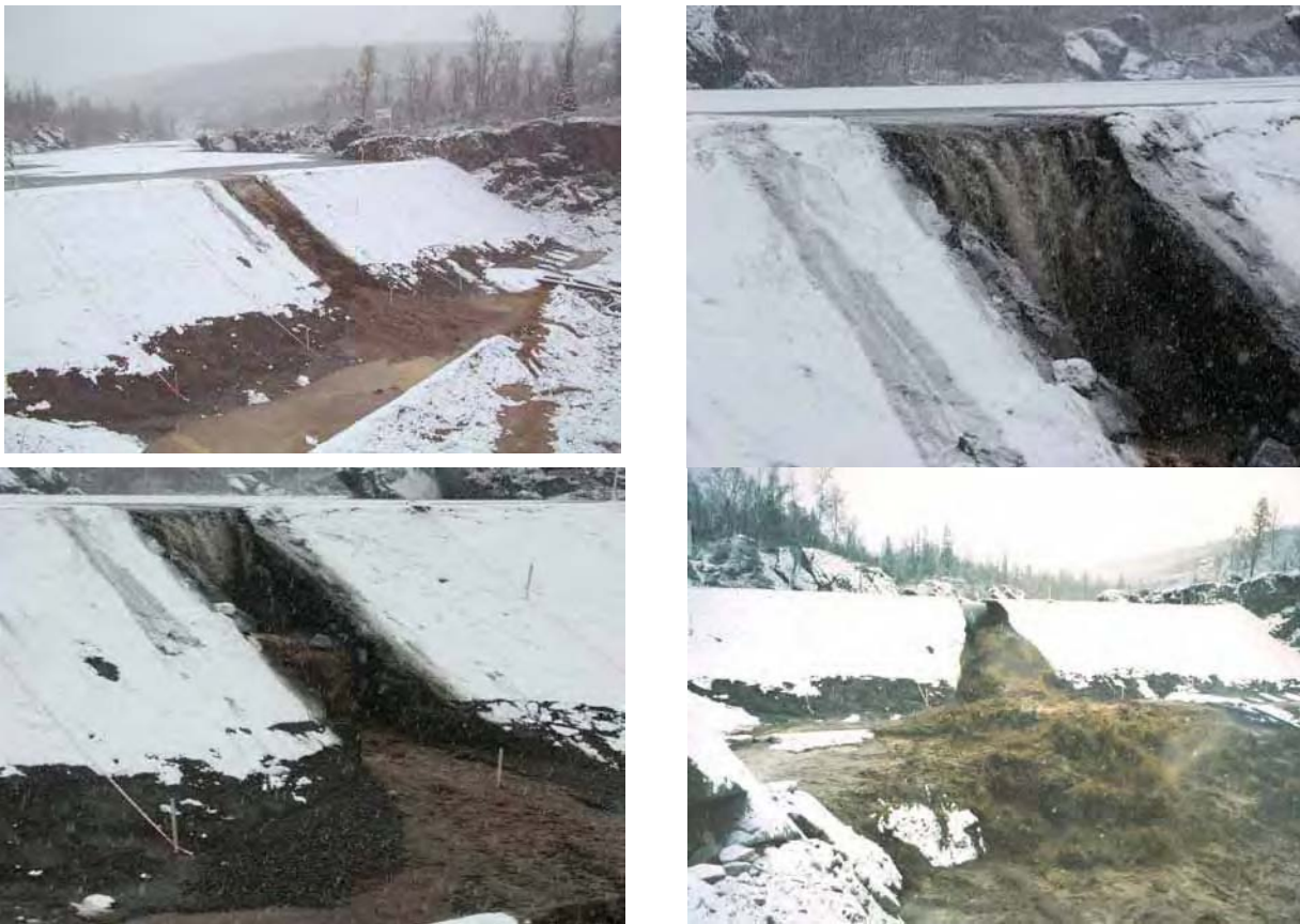
Figure 9 Pictures taken during the test of the gravel dam
