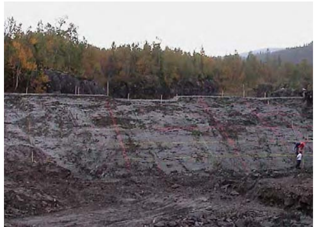
Figure 10. Embankment overtopping setup.
