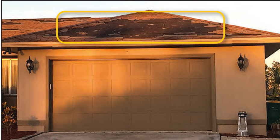
Figure 4-12: House with shingle loss near main ridge and between roof hips (yellow oval) (EWS = 109 mph; EDWS = 170 mph) (Marco Island)
