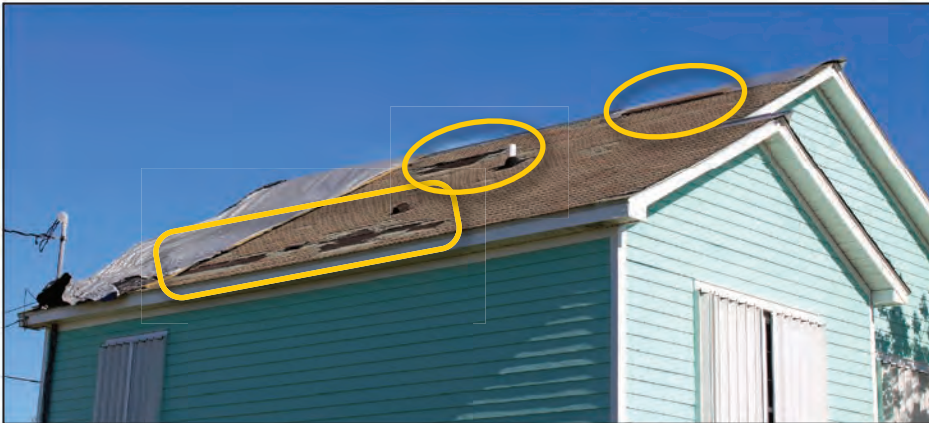
Figure 4-8: Asphalt shingle loss shown inside yellow ovals for house shown in Figure 4-7 (EWS = 111 mph; EDWS = 180 mph) (Big Coppitt Key)
