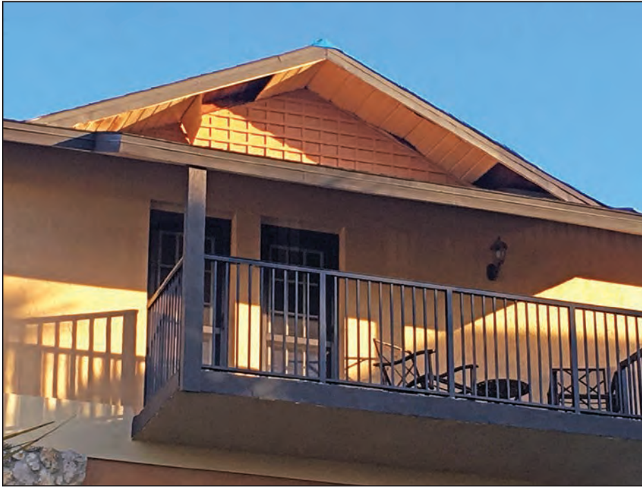
Figure 4-25: Metal soffit panel loss apartment gable end overhang (EWS = 104 mph; EDWS = 166 mph) (Naples)
