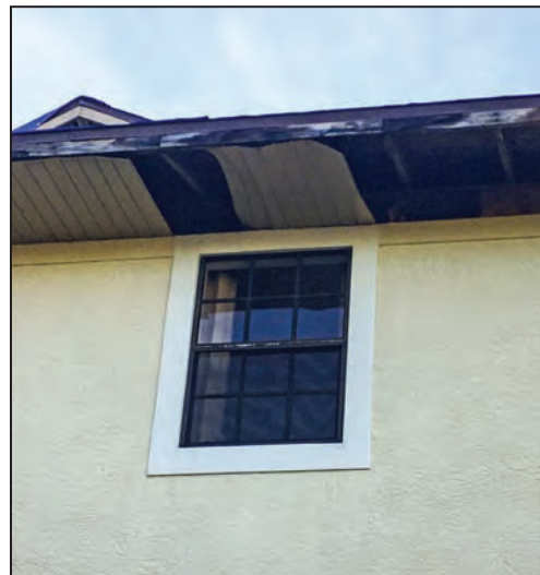
Missing metal soffit panels are shown below damaged fascia; located on the other side of the corner shown in left image.
