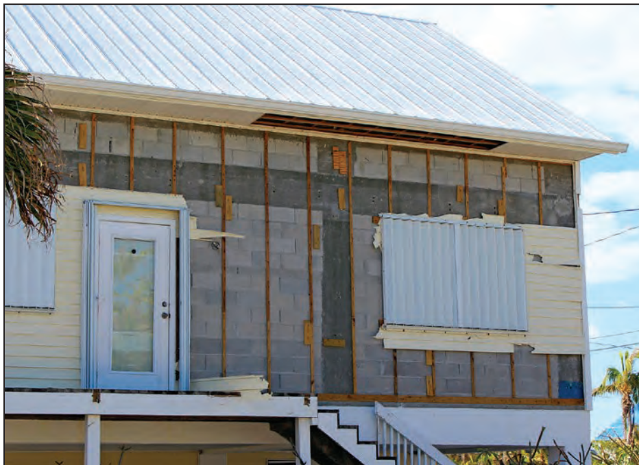
Figure 4-31: House with irregular fastener pattern and apparent lack of a proper starter strip (EWS = 114 mph; EDWS = 180 mph) (Little Torch Key)
