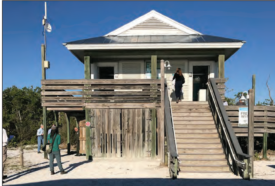
Figure 3-34: Elevated restrooms with ground-level enclosure. Lovers Key State Park restroom (Site 2; Lee County) enclosure sustained shallow flooding but no damage during Hurricane Irma.
