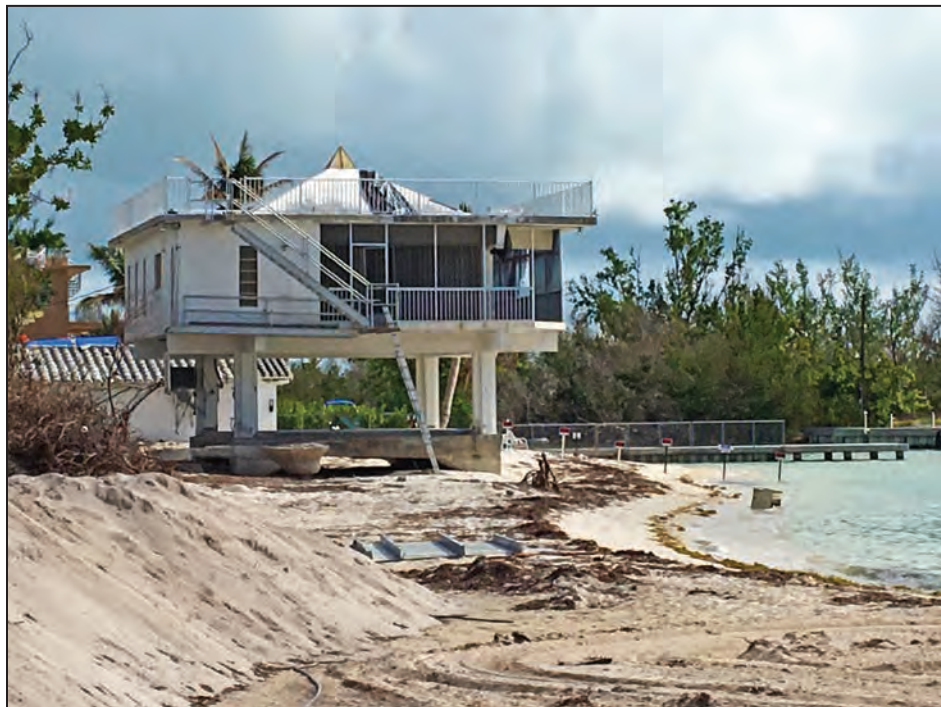
Figure 3-16: Erosion was likely due to wave attack around the foundation of this house on Sombrero Beach Road (Marathon, FL)
