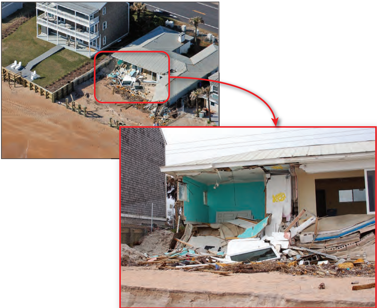
Figure 3-29: House on a shallow foundation that collapsed after it was undermined following failure of the bulkhead during Hurricane Irma (St. Johns County, FL)
