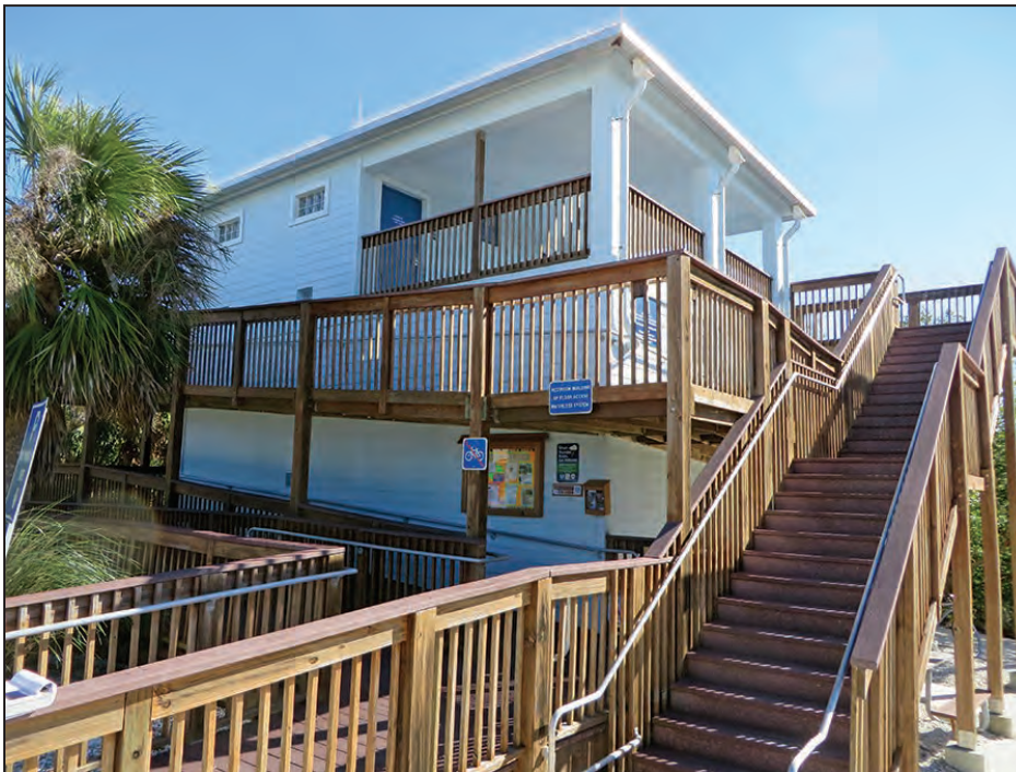
Figure 3-33: Elevated restrooms with ground-level enclosure. Bunche Beach Preserve restroom (Site 1; Lee County), where the degree of flooding in the enclosure, if any, would have been shallow.
