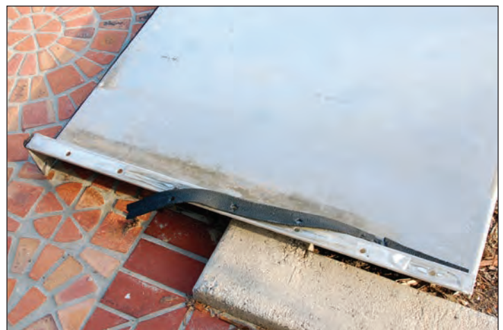
Figure 3: Torn gasket on metal flood panel after panel was removed. Gasket must be replaced before the next deployment.
