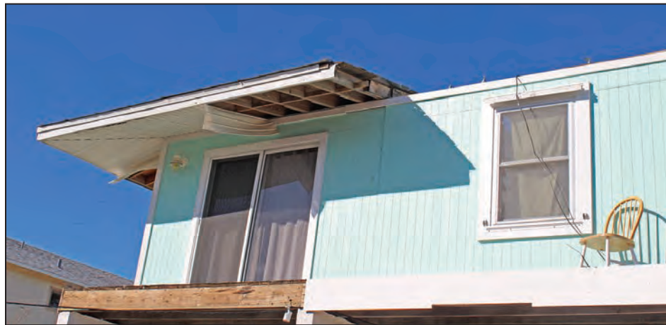
Figure 4-3: South end of east-facing wall; the south end of the roof remained in place (EWS = 113 mph; EDWS = 180 mph) (Cudjoe Key)
