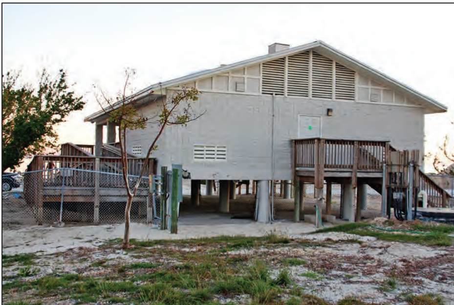
Figure 3-40: Elevated Long Key State Park restroom without ground-level enclosure and that sustained no flood damage during Hurricane Irma (Site 9; Monroe County)
