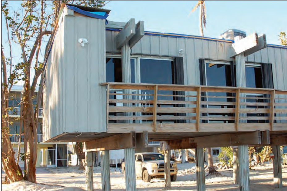
Figure 3-7: Example of a breakaway wall that was reported by a local code official to have performed as intended (Lower Matecumbe Key, FL)
