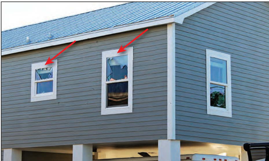
Figure 4-32: Residence with two windows where the outer panes were broken (see red arrows) but the inner panes stayed intact (EWS = 113 mph; EDWS = 180 mph) (Ramrod Key)
