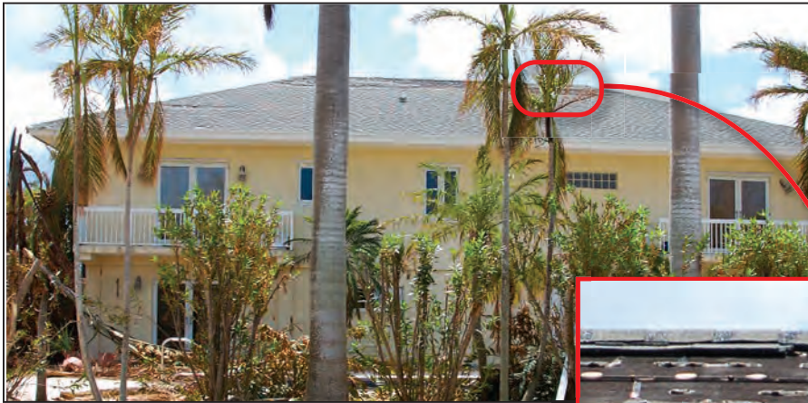
Figure 4-10: Residence that lost shingles near the ridge (EWS = 113 mph; EDWS = 180 mph) (Sugarloaf Key)
