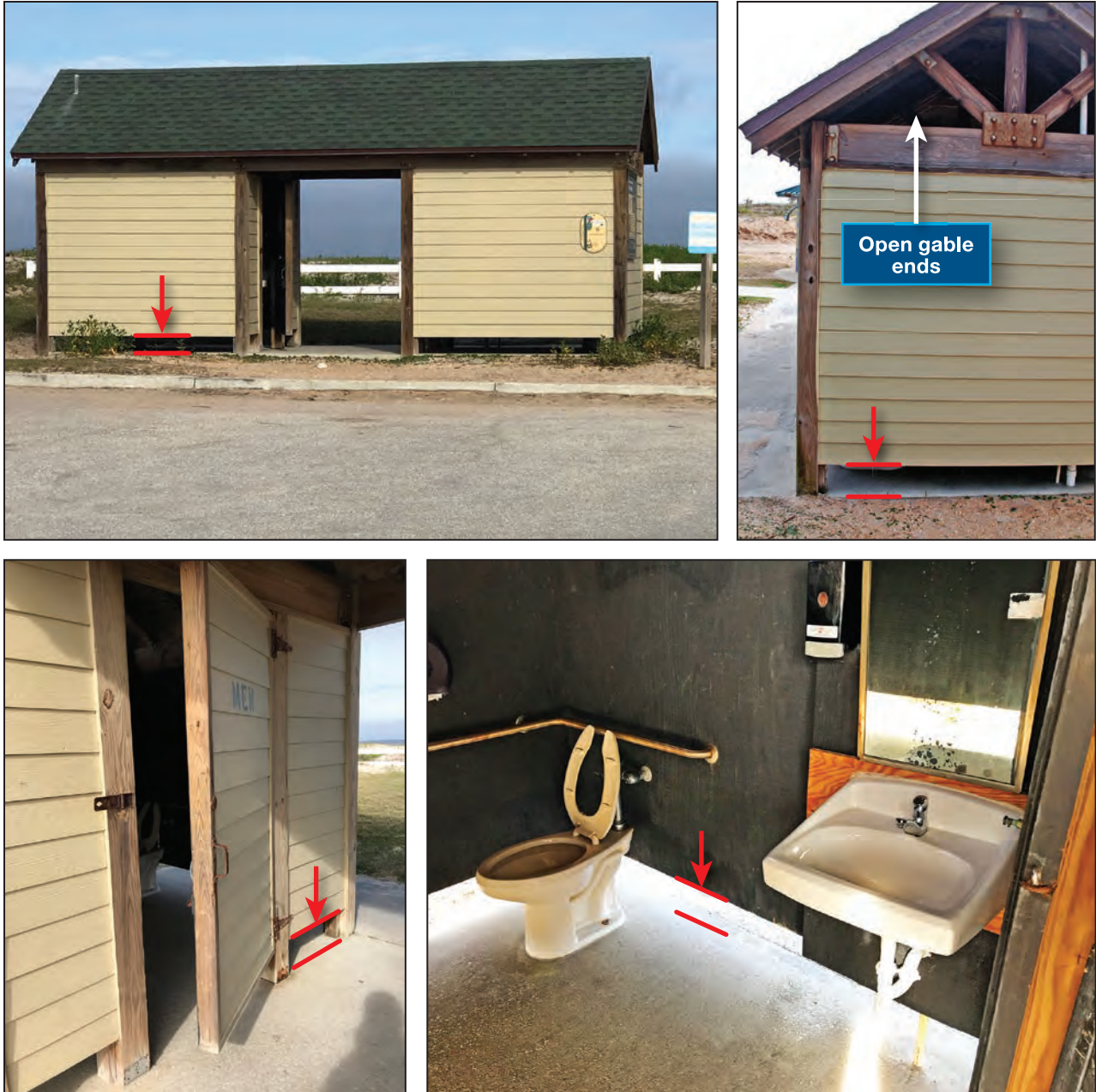
Exterior and interior photos of a restroom building at Surfside Park, St. Johns County. The wood frame outer walls do not extend to the floor slab (red arrows), and gable ends are open, allowing light and air to enter the restrooms. There is no electric service to the restrooms. The building likely sustained no flood damage during Irma.
