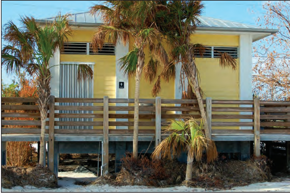
Figure 3-39: Elevated restrooms at Sombbrero Beach Park without ground-level enclosure and that sustained no flood damage during Hurricane Irma (Site 7; Marathon)
