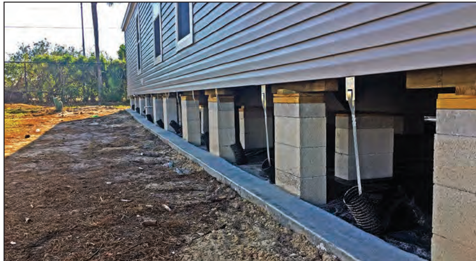
Figure 4-40: Consistent anchorage pattern observed on a new MH unit installation (EWS = 105 mph; EDWS = 164 mph) (Collier County)
