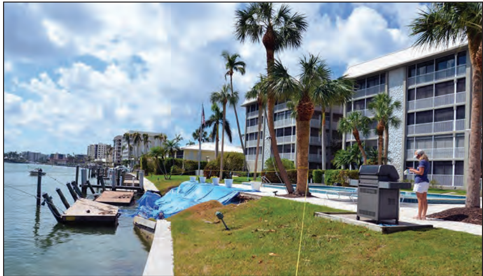
Figure 3-27: Failure of bulkhead (anchor system) (Naples, FL)
