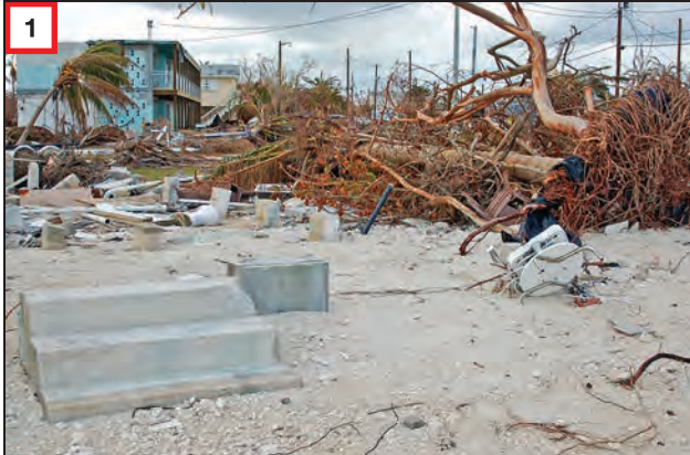
1 House near shoreline and subject to wave action/ high water velocity was washed off its foundation and destroyed.
