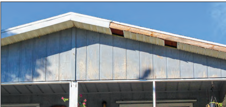
Figure 4-23: House with metal soffit loss below missing fascia cover (EWS = 114 mph; EDWS = 180 mph) (Big Pine Key)
