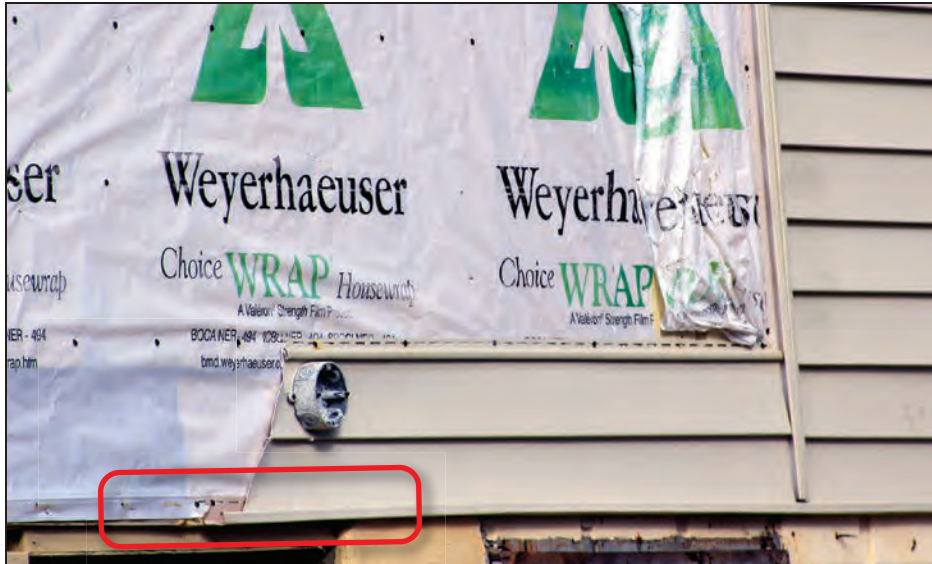
Figure 4-30: House that lacked a proper starter strip, as shown in the red outline (EWS = 114 mph; EDWS = 180 mph) (Little Torch Key)
