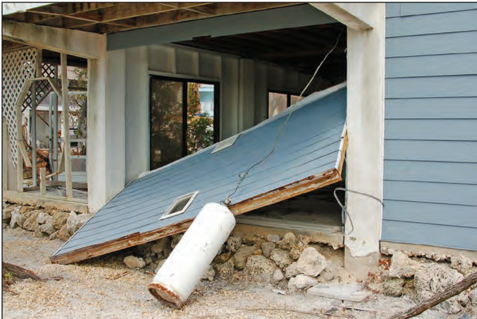
Figure 3-8: Example of partial failure of breakaway wall, with no associated damage to main structure observed (Cudjoe Key, FL)
