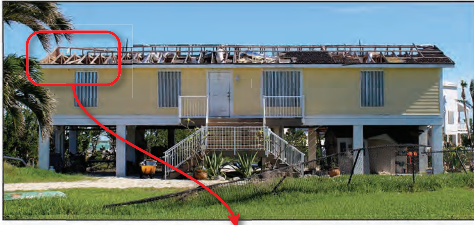
Figure 4-1: House with structural damage to roof system (EWS = 113 mph; EDWS = 180 mph) (Sugarloaf Key)
