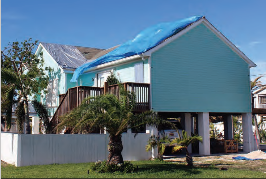
Figure 4-7: The MAT could not observe much of the asphalt roof damage on this house because it was covered by a tarp (EWS = 111 mph; EDWS = 180 mph) (Big Coppitt Key)
