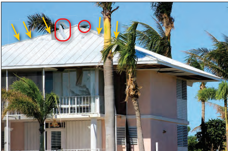
Figure 4-16: House with damaged metal roof system (EWS = 113 mph; EDWS = 180 mph) (Sugarloaf Key)
