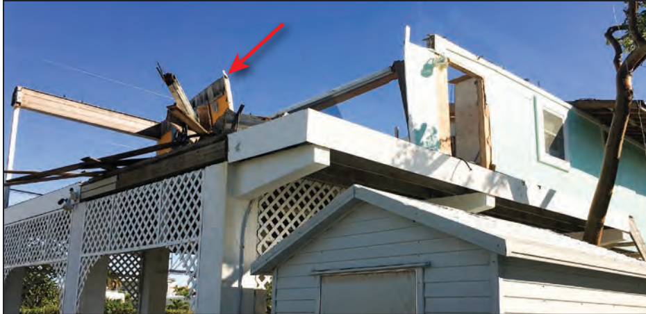
Figure 4-5: Remainder of the screened porch and exterior wall (EWS = 113 mph; EDWS = 180 mph) (Cudjoe Key)
