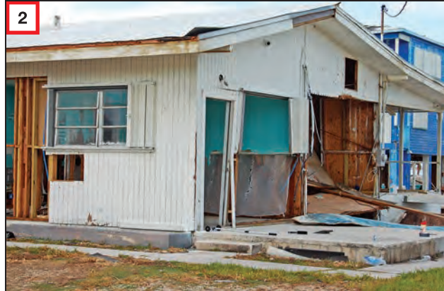
2 Inundation, water velocity, and debris damage to buildings situated farther from the shoreline.
