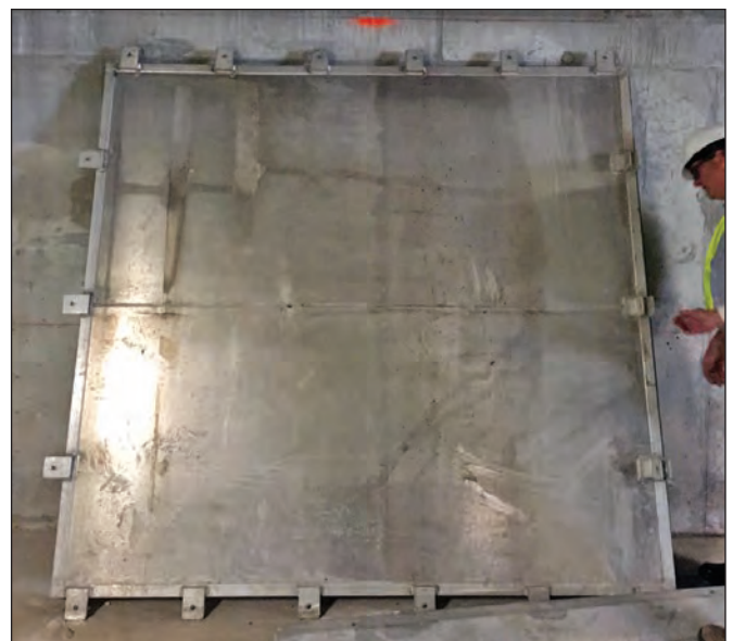
Figure 1: Large (6 feet high x 6 feet wide) metal flood panel requiring special equipment for installation
