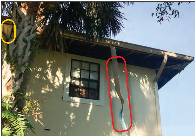
Dangling fascia cover (red outline) is shown adjacent to missing metal soffit panels near the corner of a Naples apartment building (yellow outline indicates intact soffit panels).
