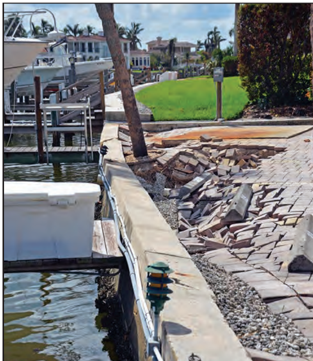
Figure 3-28: Bulkhead toe failure (insufficient embedment) (Naples, FL)
