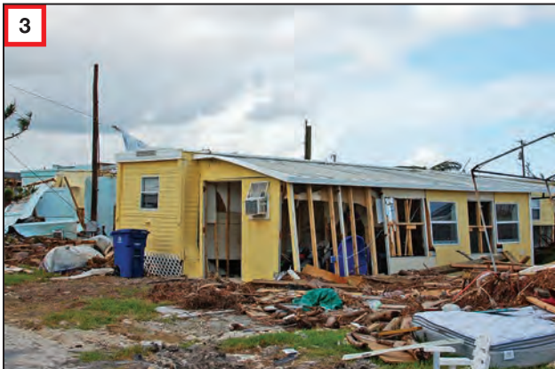
3 Inundation, water velocity, and debris damage to buildings situated farther from the shoreline.
