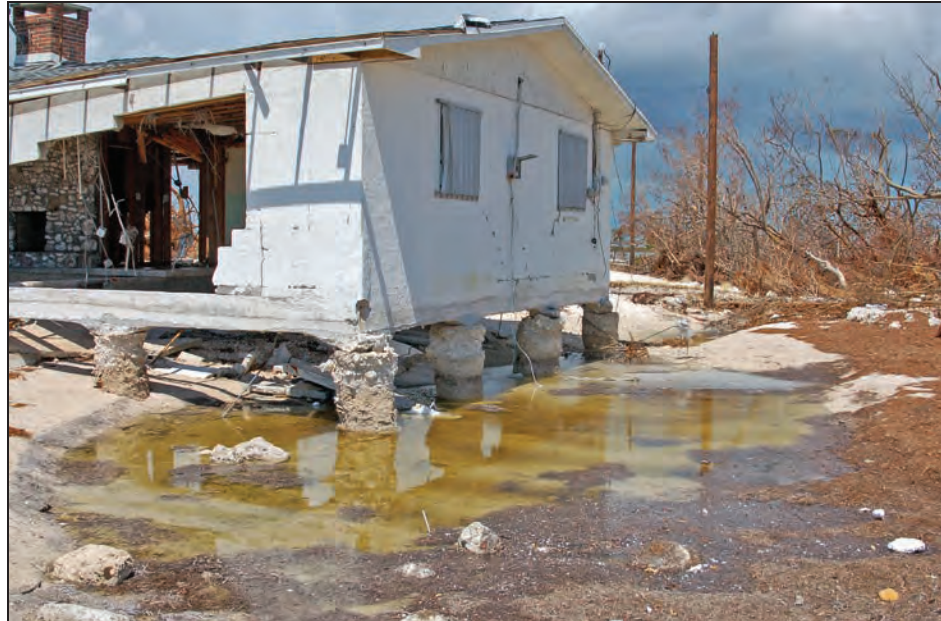
Figure 3-15: Scour was likely due to waves and high-velocity flow at this house on Long Beach Drive (same house is shown in Figure 3-6) (Big Pine Key, FL)
