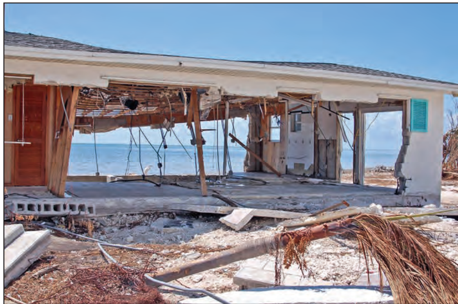
Figure 3-6: House constructed at grade where the masonry walls parallel to the shoreline were destroyed; this house was near the house shown in Figure 3-5 (Big Pine Key, FL)
