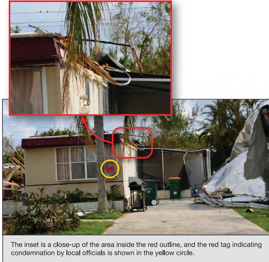
Figure 4-46: MH unit where carport detached from the unit, opening the building envelope across the top of a wall (EWS = 105 mph; EDWS = 166 mph) (Collier County)
