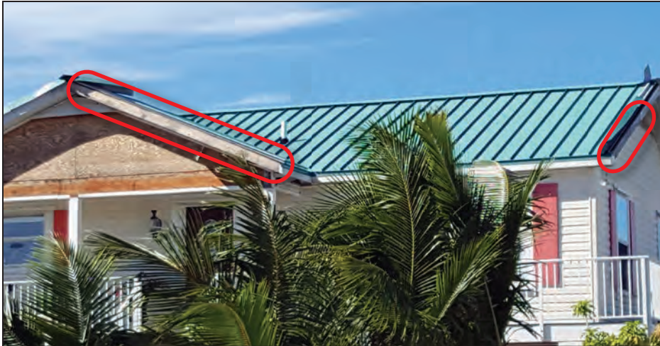
Figure 4-15: House with separated metal roof trim and missing fascia cover (red ovals) along gable end. (EWS = 113 mph; EDWS = 180 mph) (Sugarloaf Key)
