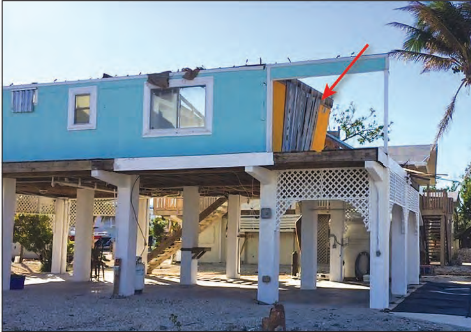
Figure 4-4: North end of east-facing wall where the roof was (EWS = 113 mph; EDWS = 180 mph) (Cudjoe Key)
