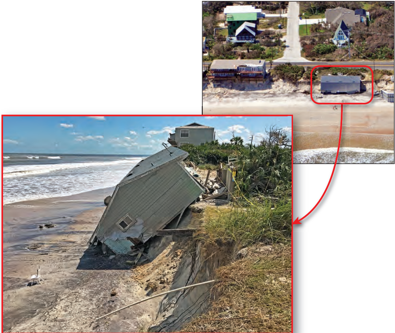
Figure 3-20: Collapsed house on shallow foundation that was undermined by erosion induced by Hurricane Irma (Vilano Beach, FL)
