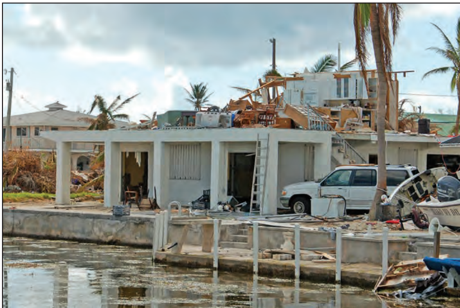
Figure 3-12: Car and debris that washed into a house (Big Pine Key, FL)
