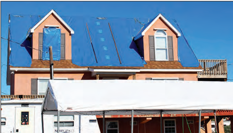
Figure 4-9: House with asphalt shingle loss as evidenced by tarp (EWS = 120 mph; EDWS = 180 mph) (Marathon)
