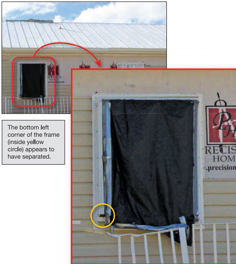
Figure 4-35: House with impact-resistant shutter system damaged by wind-borne debris; opening was covered at the time the MAT visited (EWS = 114 mph; EDWS = 180 mph) (Little Torch Key)
