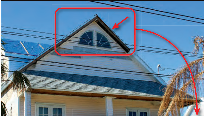
Figure 4-18: House that lost its soffit along the right side of the front-facing gable (EWS = 114 mph; EDWS = 180 mph) (Little Torch Key)
