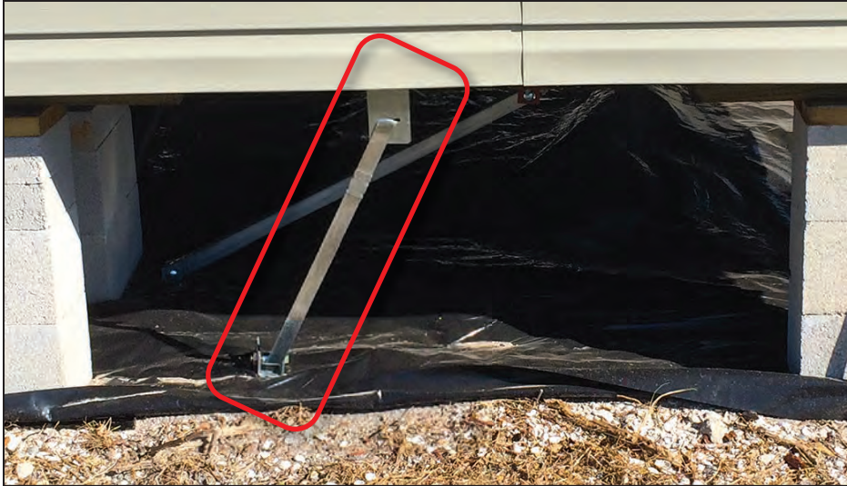
Figure 4-41: New MH unit installation with misaligned anchor strap installation (red outline) was otherwise anchored consistently with other post-Irma examples (EWS = 105 mph; EDWS = 164 mph) (Collier County)
