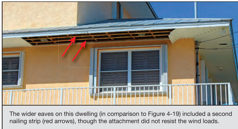
Figure 4-20: Dwelling with similar soffit panel attachment and loss as shown in Figure 4-19 (EWS = 113 mph; EDWS = 180 mph) (Sugarloaf Key)
