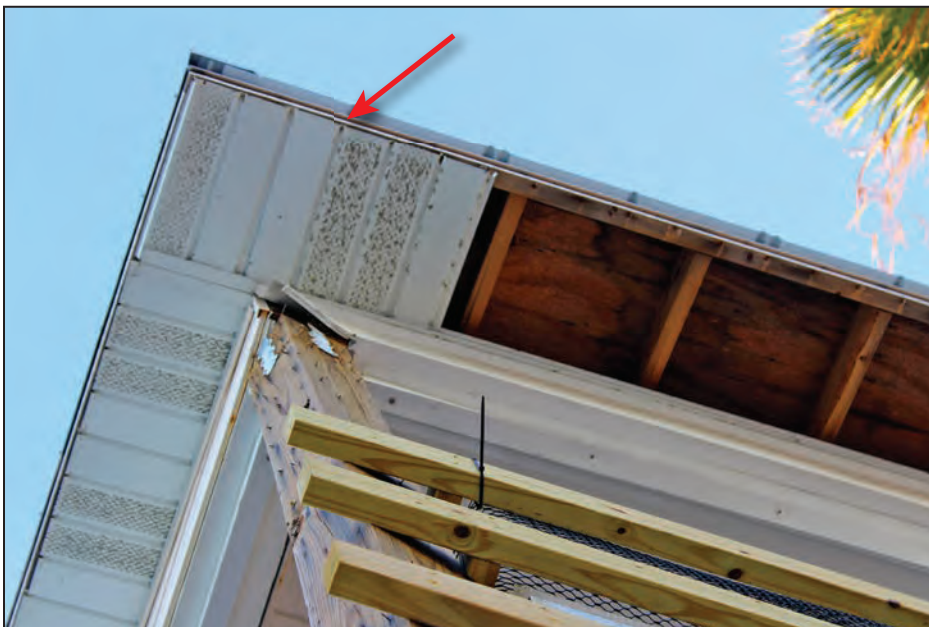
Figure 4-22: Metal soffit loss on house (EWS = 113 mph; EDWS = 180 mph) (Ramrod Key)
