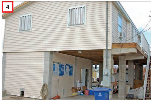
4 Minor enclosure damage to newer, elevated house situated away from the shoreline.
