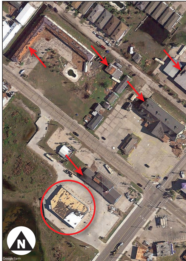
Figure 4-122: Aerial view of a pharmacy with roof damage (135 mph) (Port Aransas)
