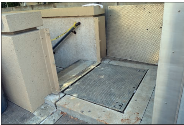
Floodgate protecting pedestrian access to the underground Green Parking Garage.
