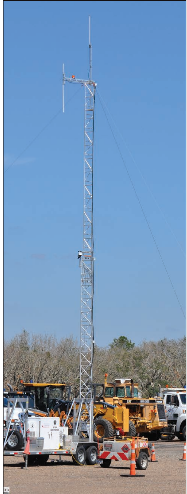
Figure 4-83: Portable communications tower
