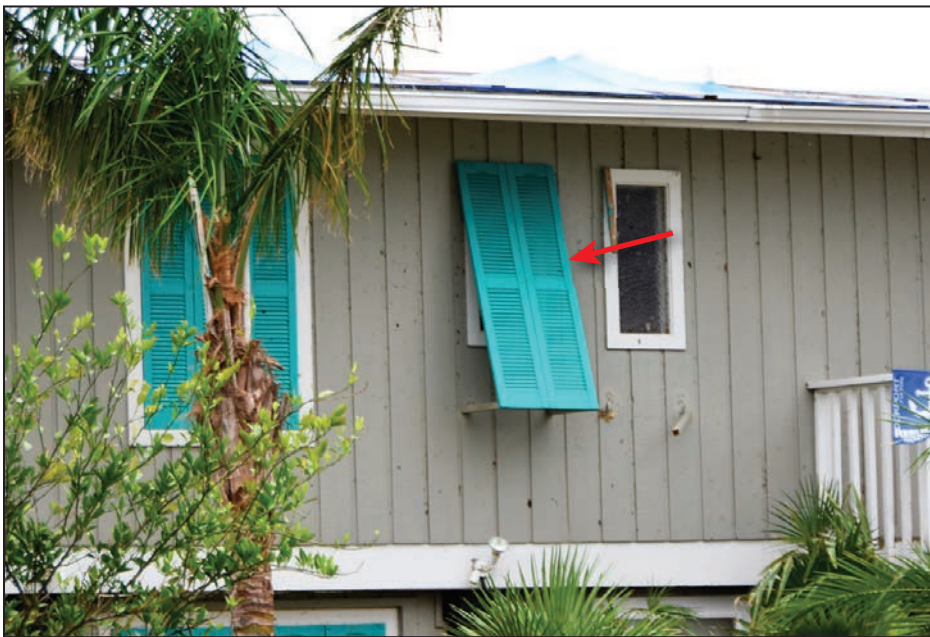
Figure 4-56: Operable Bahama shutters (red arrow) (Key Allegro)
