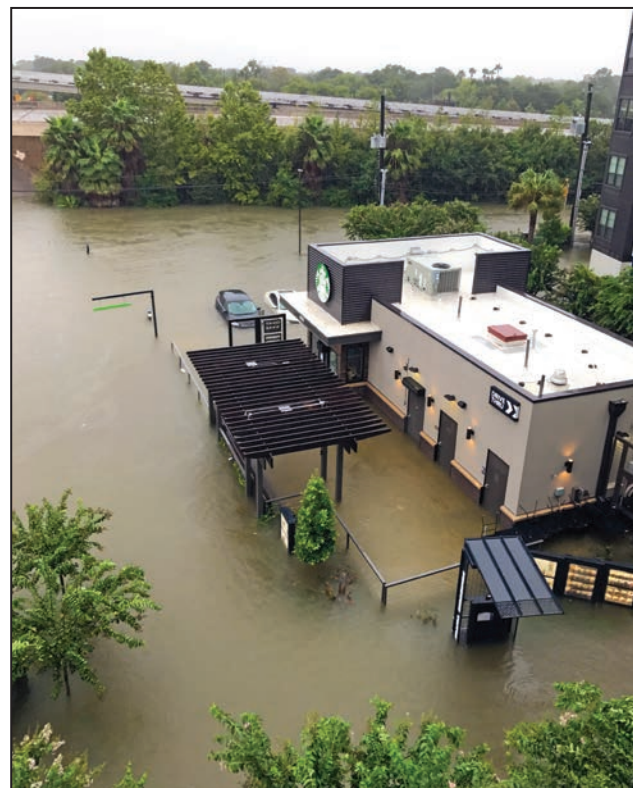
Figure 3-92: Starbucks during Hurricane Harvey flooding
