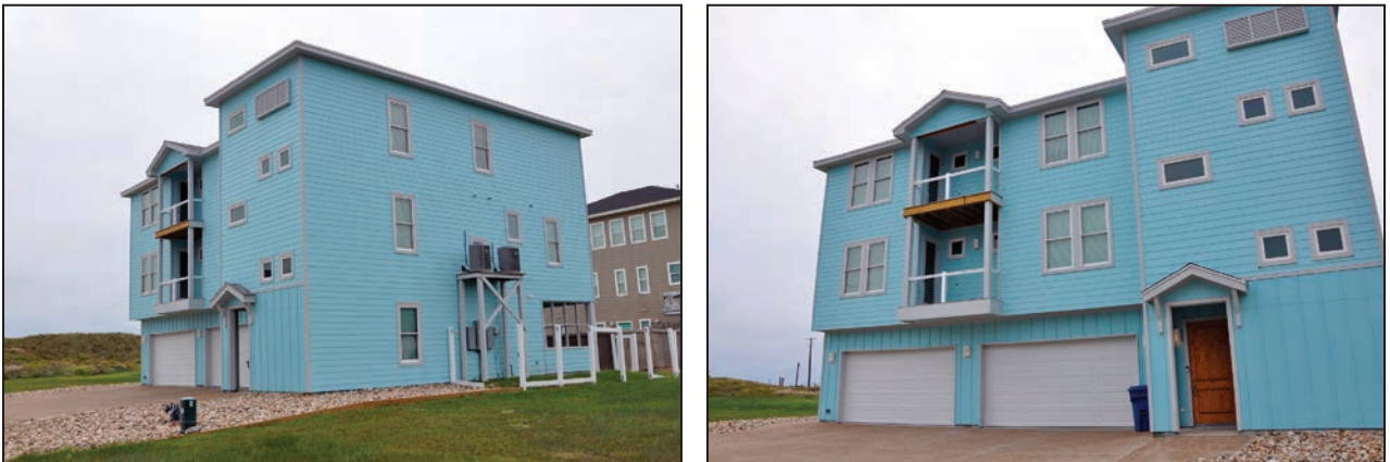
Figure 3-10: Relatively new house built in 2016 had limited exterior flood damage, yet interior repairs were required due to flood inundation and penetration of wind-driven rain [Zone AE]
