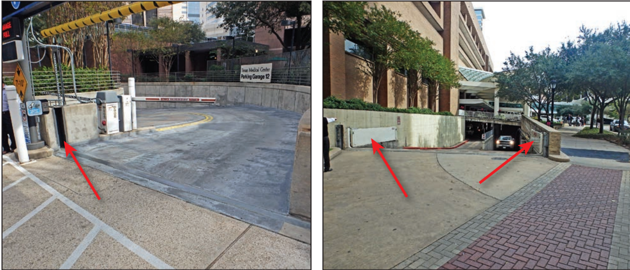
Figure 3-100: Flood log gate (left) and swing floodgate (right) at parking garage entrances
