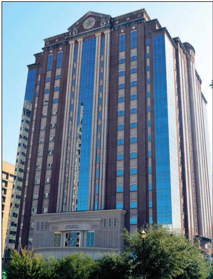
Figure 3-45: Harris County Civil Courthouse viewed from the southwest
