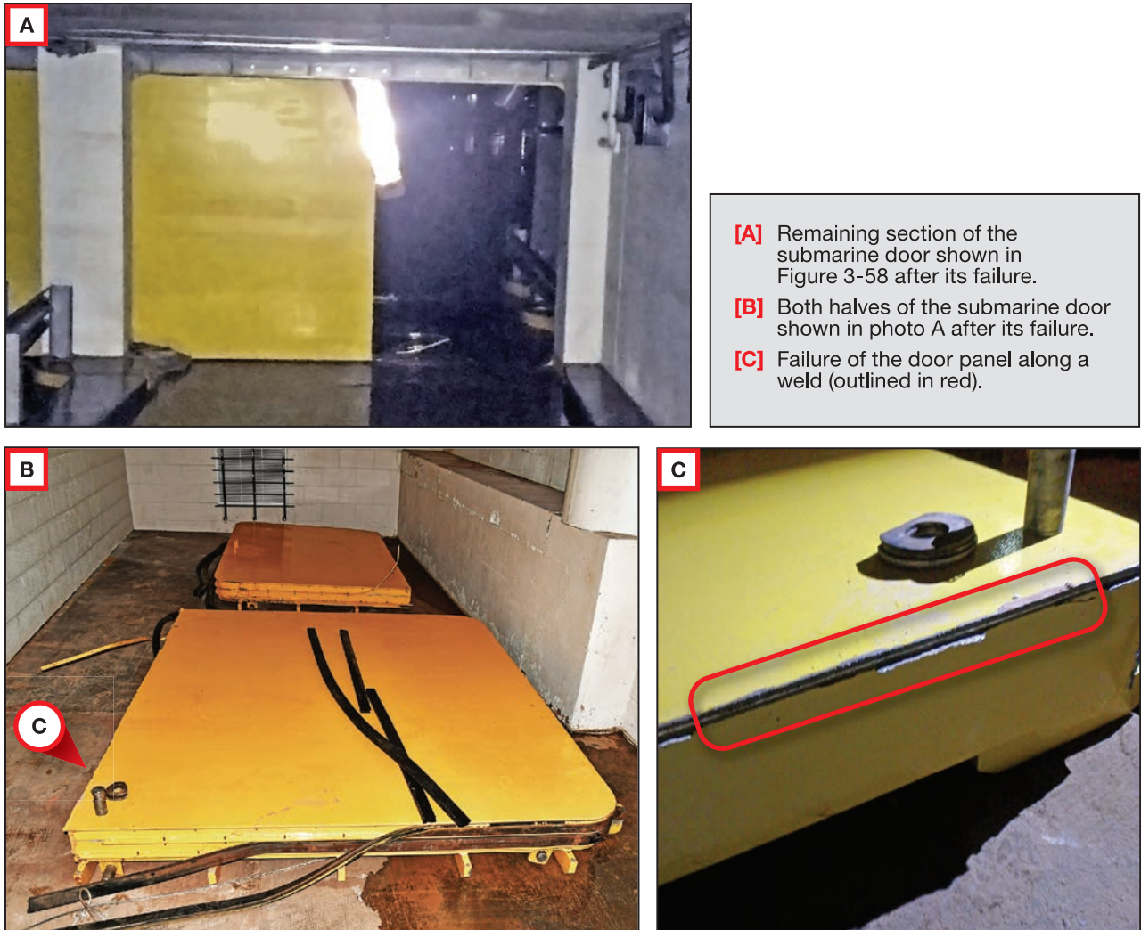
Figure 3-59: Submarine door shown in Figure 3-58 after its failure PHOTOGRAPHS COURTESY OF CARLOS GUTIERREZ, CSF CONSULTING
