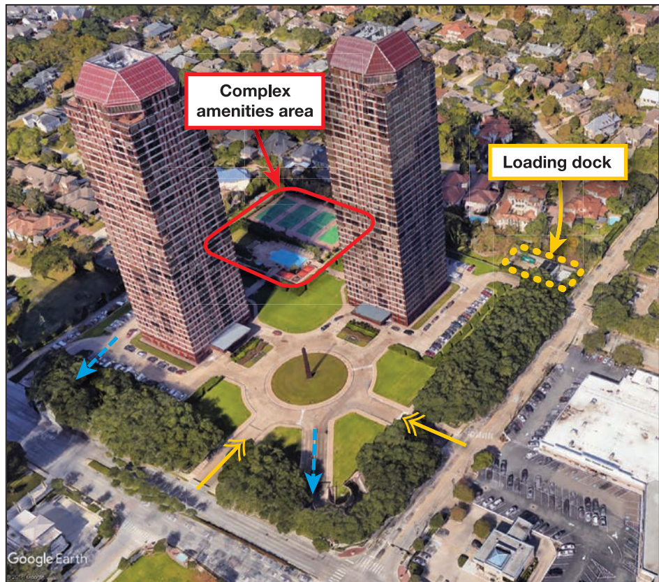
Figure 3-84: Four Leaf Towers Condominium Complex, where yellow double arrows indicate street-level access locations to the complex and blue dashed arrows indicate access to parking garage
