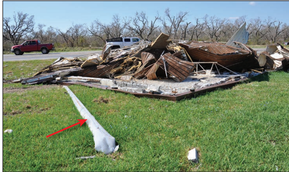
Figure 4-77: Wind-borne roof assembly debris (roof assembly is upside down)
