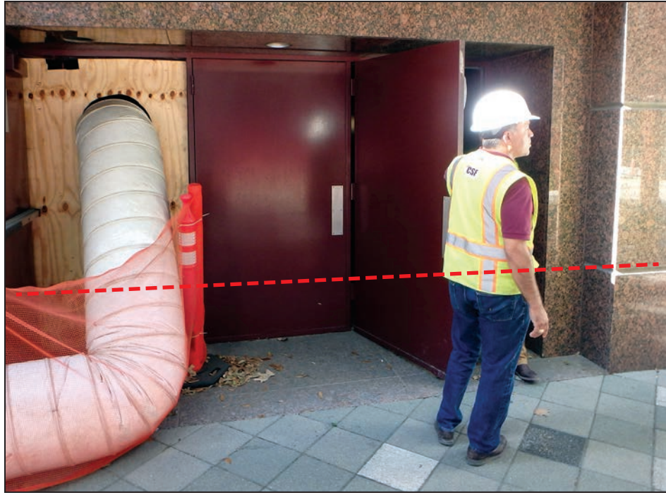
Figure 3-67: Emergency exit door along the east side of the Wortham Theater; the red line indicates the approximate HWM during Hurricane Harvey
