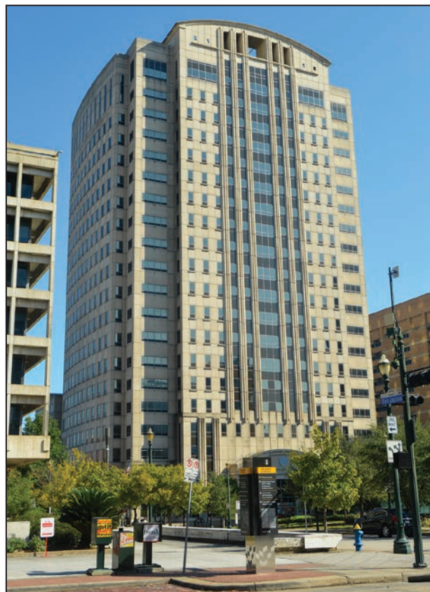
Figure 3-35: Harris County Criminal Justice Center viewed from the southwest
