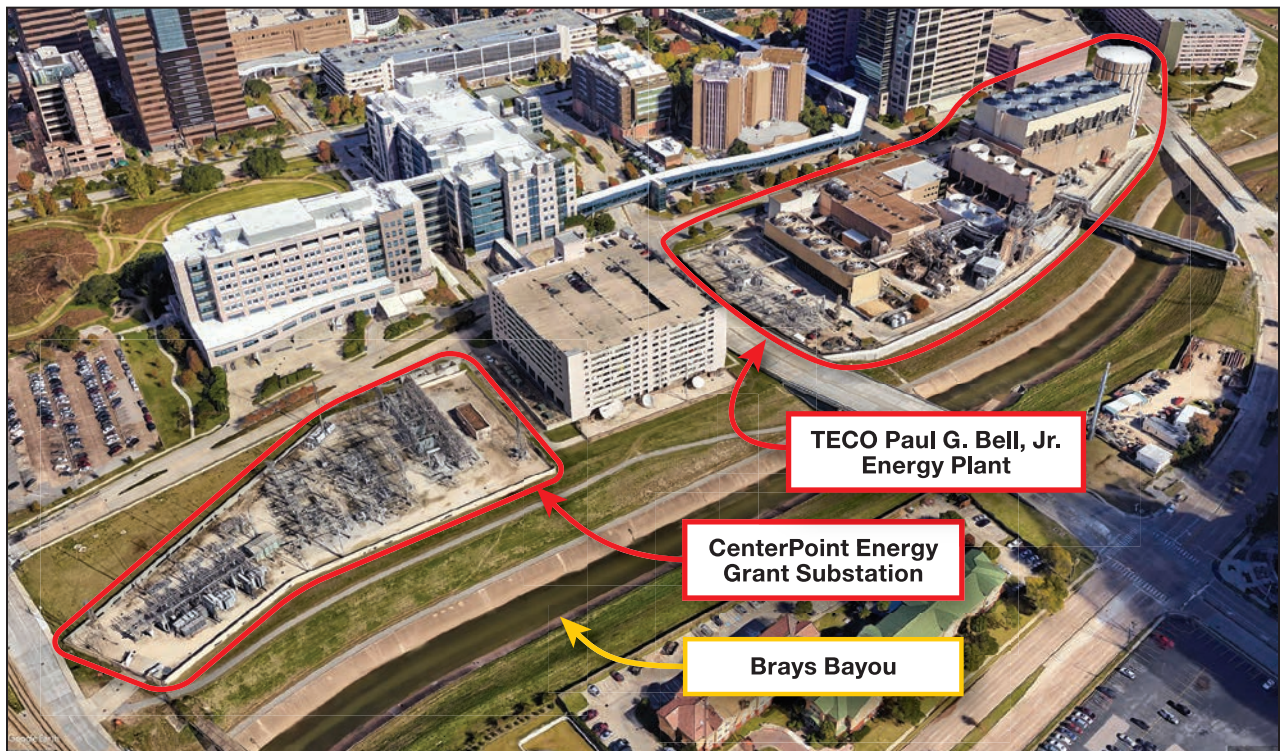
Figure 3-117: CenterPoint Energy Grant Substation and TECO Paul G. Bell, Jr. Energy Plant; aerial view looking northeast
