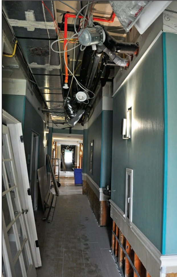
Figure 4-127: First floor corridor of a hotel (Rockport)
