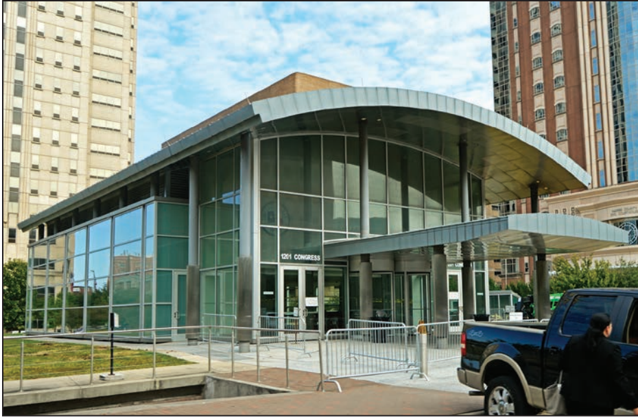
Figure 3-42: Jury Assembly Building viewed from the south
