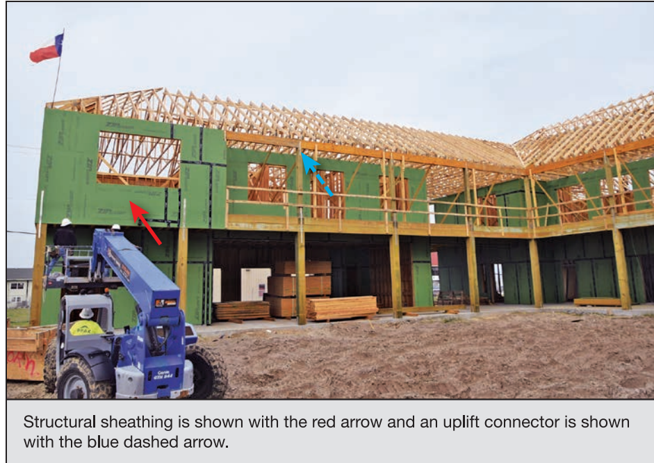
Figure 4-1: Apartment building under construction (Rockport)
