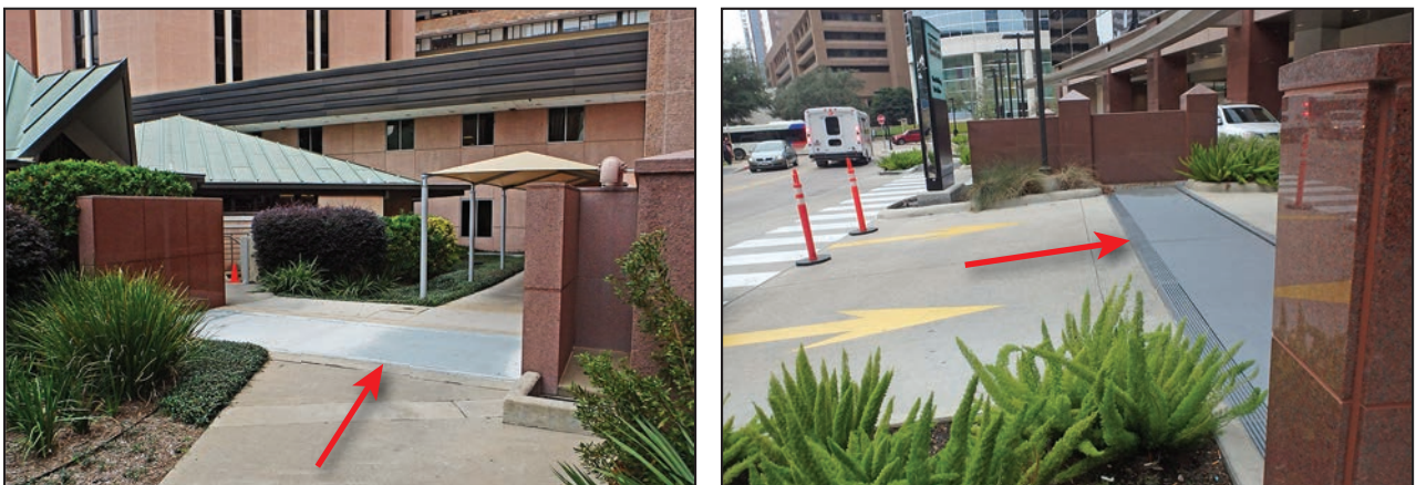
Figure 3-105: Passive floodgates (red arrows) at entrances through floodwall at the Main Building
