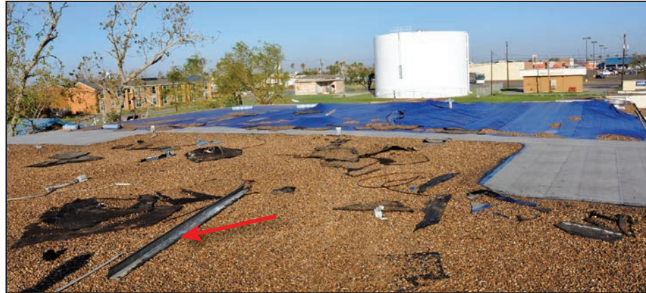
The red arrow indicates a section of metal edge flashing.
