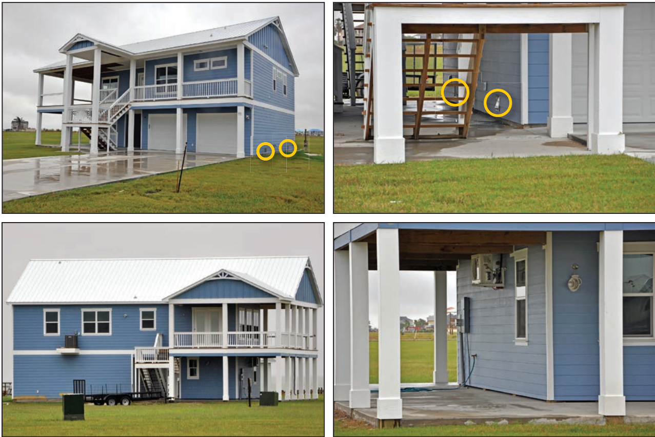
Residential building constructed with proper openings for the garage enclosure (top row, indicated by yellow circles), but no opening in the enclosure for access to the house (bottom row).
