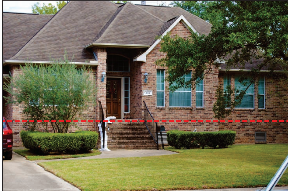
Figure 3-7: This elevated house built in 2002 (HWM, shown as the dotted red line) had much less damage than surrounding older slab-on-grade houses (example shown in Figure 3-8) [Zone AE]
