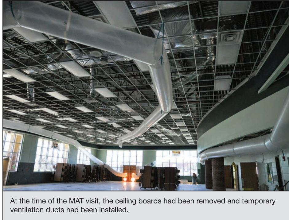
Figure 4-105: Interior view of the cafeteria
