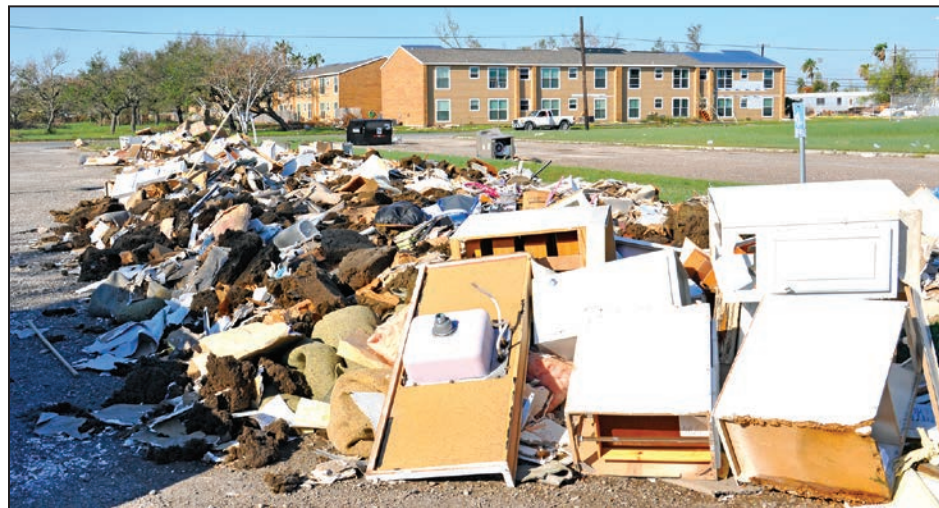
Figure 4-93: Cabinets and other debris from within the hospital
