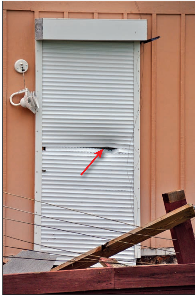
Figure 4-55: Classic roll-down shutter with missile impact (red arrow) (Copano Village)
