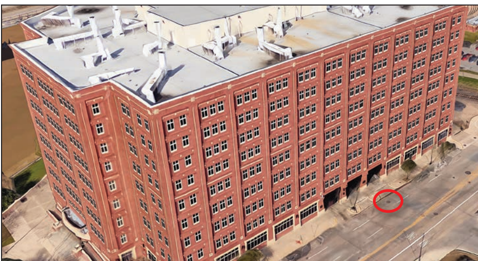
Figure 3-29: Location of below-grade communication vault (red circle) on N. San Jacinto Street
