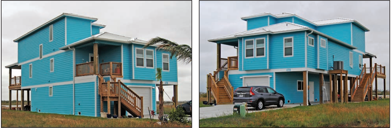
Figure 3-15: Elevated residence built in Nueces County in 2016 to Zone AE floodplain management requirements [Zone VE, per updated preliminary FIRM]
