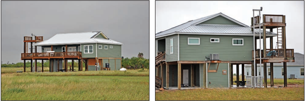
Figure 3-9: Elevated residence built in 2016 with flood damage (approximately $12,000) [Zone X]
