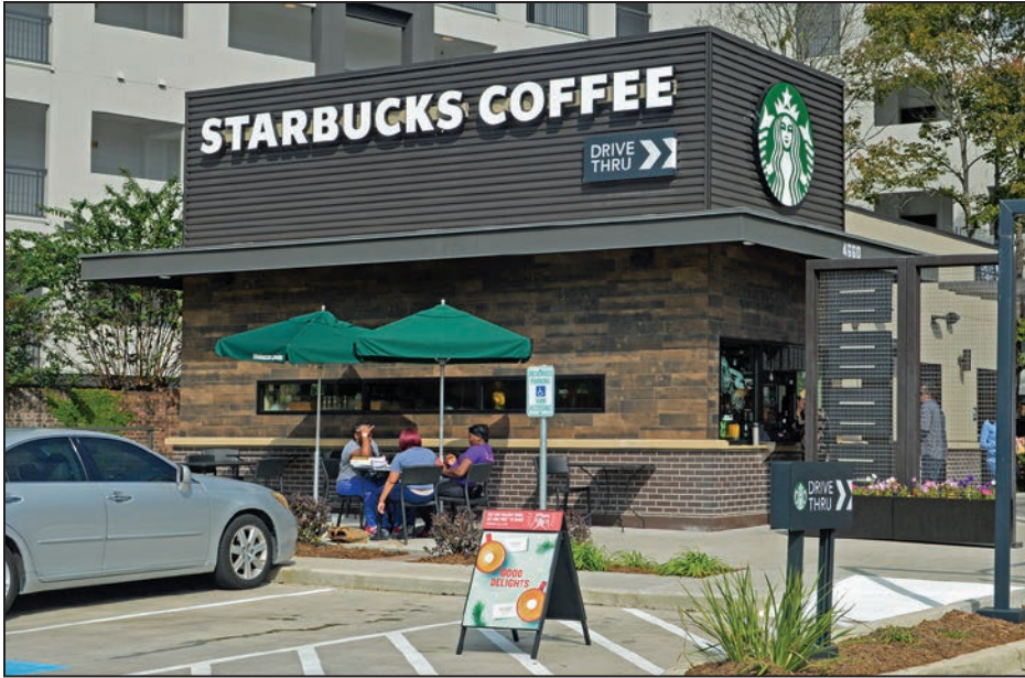
Figure 3-89: Shows the Starbucks building elevated on fill with dry floodproofing
