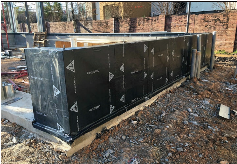
Figure 3-90: Membrane installed on the fully grouted and reinforced CMU wall
