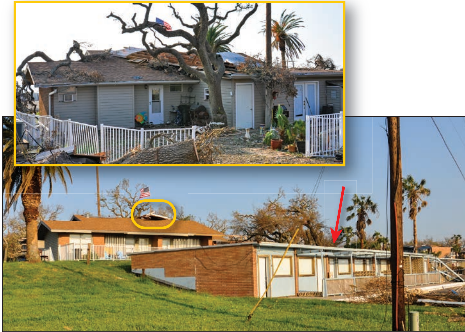
Figure 4-96: Building with aggregate surfaced BUR (Exposure D)
