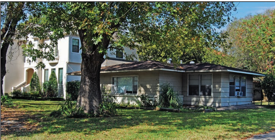
Figure 3-22: Example of an elevated residence (left side) next to a non-elevated residence (right side); the elevated house sustained much less damage during Hurricane Harvey
