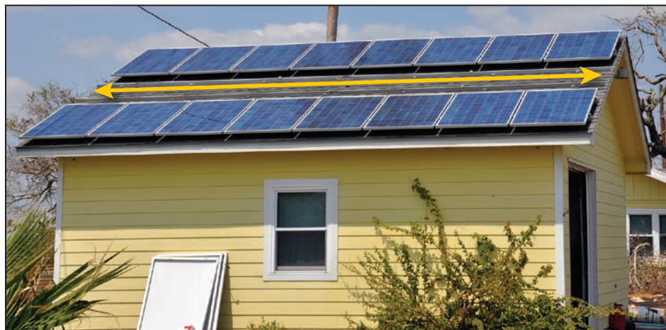
Figure 4-149: The yellow arrow indicates the row of missing solar panels
