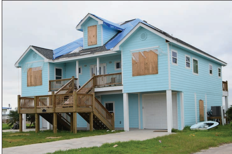
Figure 4-53: Typical plywood shutter installation on house (Rockport)
