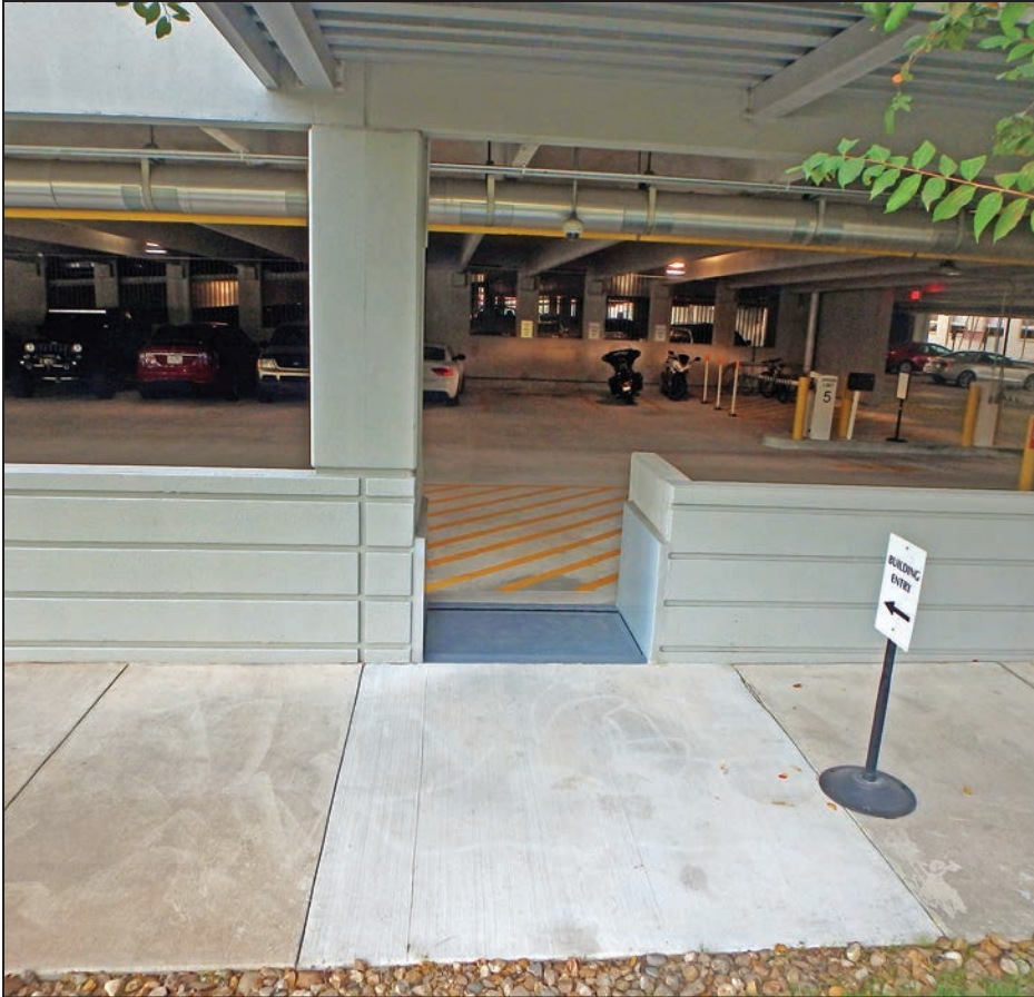
Figure 3-83: Parking garage for the Houston Galleria Office Tower
