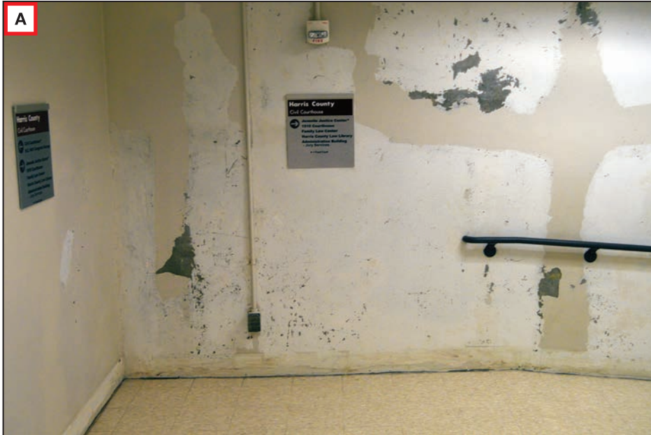
Figure 3-49: Civil Courthouse corridor
