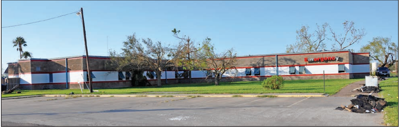
Figure 4-84: General view of the regional medical center (Aransas Pass)
