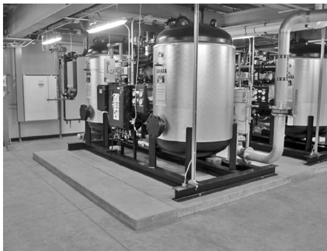
FIGURE C13.1-6 Skid-Mounted Components
