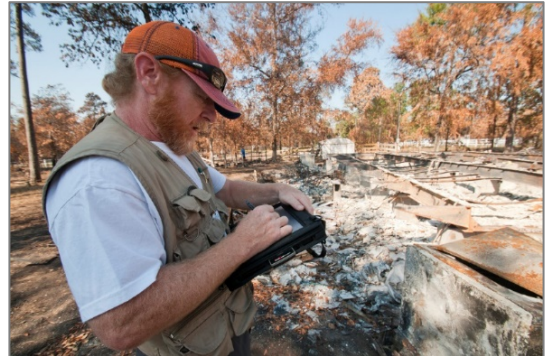
A FEMA inspector verifies wildfire damage at a severely impacted home site in Texas.
