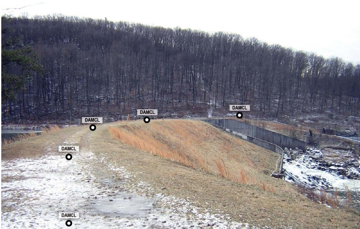
Figure 8: Typical Dam Photograph: Dam Centerline (Displays Survey Code Locations)
