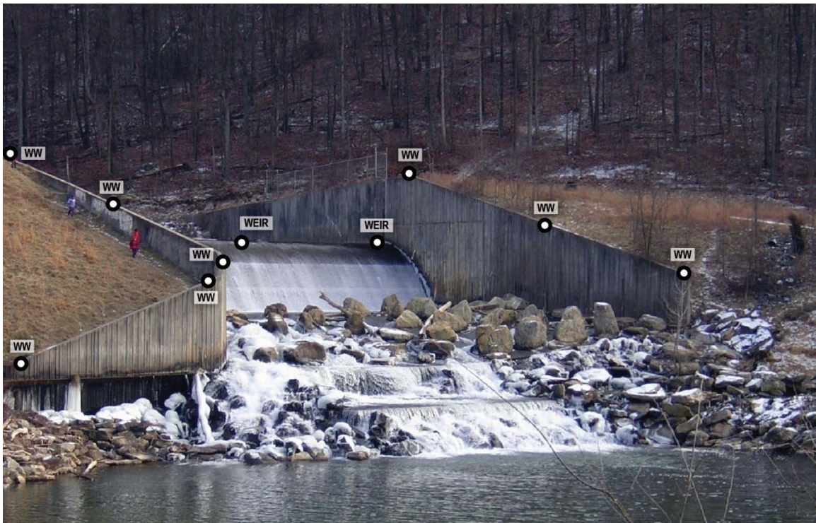
Figure 9: Typical Dam Photograph: Spillway (Displays Survey Code Locations)
