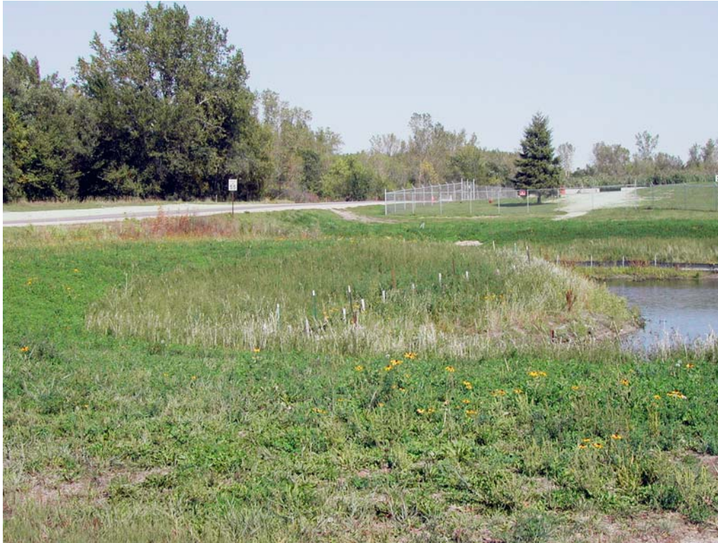
View of the north edge of existing stormwater pond and inlet. CR 17 visible in top left.
