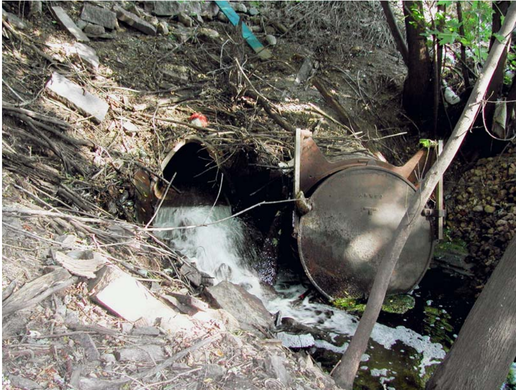
View of existing stormwater pond outlet and debris.
