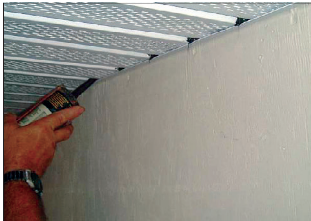
Figure 4. Applying dabs of sealant.
