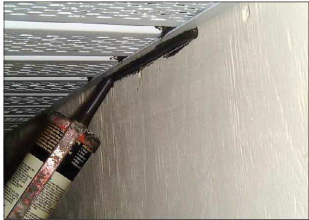
Figure 3. Applying a bead of sealant. (Note: Black sealant was used so that it would be visible in the photograph. Normally a matching sealant color would be used.)
