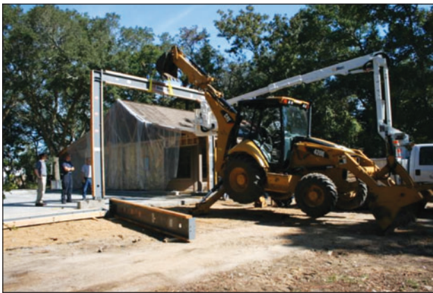
Figure 4. Installation of a prefabricated ordinary moment frame.
