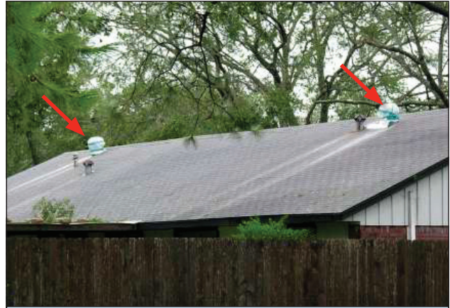
Figure 14. Plastic wrapped turbines.
