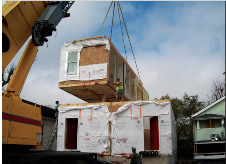
Figure 1. Construction of a modular home.
