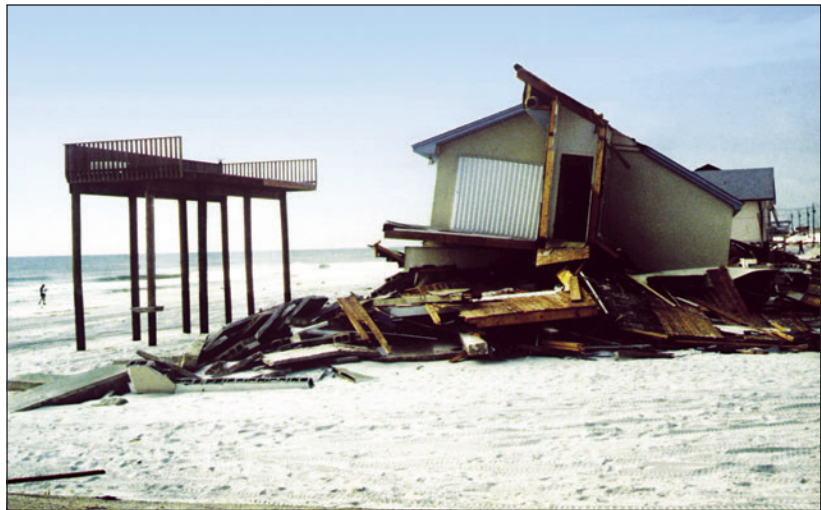
Damage from Hurricane Opal in Florida. This deck was designed to meet State of Florida Coastal Construction Control Line (CCCL) requirements. The house predated the CCCL and did not meet the requirements.
