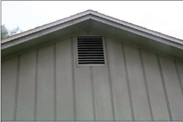
Figure 9. Gable end vent.
