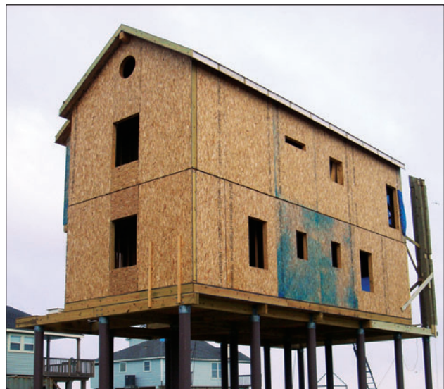
Figure 2. Construction of a Structural Insulated Panel house.
