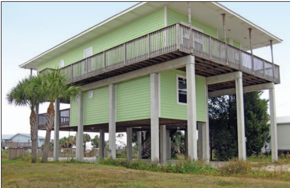
Figure 2-23. Above-grade enclosure (Perry, FL)
