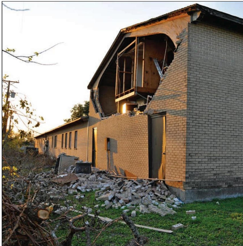
Figure B3-15: Example of falling debris hazard: Brick veneer failure on church (Refugio, Texas, 2017 hurricane)
