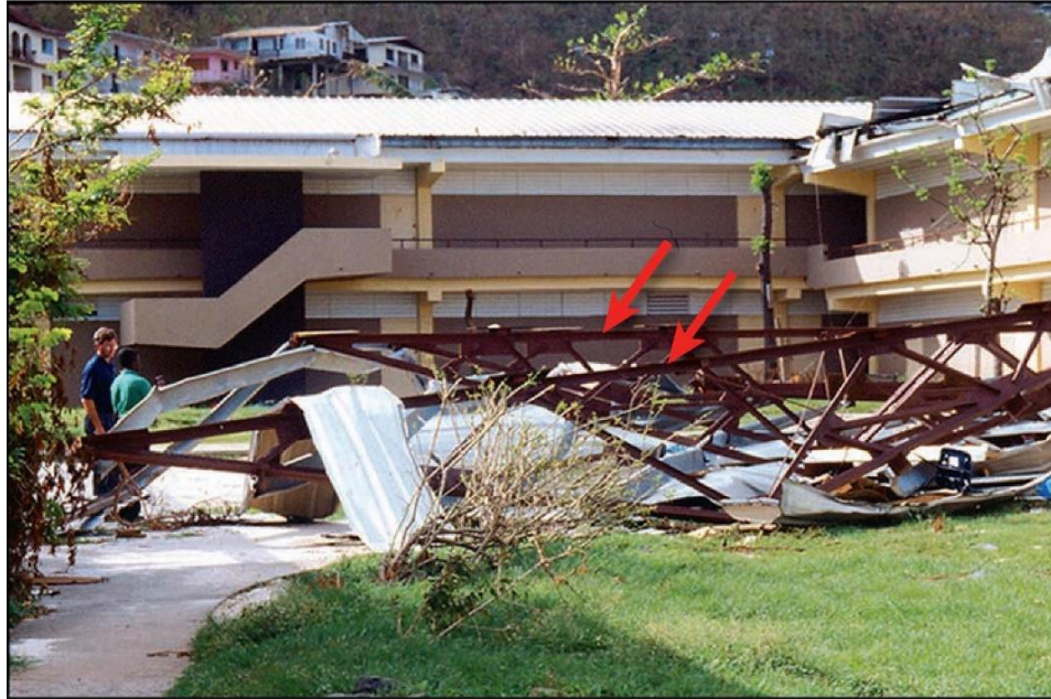
Figure B8-4: Large debris: Steel roof trusses that blew off a school (U.S. Virgin Islands, 1995 Hurricane Marilyn)
