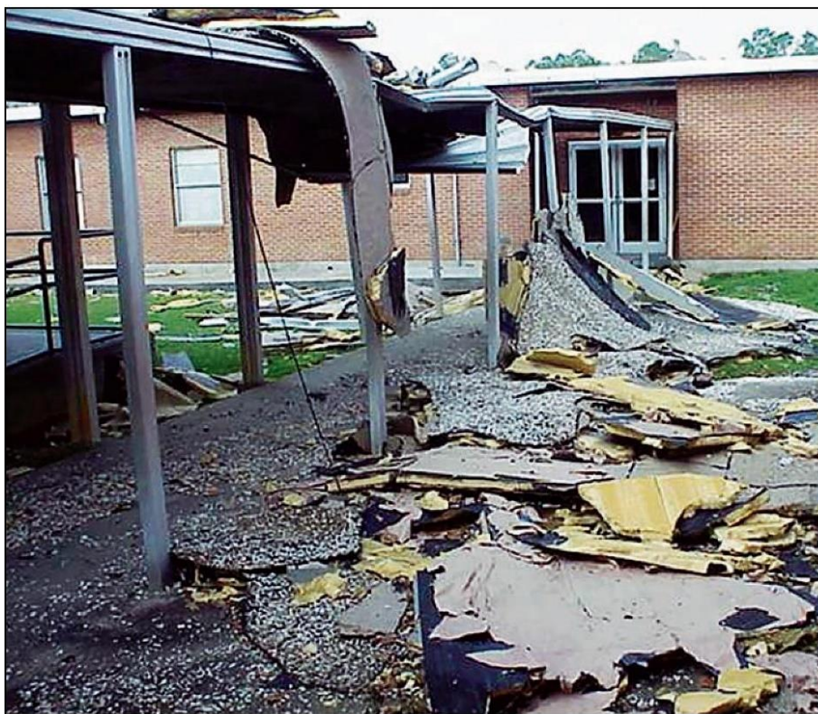
Figure B8-1: Medium debris: Pieces of a built-up roof from Hurricane Katrina (MS, 2005)
