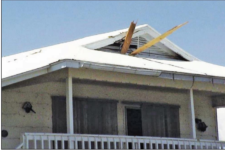
Figure B8-10: Impact of structural wood members in the gable end from a neighboring house (Pine Island, Florida)
