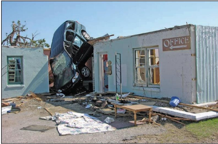
Figure B3-16: Vehicle rollover (Greensburg, Kansas, 2007 tornado)
