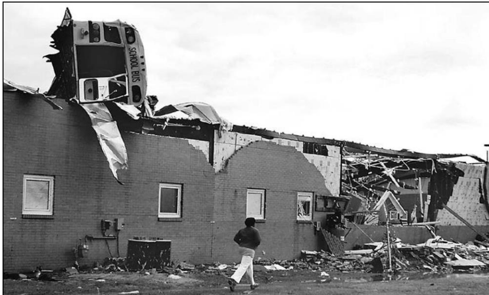
Figure B8-7: Large debris: A school bus was lifted atop a school (Caledonia, Mississippi, tornado, 2008)
