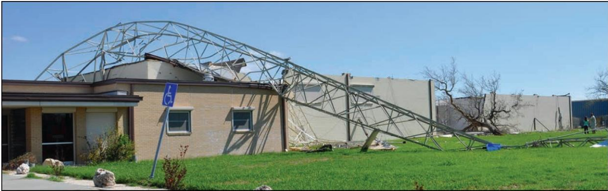
Figure B3-13: Laydown of communications tower onto a building (Rockport, Texas, 2017 hurricane)
