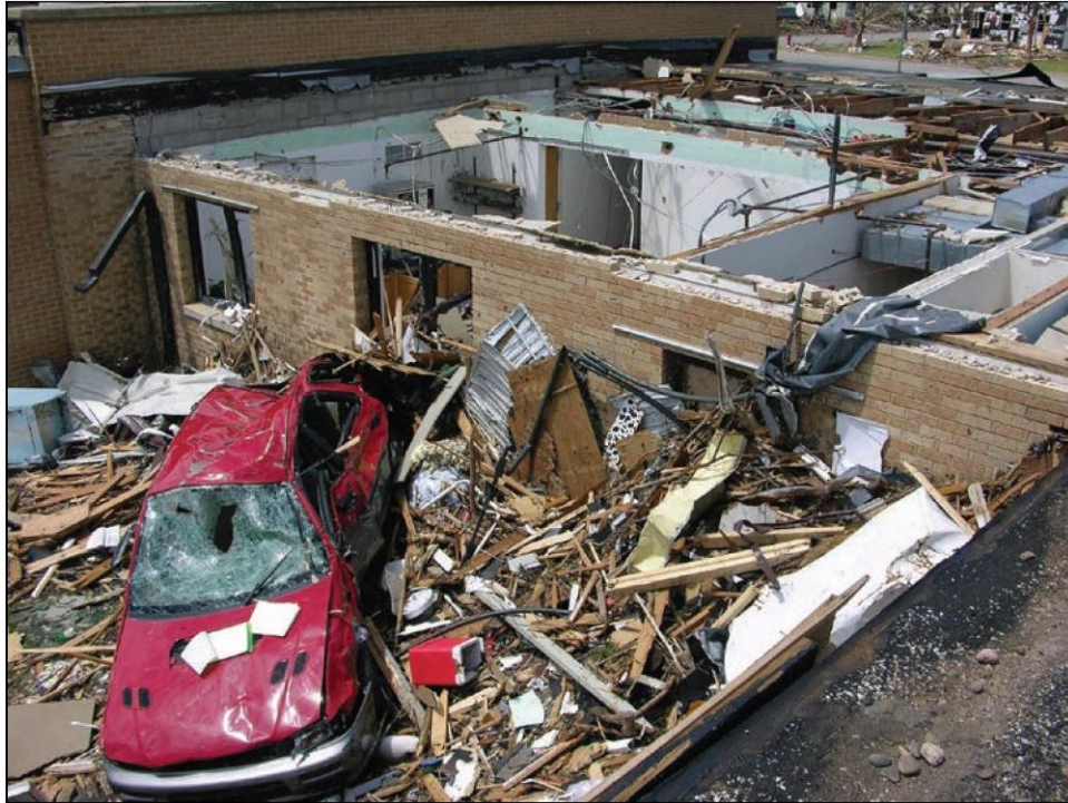
Figure B8-8: Representative quantity, size, and type of debris that is often generated by a strong or violent tornado. The building damage at this site was indicative of an EF3 tornado. (Greensburg, Kansas, 2007)
