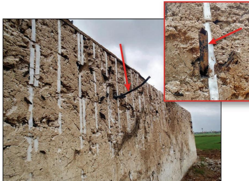
Figure B8-17: Red arrows show a steel tube that perforated a waffle grid ICF wall. Inset shows the tube in the “as found” condition and main photograph shows the tube after it was partially pulled out of the wall. (Moore, Oklahoma, 2013 tornado)
