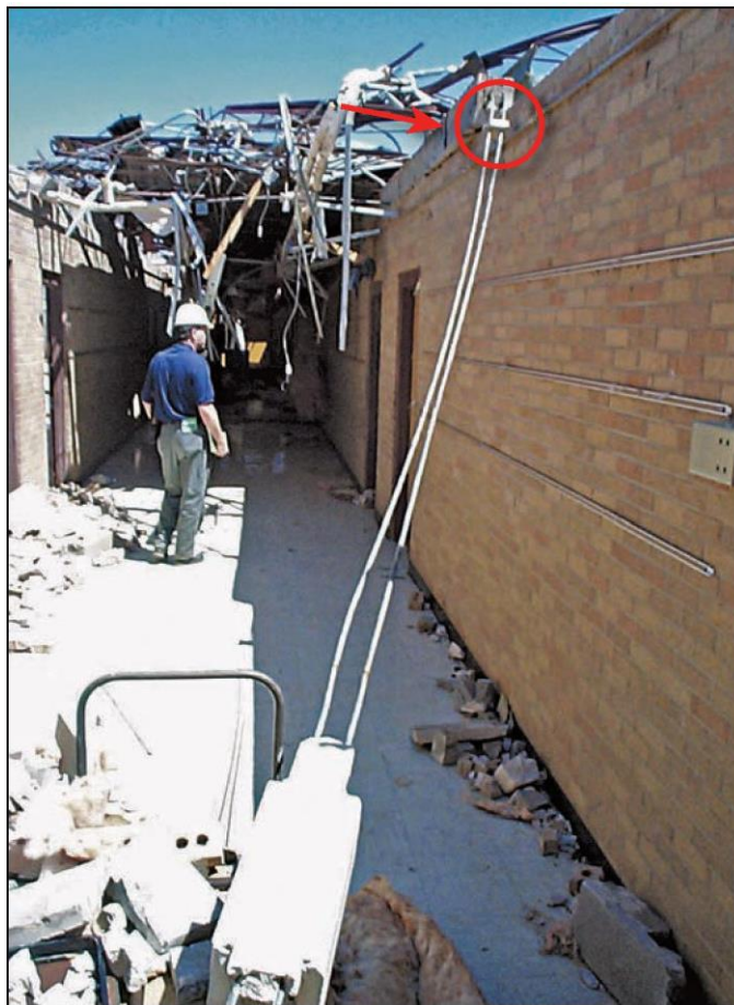
Figure B3-8: Failure of load path between the bond beam and the top of the unreinforced masonry wall when struck by an F4 tornado (Moore, Oklahoma 1999 tornado)
