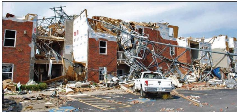
Figure B3-14: Laydown of a large communications tower onto a building (Joplin, Missouri, 2011 tornado)
