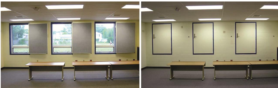
Figure A4-5: Interior operated safe room shutters in a multi-purpose classroom/safe room. Image on left is normal usage; image on right shows shutters in "lock down" position where they are closed and latched
