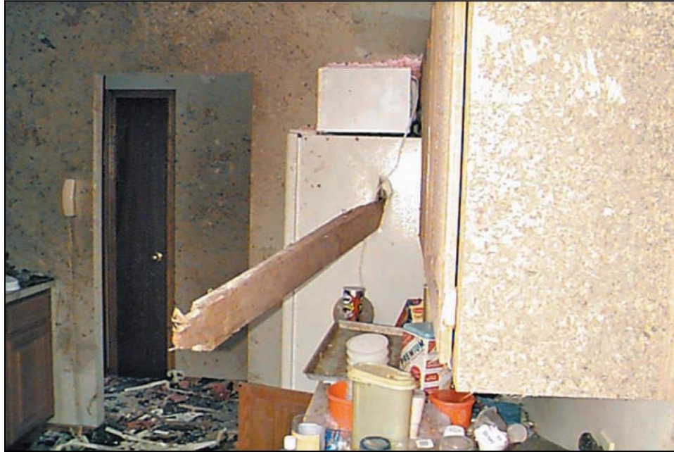
Figure B8-9: Refrigerator pierced by a 2x6. The portion of the 2x6 that is visible was 4 feet 8 inches long. It went several inches into the freezer compartment. (Oklahoma City, Oklahoma, 1999 tornado)
