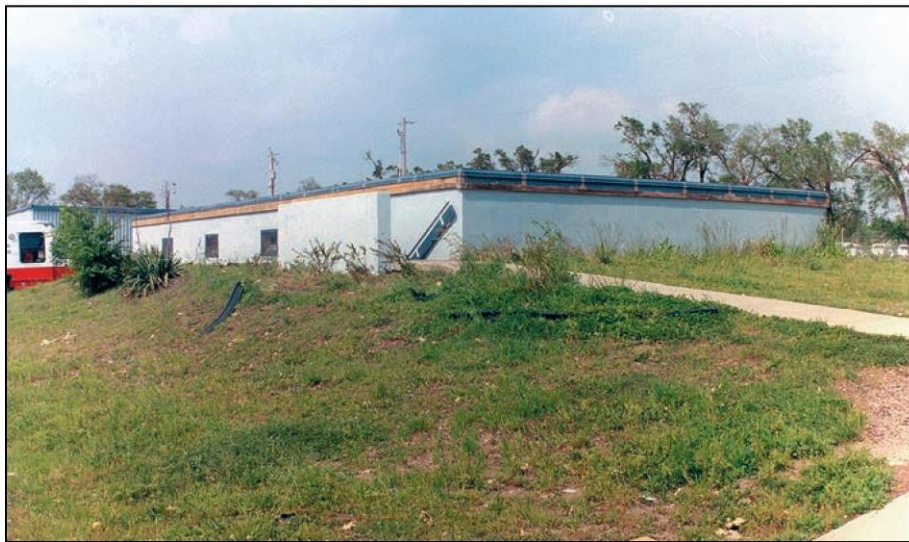
Figure B3-10: View of a community shelter that is partially below grade (Wichita, Kansas, 1999 tornado)
