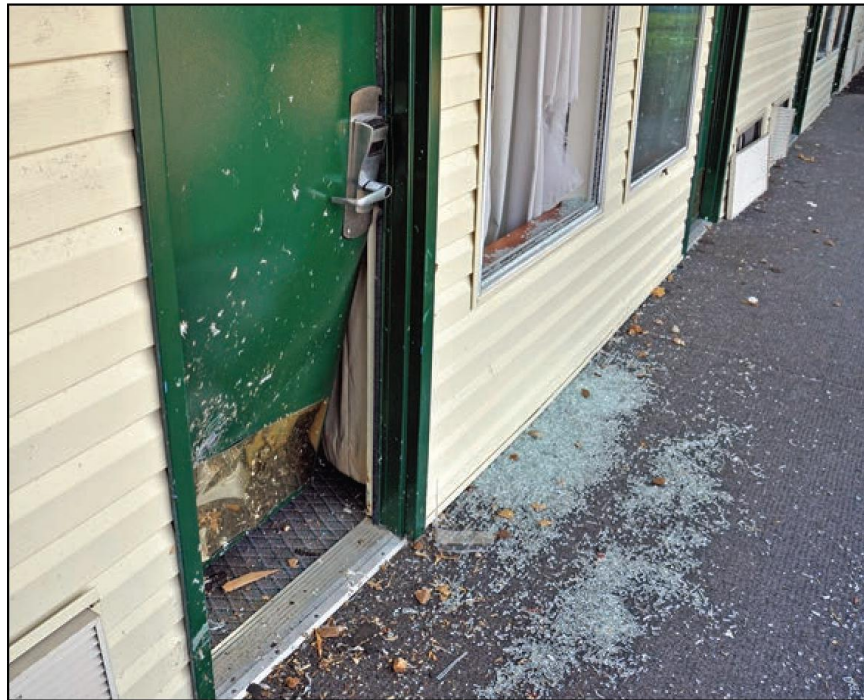
Figure B8-18: This metal door was damaged by wind-borne debris generated by a weak tornado. The bottom hinge was damaged, but the single latch was able to resist the modest wind and impact load. The door was on the verge of failing. (St. Louis, Missouri, 2013 tornado)
