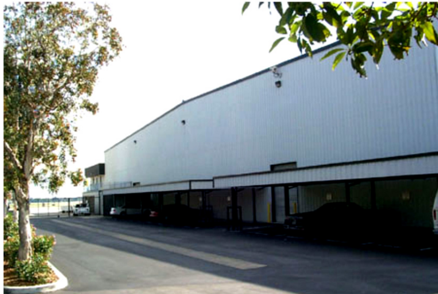
Figure E-18 Prefabricated metal building (S3, light metal building).
