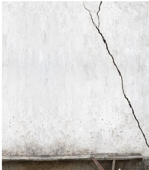
Figure F-7 Concrete cracks.
