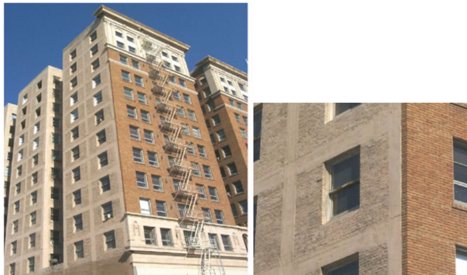
Figure E-33 C3 building and detail showing concrete frame with URM infill (left wall), and face brick (right wall).
