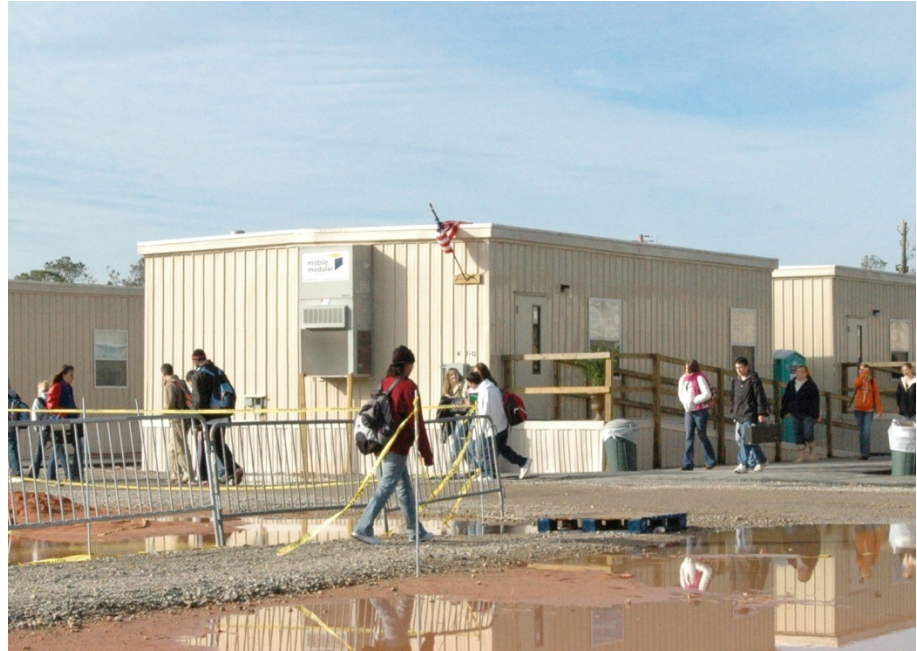
Figure 7-21 Exterior view portable classrooms at New City High School (from www.fema.gov ).
