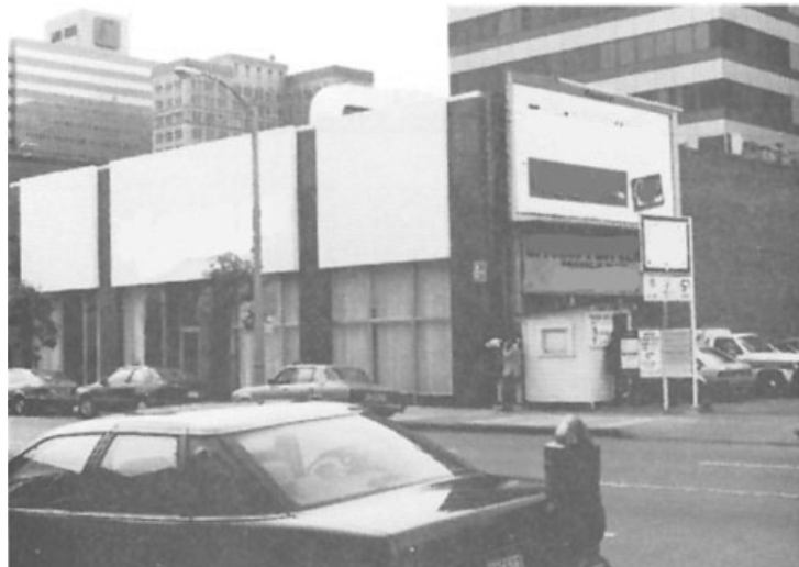
Figure D-8 A 1970s renovated façade hides a URM bearing wall structure.
