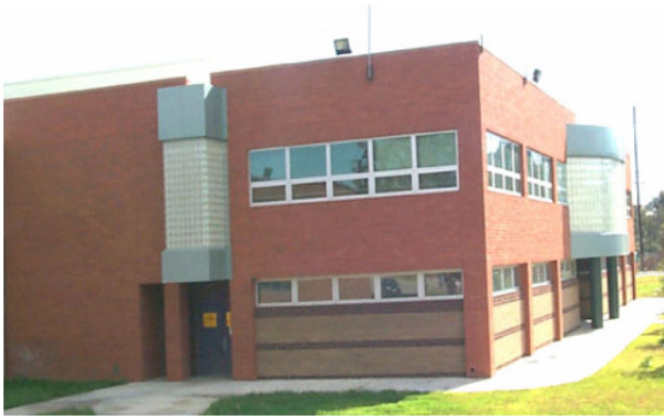
Figure 7-15 Exterior view of modern reinforced brick masonry building at Roosevelt Elementary School.
