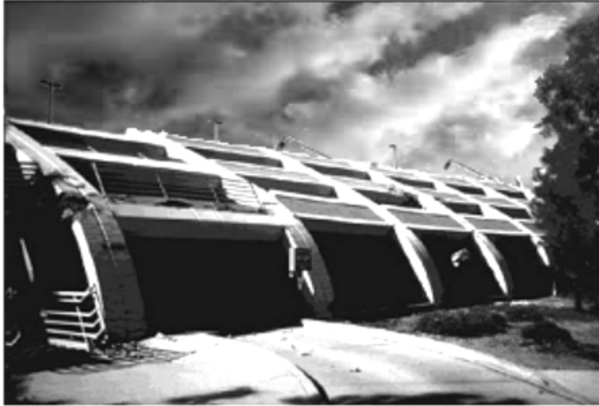
Figure E-25 Extreme example of ductility in concrete, 1994 Northridge earthquake.
