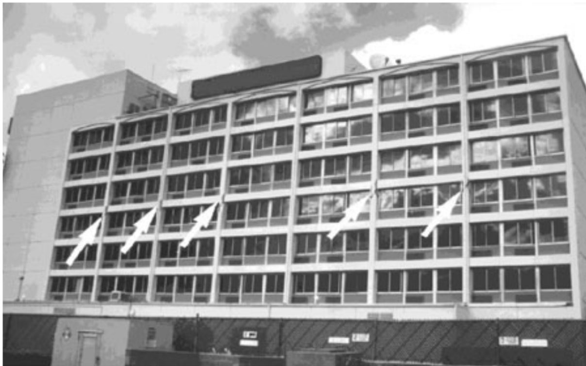
Figure E-28 Locations of failures at beam-to-column joints in nonductile frames, 1994 Northridge earthquake.
