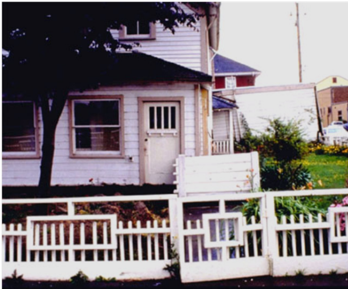
Figure G-7 Photo of house settled to the ground due to collapse of its post and pier foundation.
