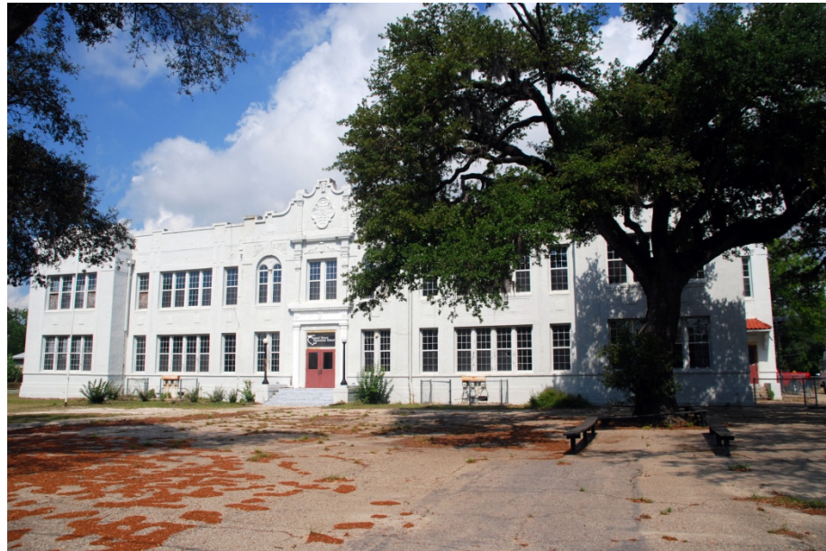
Figure 7-18 Photo of exterior of Washington Middle School (from www.fema.gov ).
