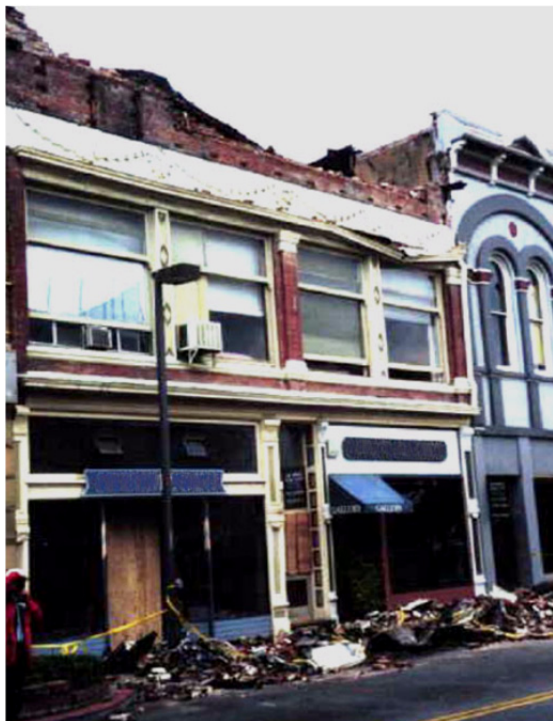
Figure E-52 Parapet failure leaving an uneven roof line, due to inadequate anchorage, 1989 Loma Prieta earthquake.
