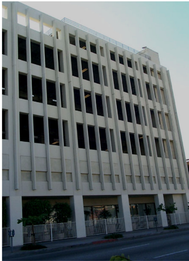
Figure E-27 Concrete moment-resisting frame building (C1) with exposed concrete, deep beams, wide columns (and with architectural window framing).
