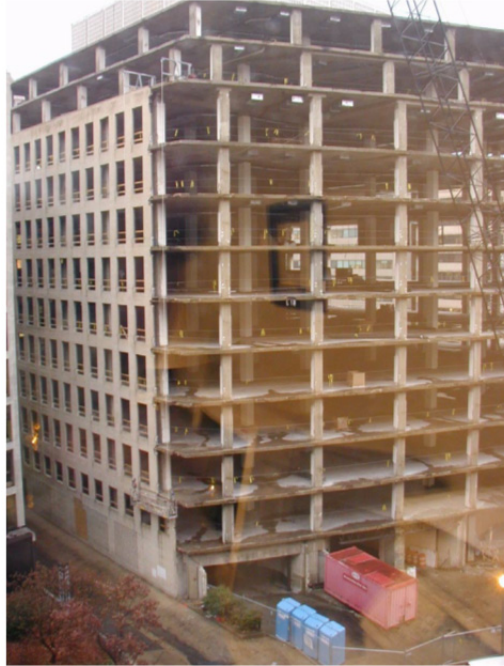
b. Reinforced concrete frame under renovation: demolition of older façade units.
