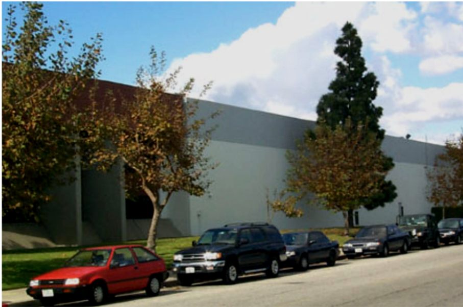
Figure E-35 Tilt-up industrial building, 1970s.
