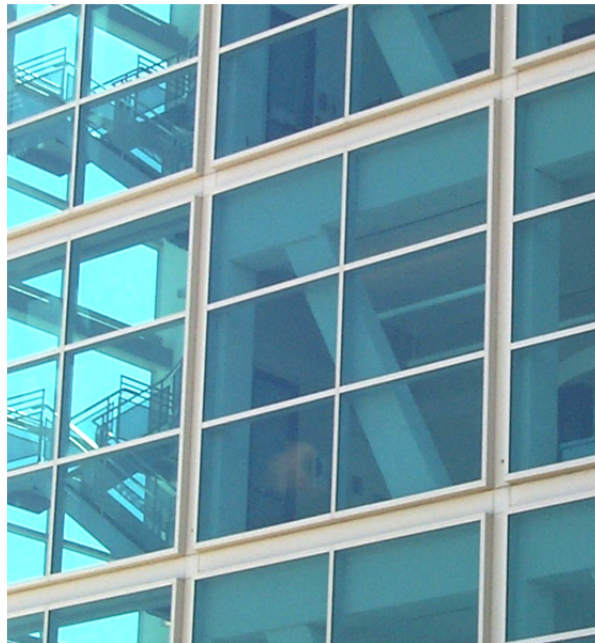
Figure 7-6 Close-up view of 3703 Roxbury Street exterior showing perimeter braced steel framing.
