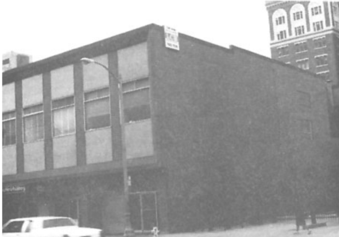
Figure D-9 A concrete shear wall structure with a 1960s renovated façade.
