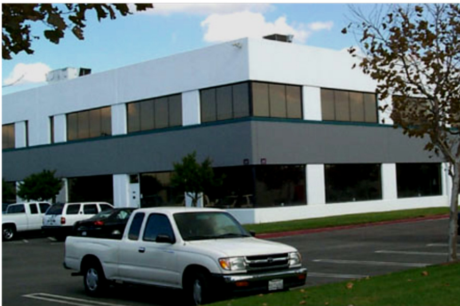
Figure E-36 Tilt-up industrial building, mid- to late-1980s.
