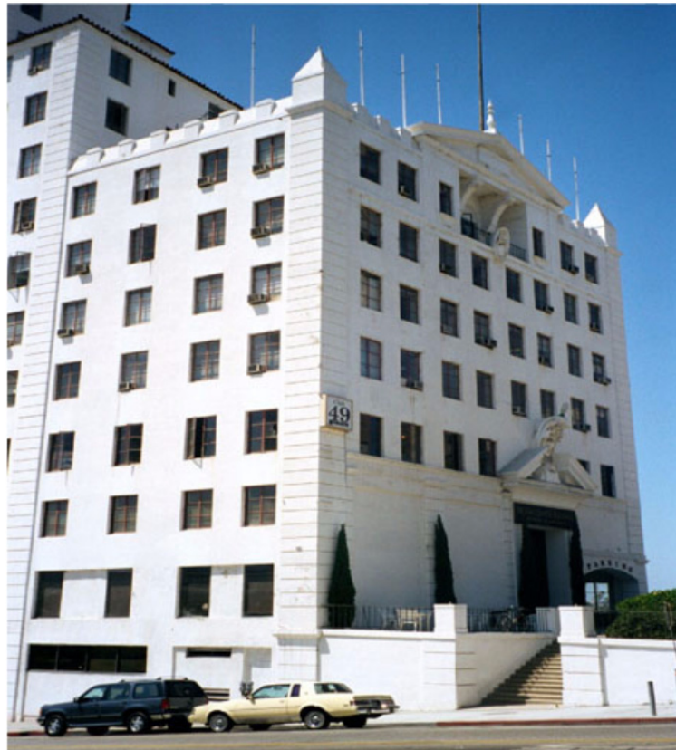
Figure E-20 Concrete shear wall on building exterior.
