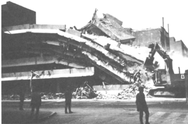
Figure G-3 Mid-rise building collapse, 1985 Mexico City earthquake.
