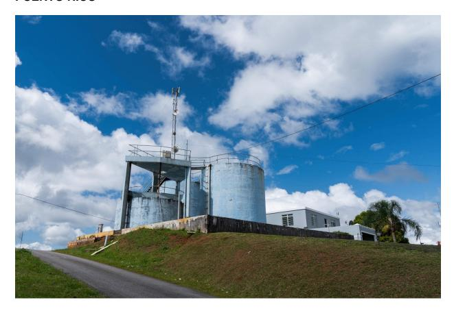
**Naranjito, Puerto Rico** (January 23, 2023). FEMA allocated over \$101,400 to repair three wells at the aqueduct system in the Anones neighborhood in Naranjito. Repairs included the chlorination replacement, which contributes to the operation and provision of drinking water for approximately 500 families in the area. Mitigation funds were assigned for a surge protector and to strengthen the fence. Photo FEMA/Eliezer Hernández
