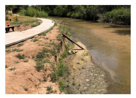
Figure 7: 2019 Mill Race North Bank Damage Conditions
