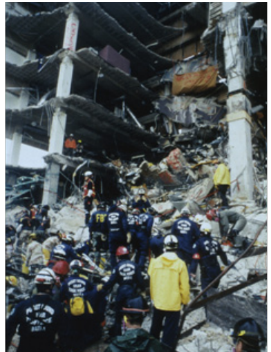
Urban Search and Rescue teams sift through the debris from the bombing of the Alfred P. Murrah Federal Building.
