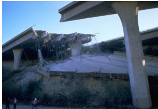
Entire highways collapsed during the Northridge Earthquake in 1994.
