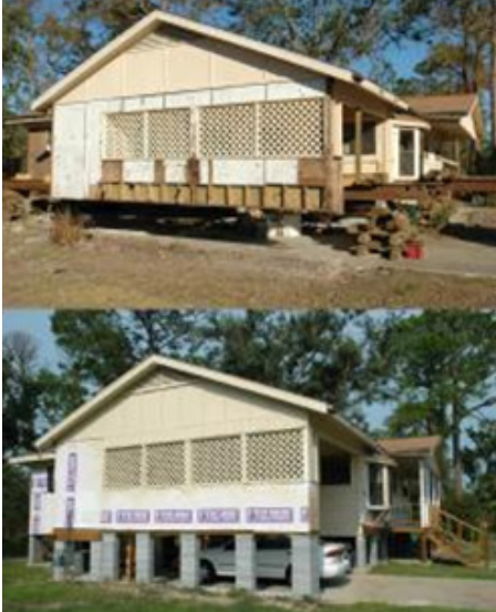
Home elevations are an important aspect of flood mitigation efforts.
