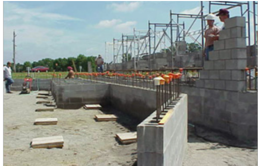
Better building practices help the long term protection of communities.
