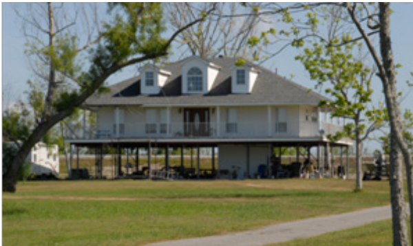
This elevated home in Port Sulphur, Louisiana is an example of the results created by mitigation.
