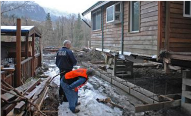
This home in Gold Bar, Washington was relocated 60 feet back from the Snohomish River to prevent future flooding.
