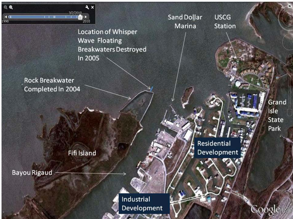
Figure 2 – Existing Conditions at Proposed Project Area
