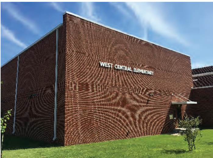
West Central Elementary School's safe room, the exterior of which is pictured here, is one of 14 safe rooms in the Joplin, Missouri school district funded in large part through the HMGP.
