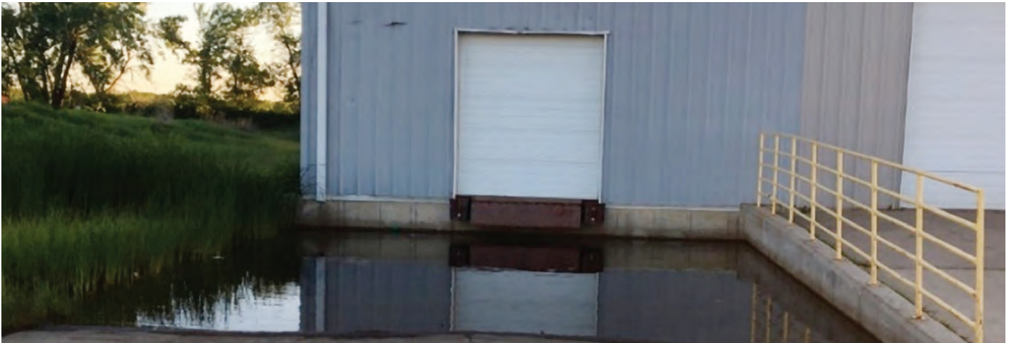
Before installation of the winged culvert.
