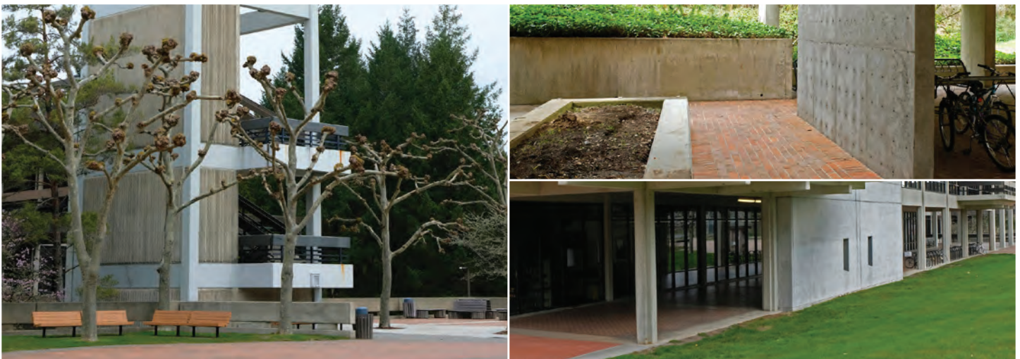
Scenes from The Evergreen State College show seismic retrofit projects that have increased the campus’ resiliency to future seismic events.
