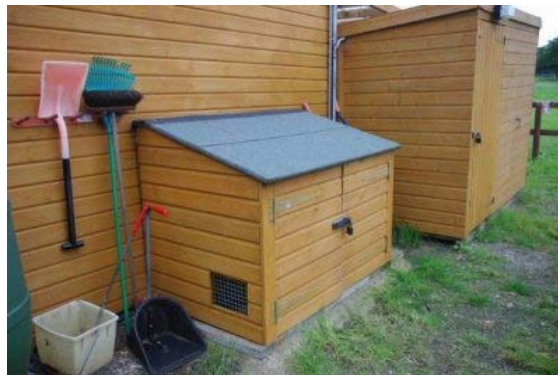
Figure 45. Attached Utility Shed
