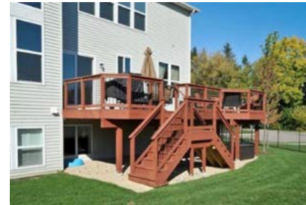
Figure 18. Deck with Double Staircase
