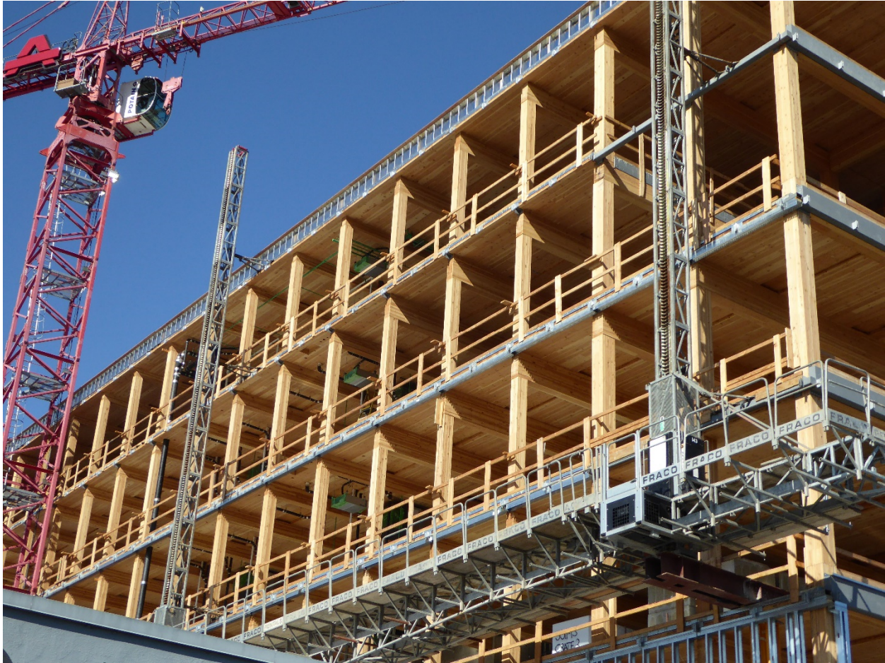
Figure 6-4. Cross-Laminated Timber Building Under Construction (Photo Credit, Sandra Hyde)
