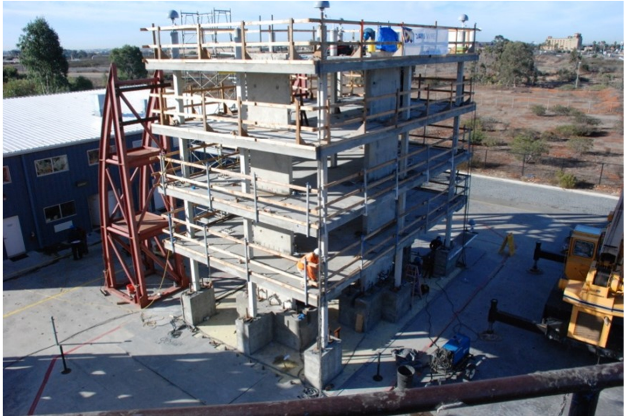
Figure 4-1. Shake Table Testing of a Four-Story Reinforced Concrete Building (Jacobs School of Engineering/University of California San Diego from https://www.flickr.com/photos/jsoe/21512310022/in/album-72157637612765485/ )
